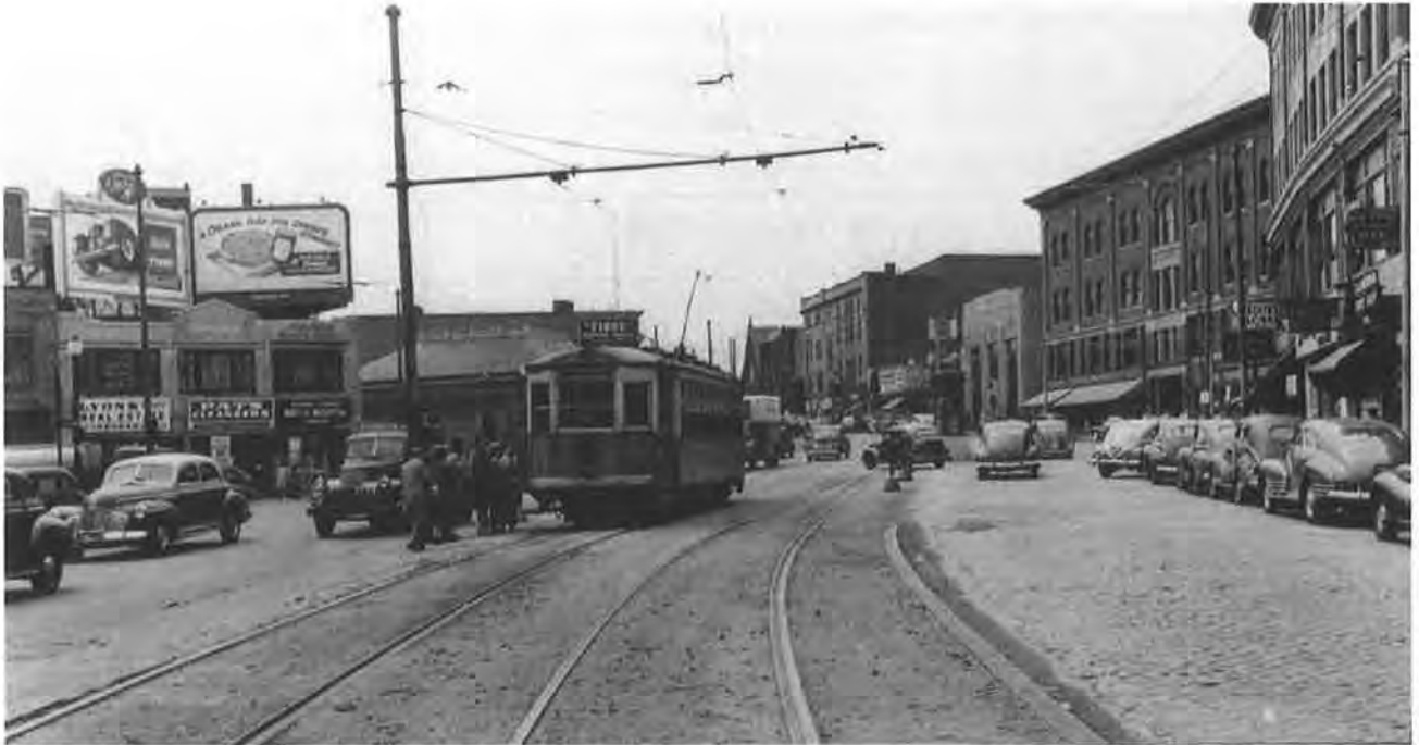
Figure 4: Typical view of a streetcar picking up passengers on Columbia Road in Dorchester near Upham's Corner, ca. late 1940s. The doublewide overhead bracket arms were a distinctive feature on Columbia Road. [Bradley H. Clarke, Streetcar Lines of the Hub: The 1940s Heyday of Electric Transit in Boston Boston: Boston Street Railway Association, 2003, 46.] (Courtesy of Bradley H. Clarke).
