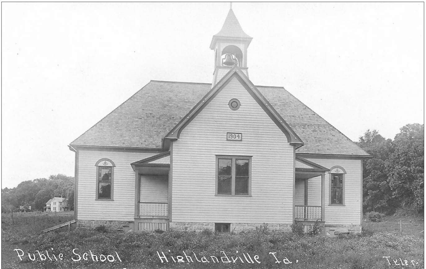
Figure 7. Undated historic photograph of the 1904 Highlandville School (on file Winneshiek County Historic Preservation Commission).
