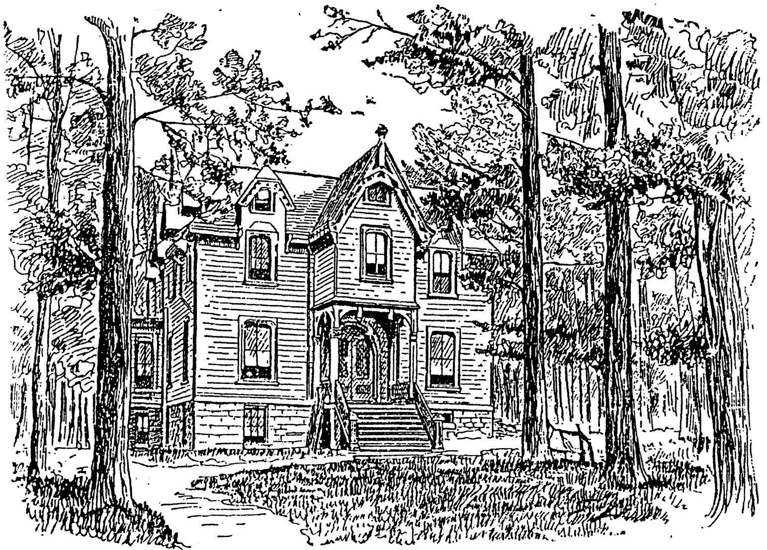
DERROM HOUSE—EAST SIDE PARK.
