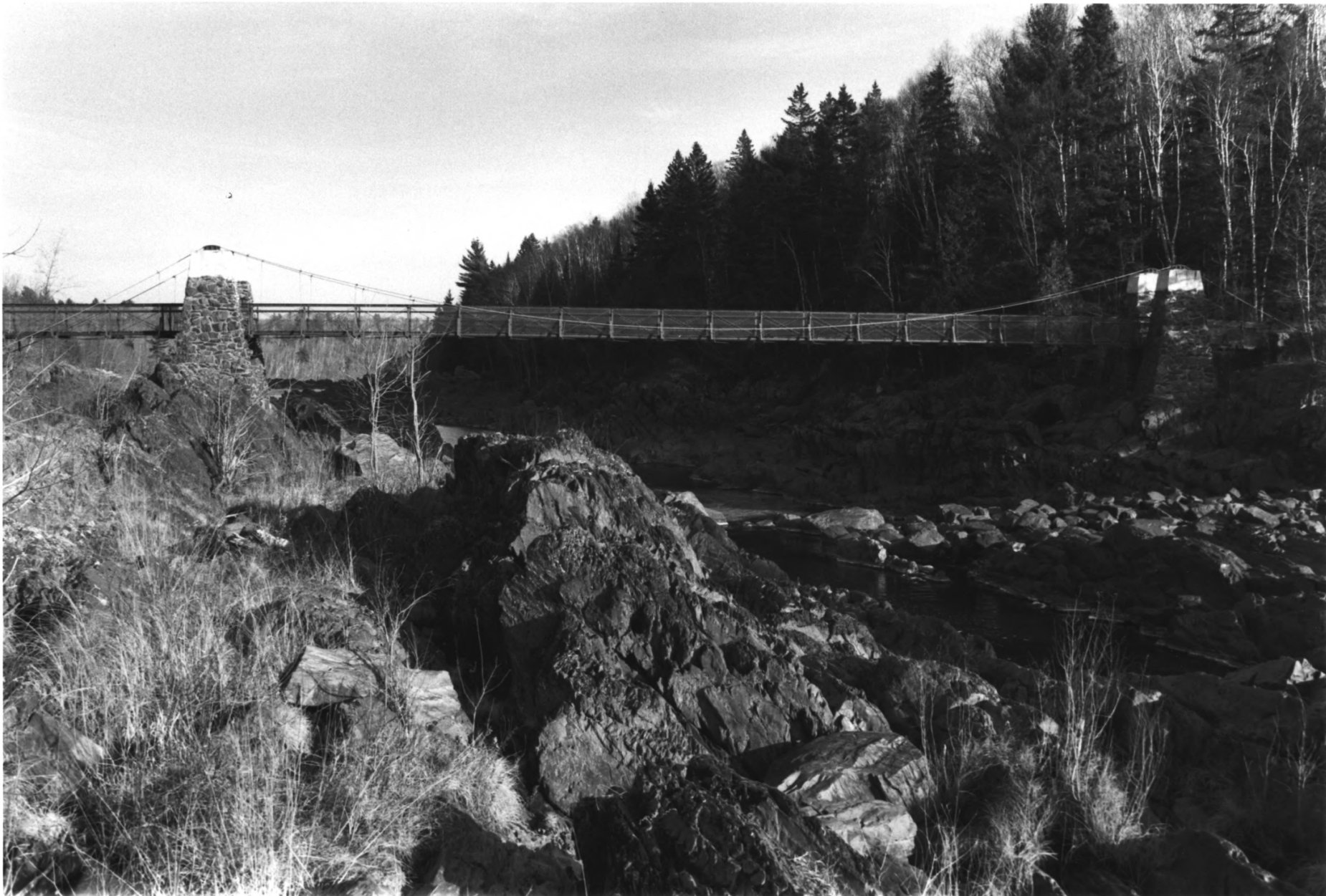
JAY COOKE STATE PARK CARLTON CO., MN STRUCTURE # 2 PHOTO I.D. 09124 #5
