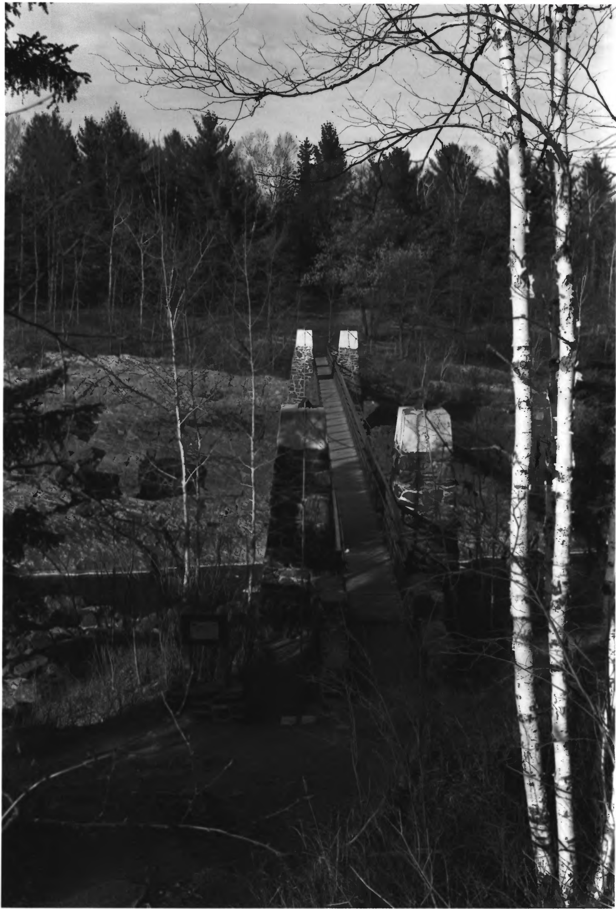
JAY COOKE STATE PARK CARLTON CO., MN STRUCTURE # 2 PHOTO I.D. 09124 # 4
