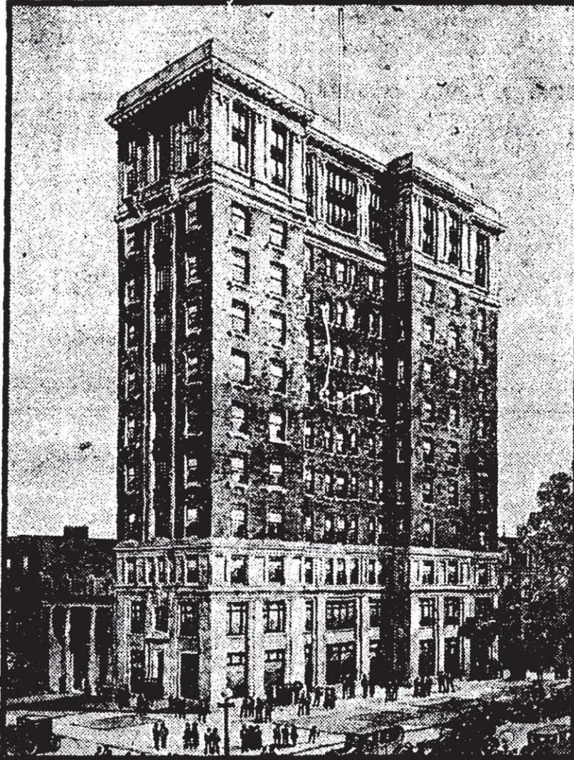
Phillips building, southeast corner of Fifteenth and K streets north-west. William S. Phillips recently purchased this property (formerly known as the Davidson building) from Davidson and Davidson, and has located his real estate offices here, occupying the entire first floor. The new offices will be formally opened tomorrow.
