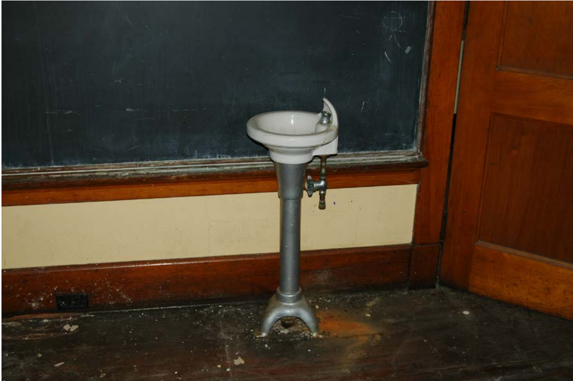
Photo #13 Classroom 2, close up view of water fountain
