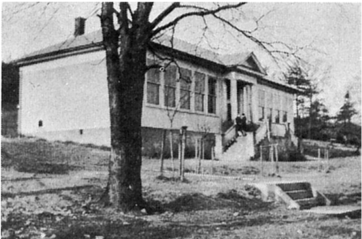
Figure 8: Lackawaxen Consolidated School, c.1924, rear façade.
