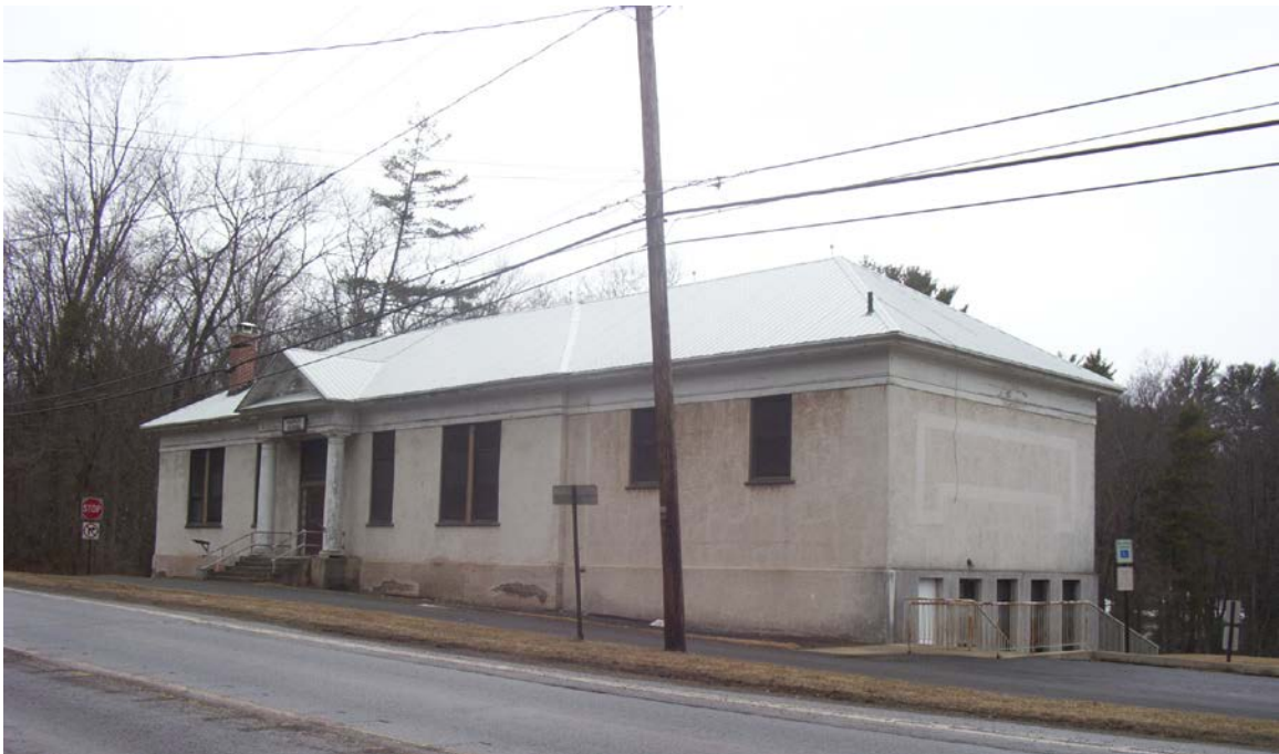
Photo #2 Southeast façade (left), northeast façade (right), camera facing west
