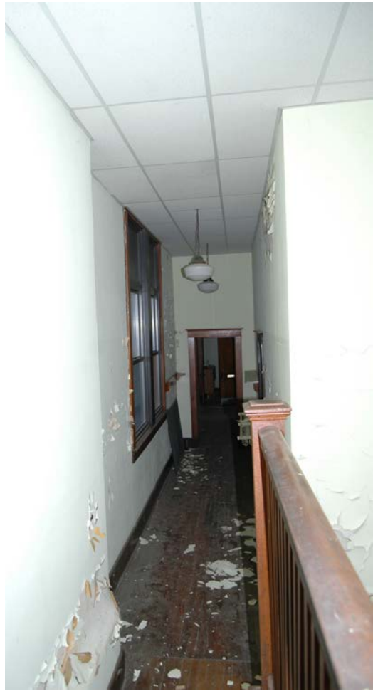
Photo #20 Front hallway, facing southwest
