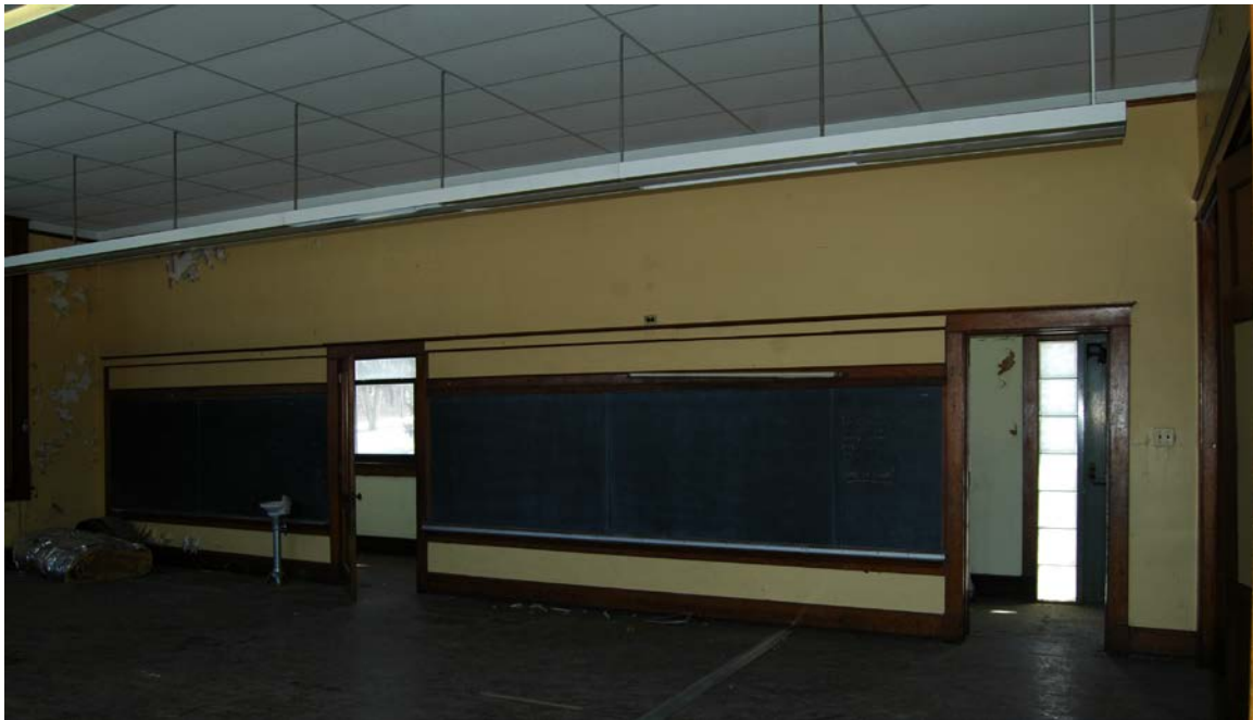
Photo #10 Classroom 2, southeast wall (oblique)
