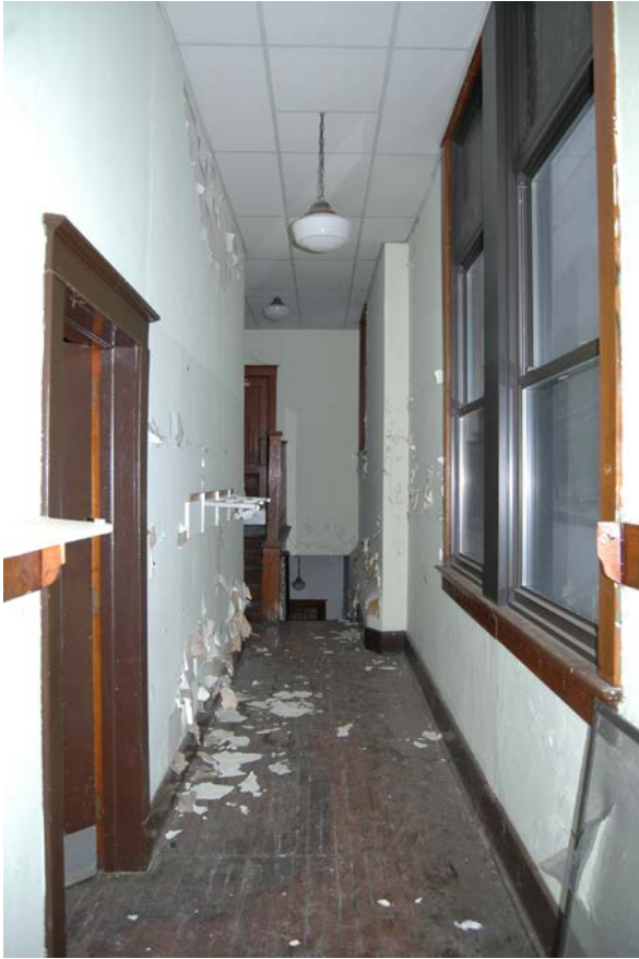
Photo #21 Front hallway, facing southwest
