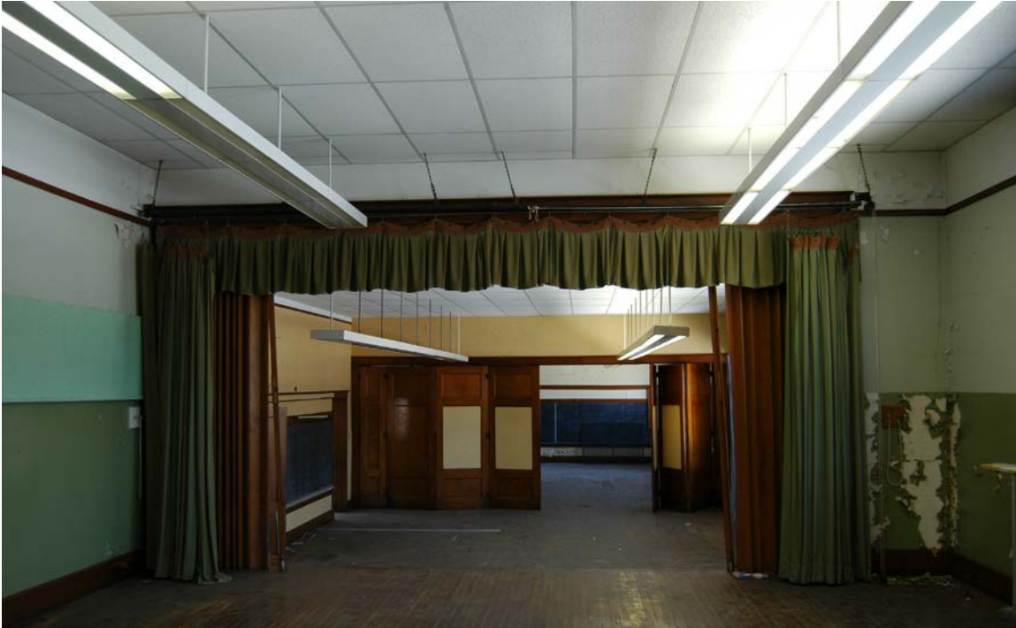
Photo #17 Stage, northeast wall (curtain wall)
