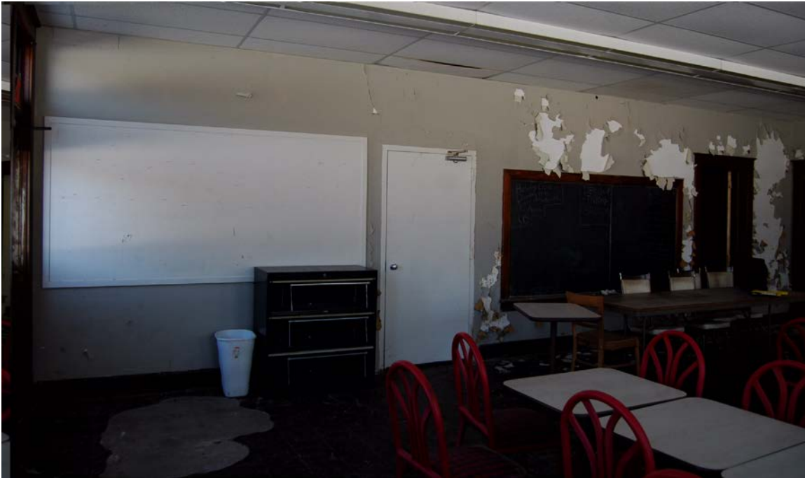
Photo #29 Music and Art room, southeast wall (oblique)
