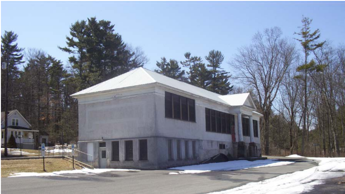
Photo #4 Northeast façade (left), northeast façade (right), camera facing south
