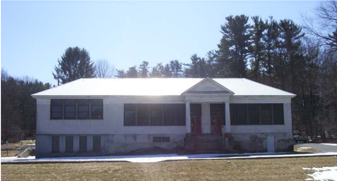
Photo #3 Northwest façade, camera facing southeast
