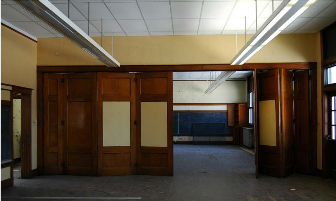
Photo #11 Classroom 2, northeast wall (accordion divider)
