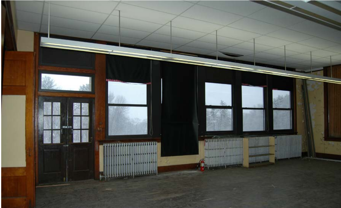
Photo #9 Classroom 2, northwest wall (oblique)
