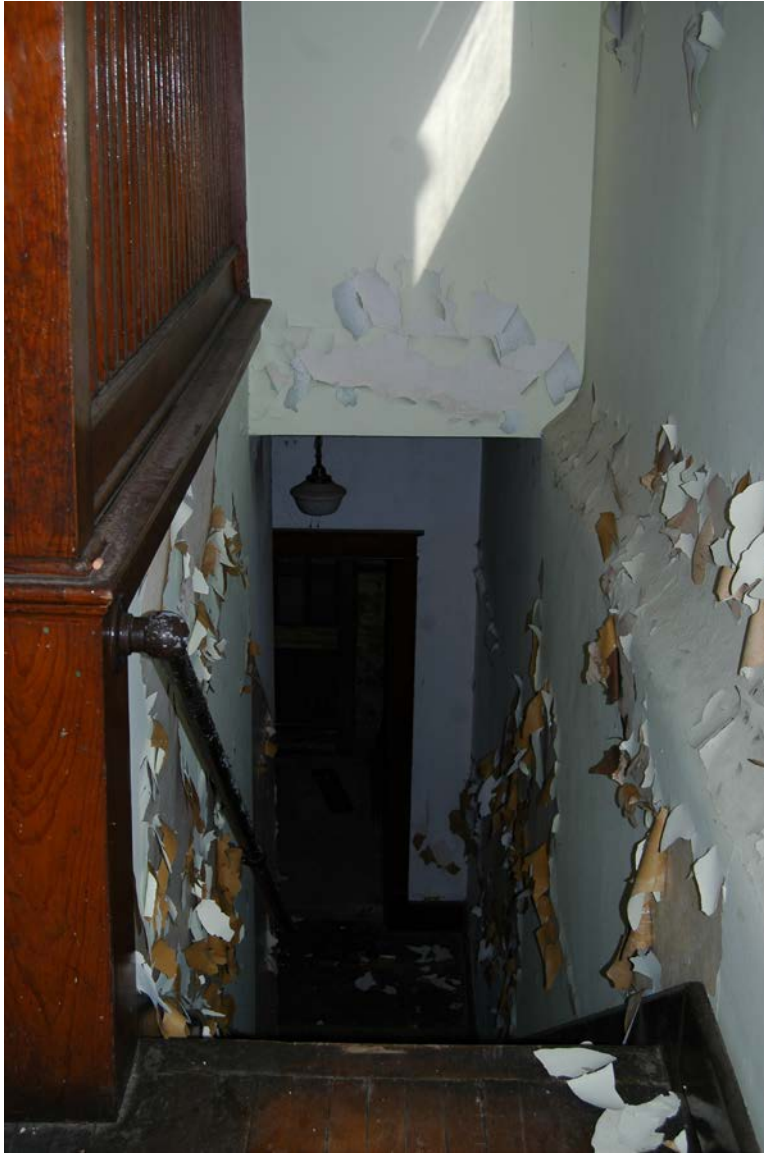
Photo #25 Stairs to basement
