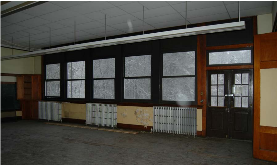
Photo #8 Classroom 1, northwest wall (oblique)
