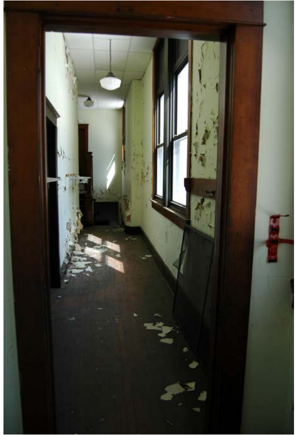
Photo #22 Front hallway, facing northeast
