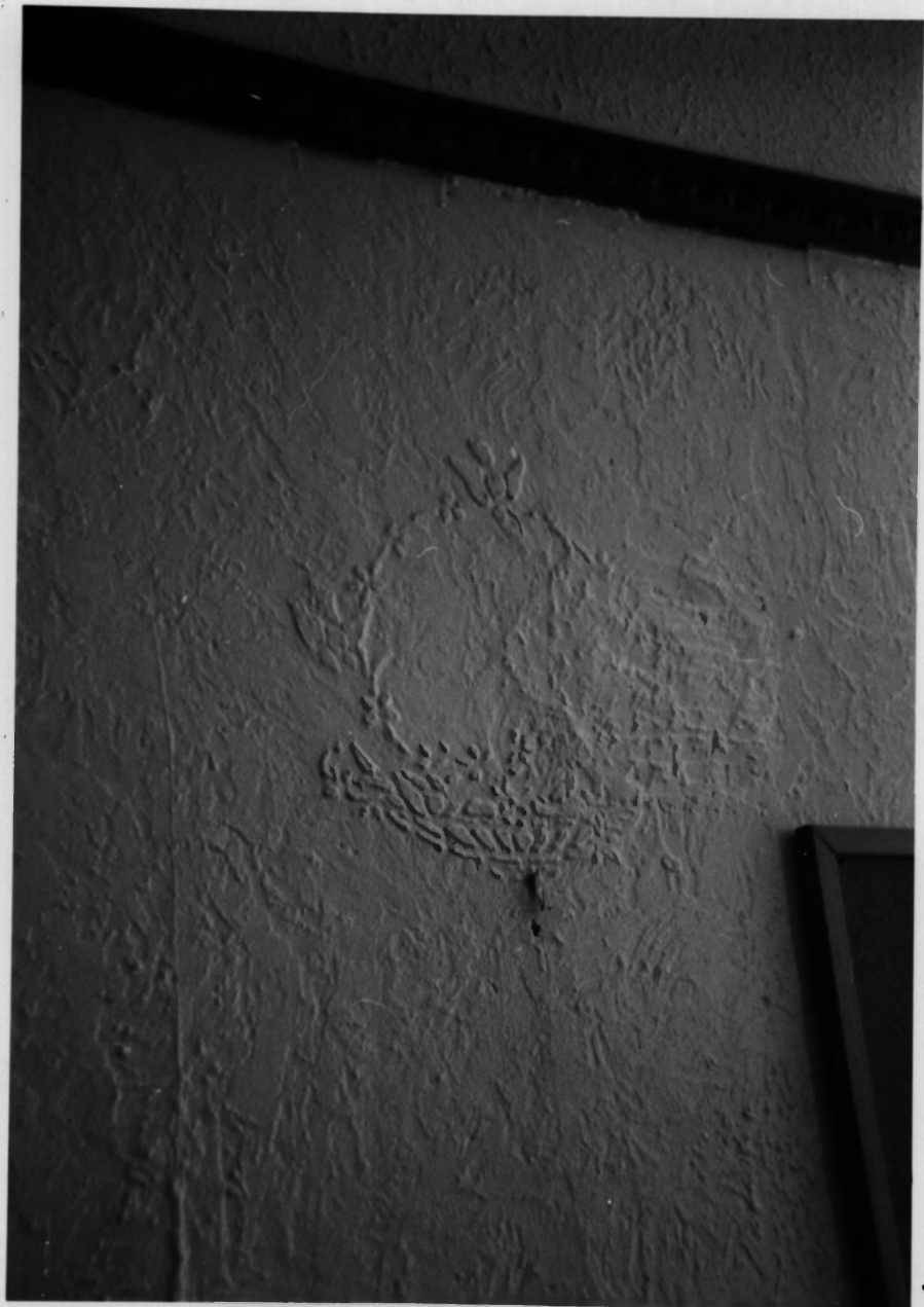
THE BEA HOUSE, PASSAIC COUNTY, HAWTHORNE, NJ #23
