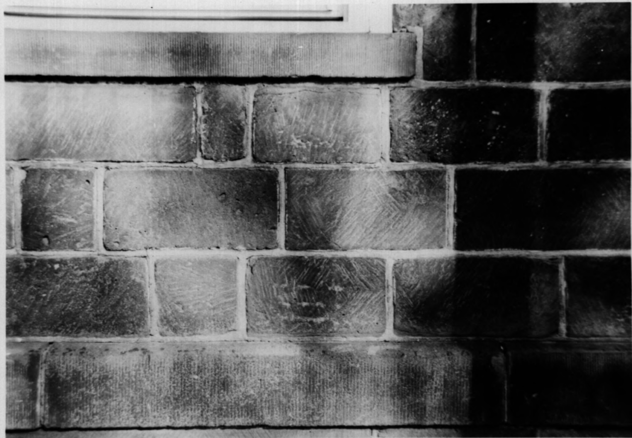
THE REA HOUSE, PASSAIC COUNTY, HAWTHORNE, NJ #4 & 31
