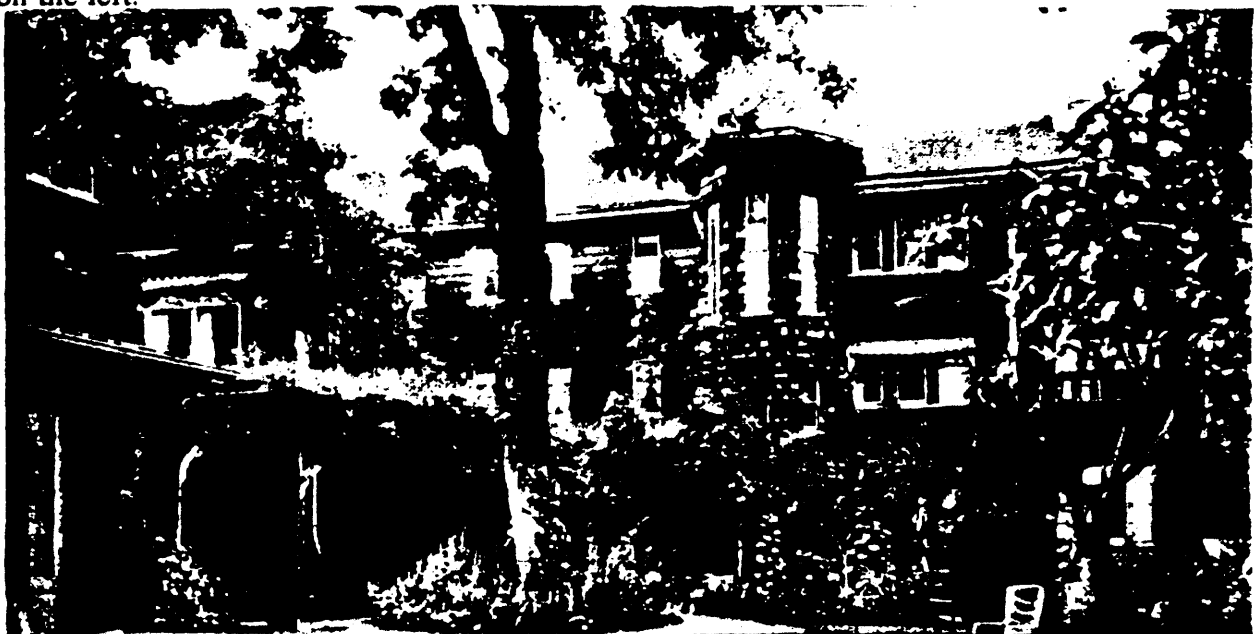
Figure 4 Although Cloyne Court is a large building, four stories plus attic, it fits the tenets of the Hillside Club by being entirely clad in unpainted brown shingles, set sufficiently back from the streets to allow for large trees and shrubs and its wide "U" shape provides for a generous south facing garden courtyard giving testimony to the attention paid to gardens and the quiet enjoyment of nature which was an important part of "building with nature".
