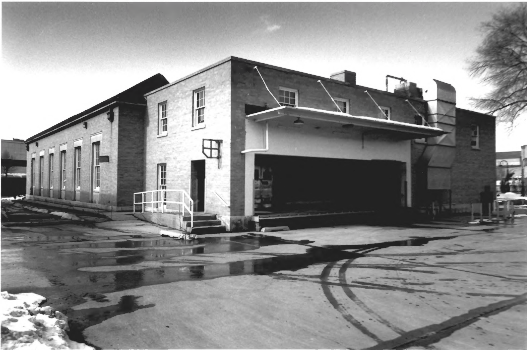
SUGAR HOUSE POSTAL STATION SALT LAKE CITY, SALT LAKE CO., UT PHOTO #2
