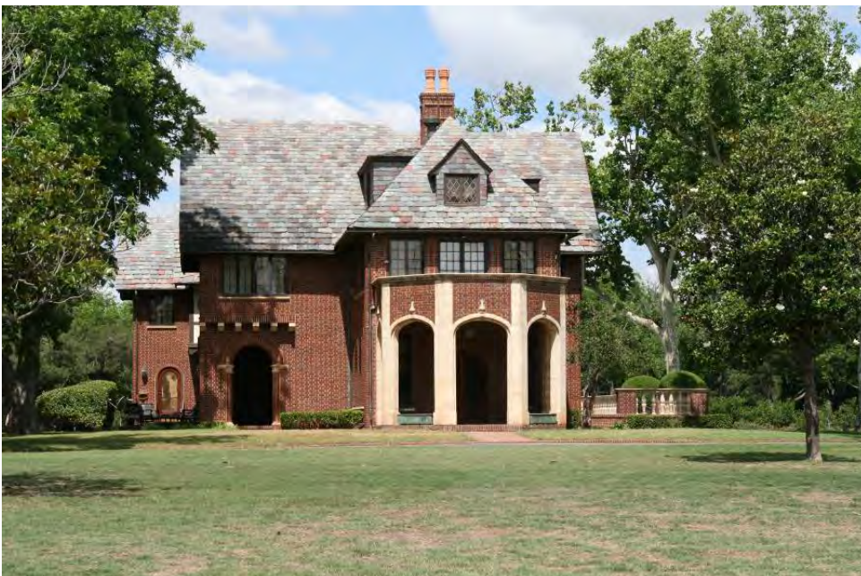
Perkins House, east elevation, camera facing west
