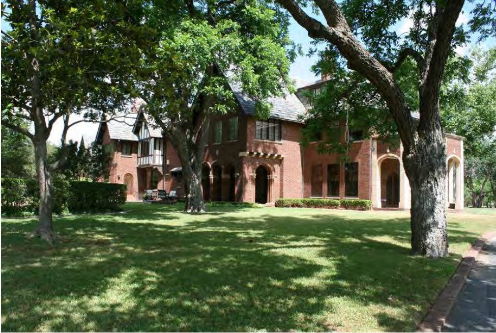
Perkins House, south elevation, camera facing northwest
