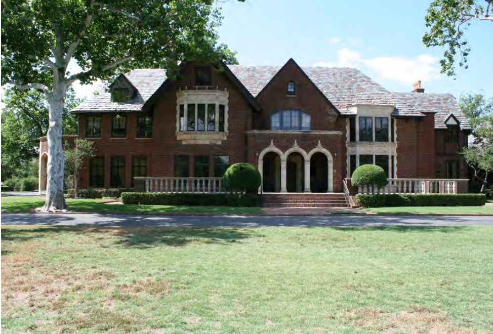
Perkins House, north elevation, camera facing south
