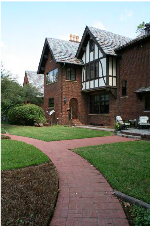
Perkins House, south elevation, kitchen wing and 1998 garage, camera facing west/northwest
