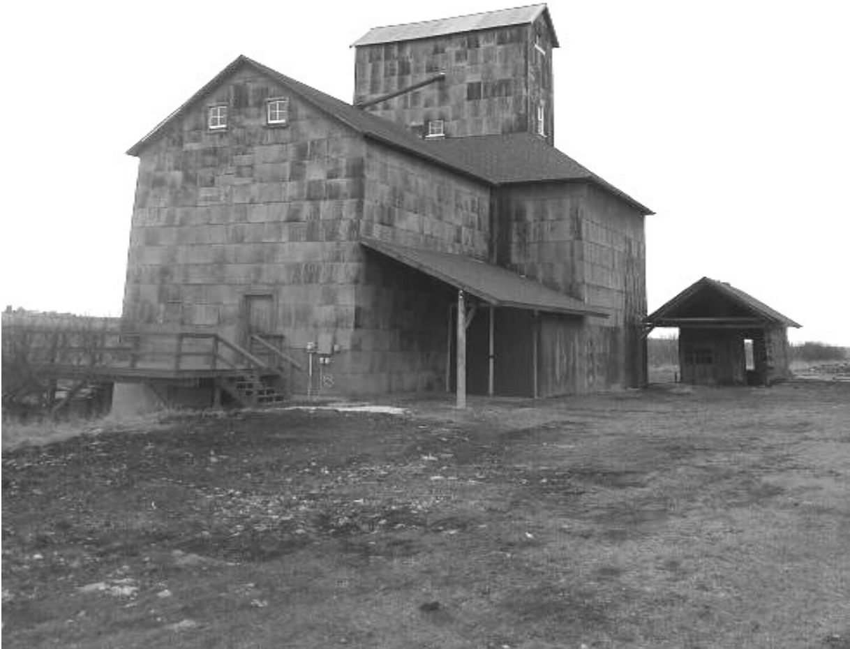
5 of 5. View of the annex, elevator and office from the southeast. Prior to rehabilitation, the East wall of the elevator was deteriorated and its foundation collapsed exposing the interior of the elevator. Now, the overhang has been re-constructed, a new wall and foundation were put in place. The annex, which consisted of four grain bins with four small ports for access into the bins, was opened up. A door and a deck were added. (Ross Iowa Grain Elevator, Ross, IA. Audubon County, Iowa. Photographer, Robert Nelson, owner. Photo taken March 2017.)
