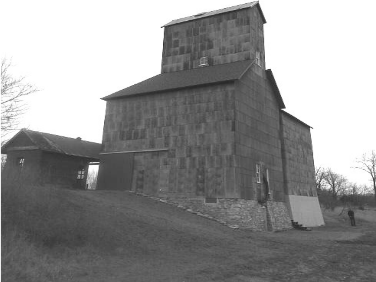
2 of 5. View of the elevator as seen from the northwest. Most of the visible portions of the limestone foundation are original, all portions below grade had collapsed. The collapsed portions of the foundation have been reconstructed and stabilized with new concrete footings. Rotten wood was replaced throughout the exterior and interior, reclaimed windows were used, new doors were built, steel siding reattached, and a new roof was installed. (Ross Iowa Grain Elevator, Ross, IA. Audubon County, Iowa. Photographer, Robert Nelson, owner. Photo taken March 2017.)
