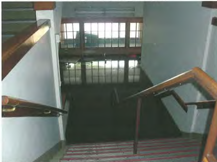
Looking down from the second floor at flooded northwest vestibule entrance during the 2008 flood. The doors are submerged. Only the transom over the doors is visible here (reflected in the flood waters also). The Collection of Jo Ellen Johnson.
