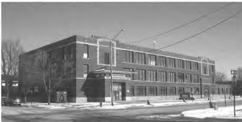
Figure 2 Grant Vocational High School, 2014. The 3 rd story areas over the two entrances framed by white masonry are going to be returned to their original appearance; the roofline arch is going to be rebuilt. Tallgrass Historians L.C.
