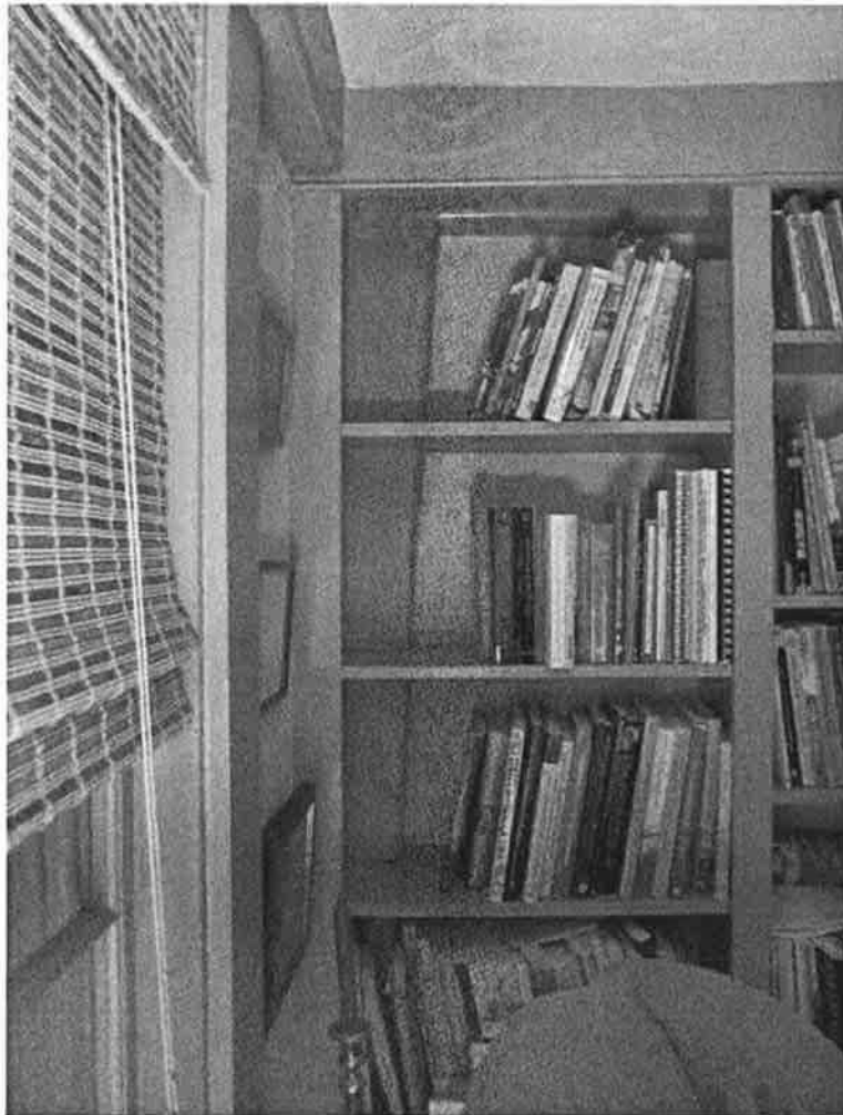
9. First Period Chamber, one of three flared corner posts
