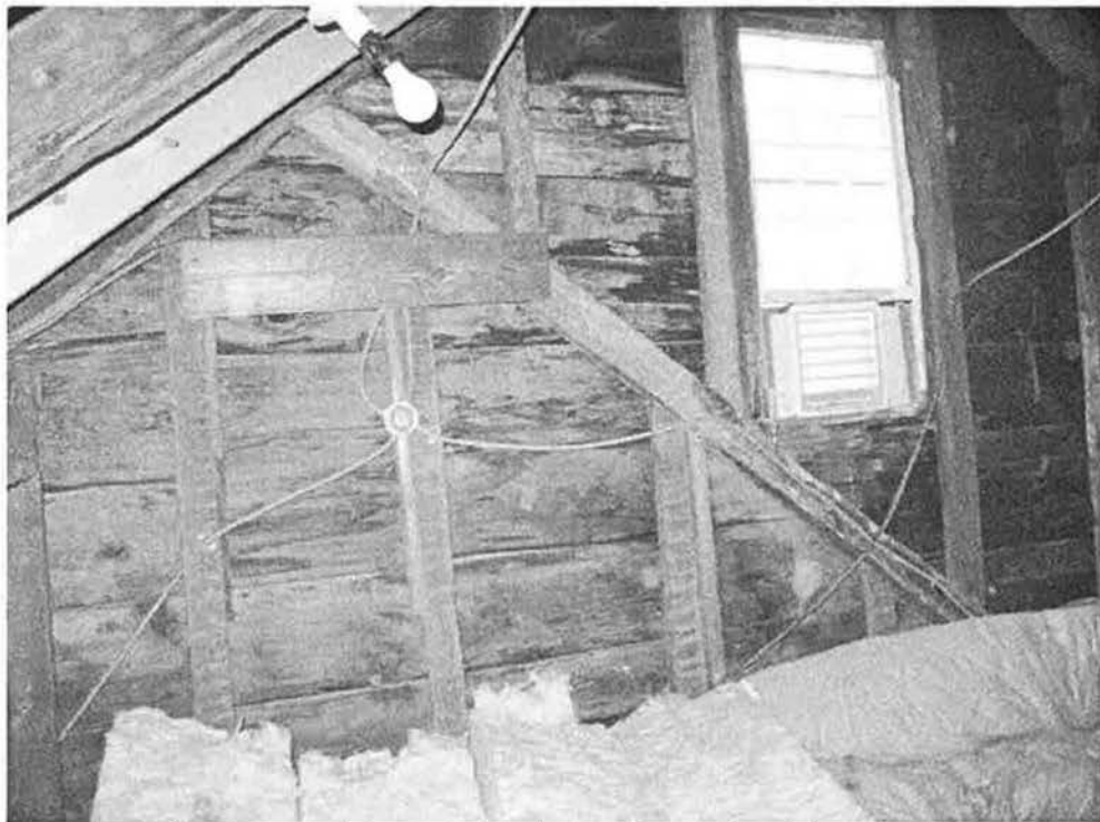
6. Attic, west gable end showing rafter of saltbox roof
