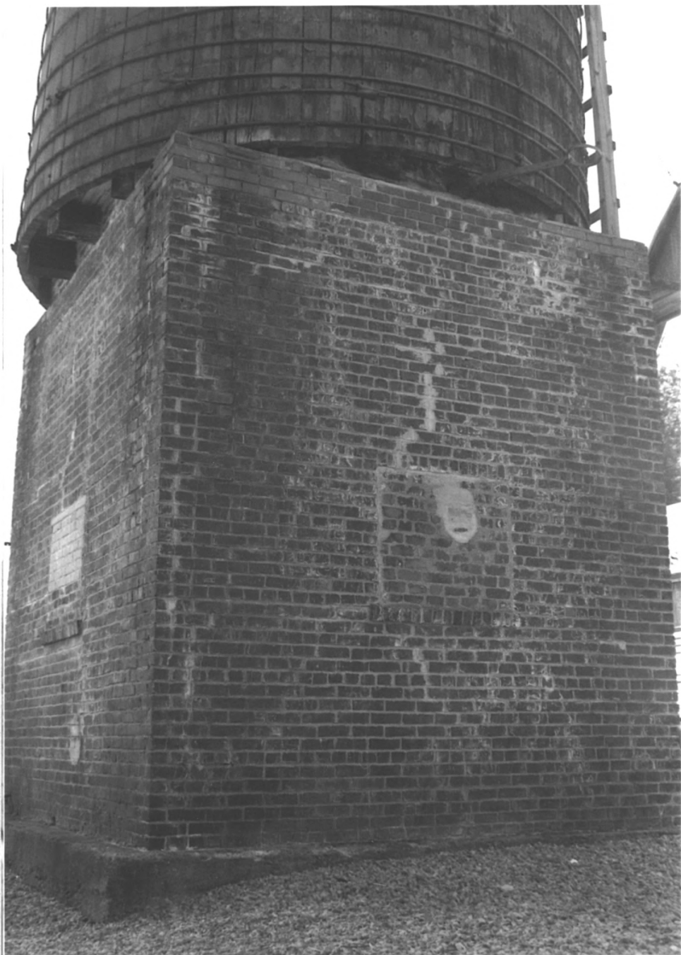
NS-MORRIS WHIPPANY WATER TANK
