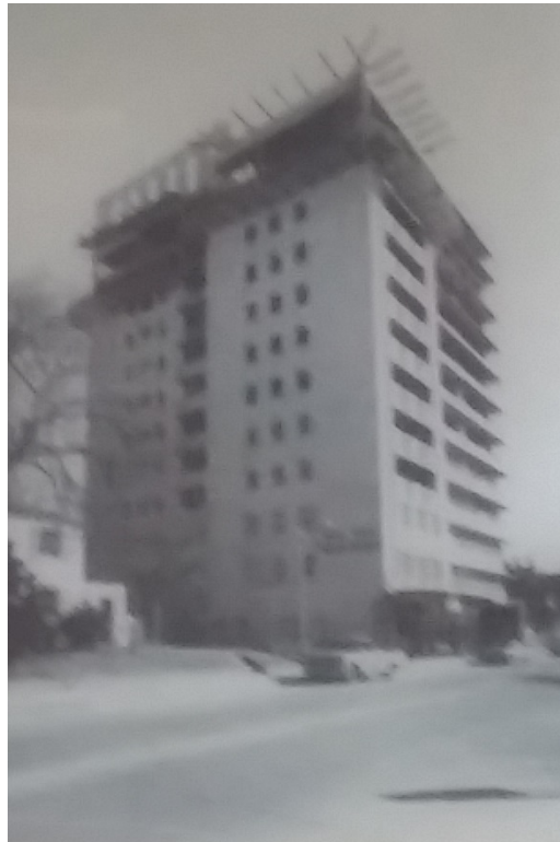
The nearly completed upper floors circa 1969 (Courtesy of Blue Cross Blue Shield of Oklahoma)
