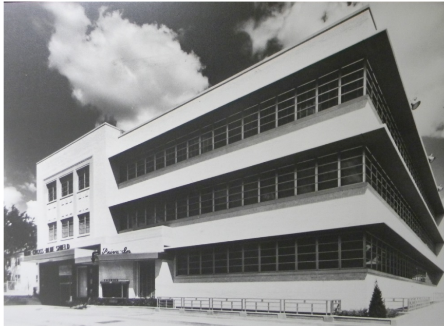
The completed first three floors of the building circa 1954, shortly after construction. (Photo courtesy of the Owner)
