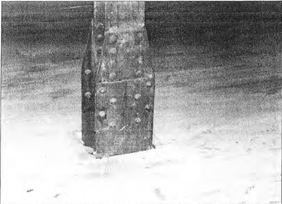
Figure 3: Column connection and demising point (Jacobsen, 2008)
