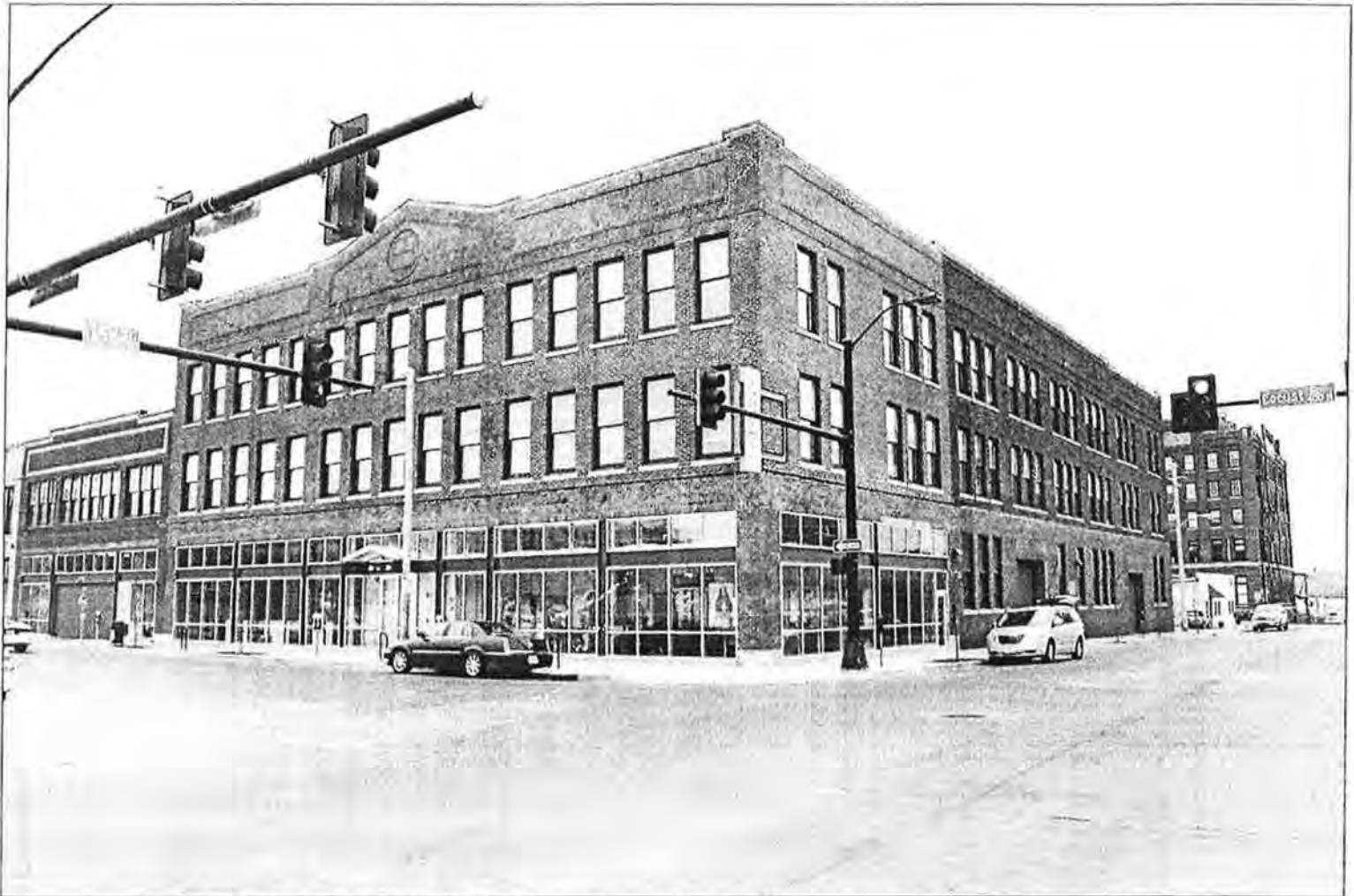
Figure 2: 1436 (left) and 1442 (right) Locust Street, looking southeast (Jacobsen, 2015)
