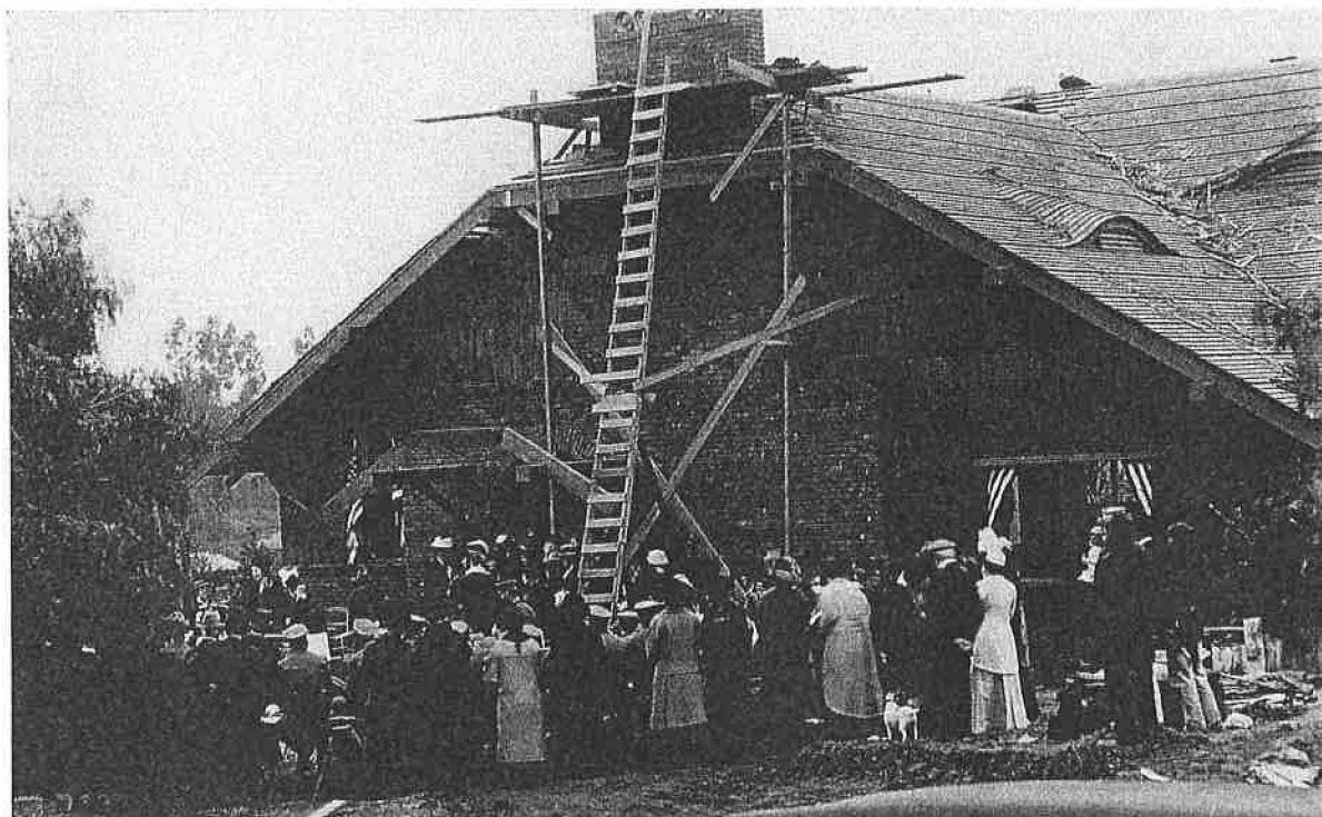
Laying the cornerstone January 8, 1915. (Courtesy of the Murdock family collection)
