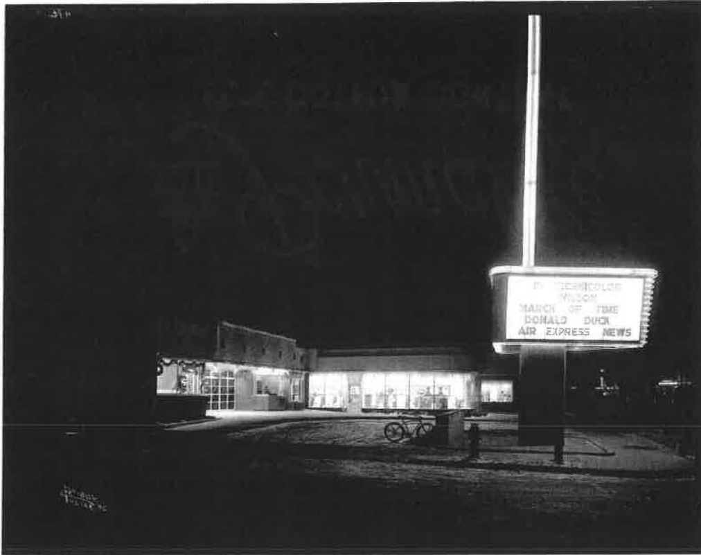
Circa 1945. Garland Theater. West (side) and south (front) facades. View: looking east. Source: Northwest Museum of Arts & Culture.
