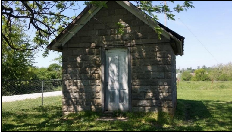
Figure 5: East elevation of caretaker's building (Jan Shupert-Arick, 2018).
