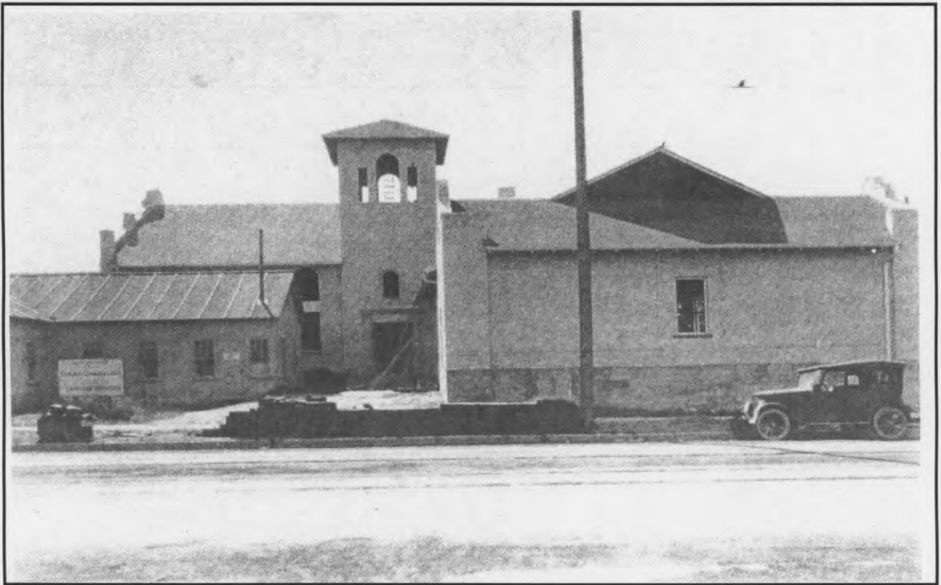
Figure 3: Sixth Avenue Community Church construction site 1923-24, camera facing south. Note temporary one story building to left side where congregation met during construction of permanent building. Trolley tracks and paved street gave good access to neighborhood from downtown Denver.
