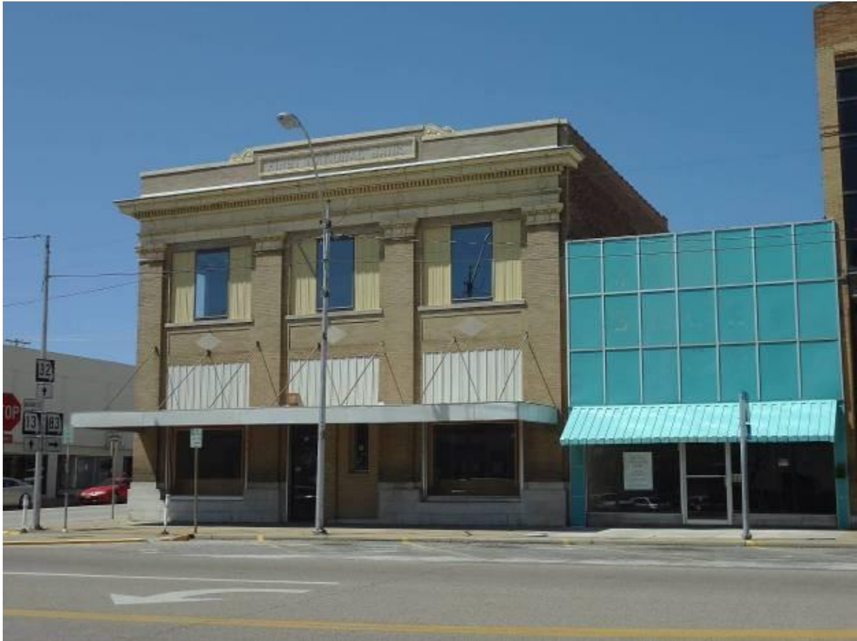
Photo 2. Façade, south wall.
