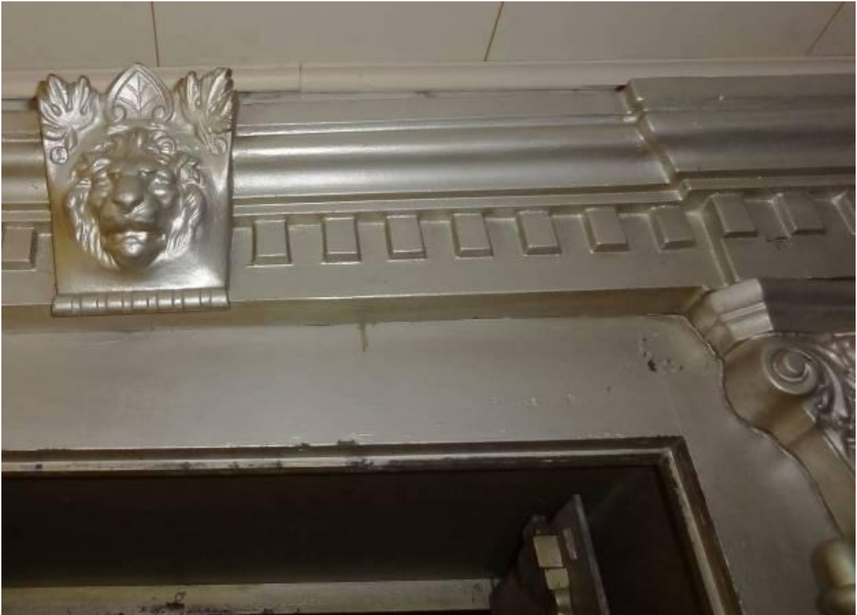
Photo 14. First floor, west side, original bank safe.
