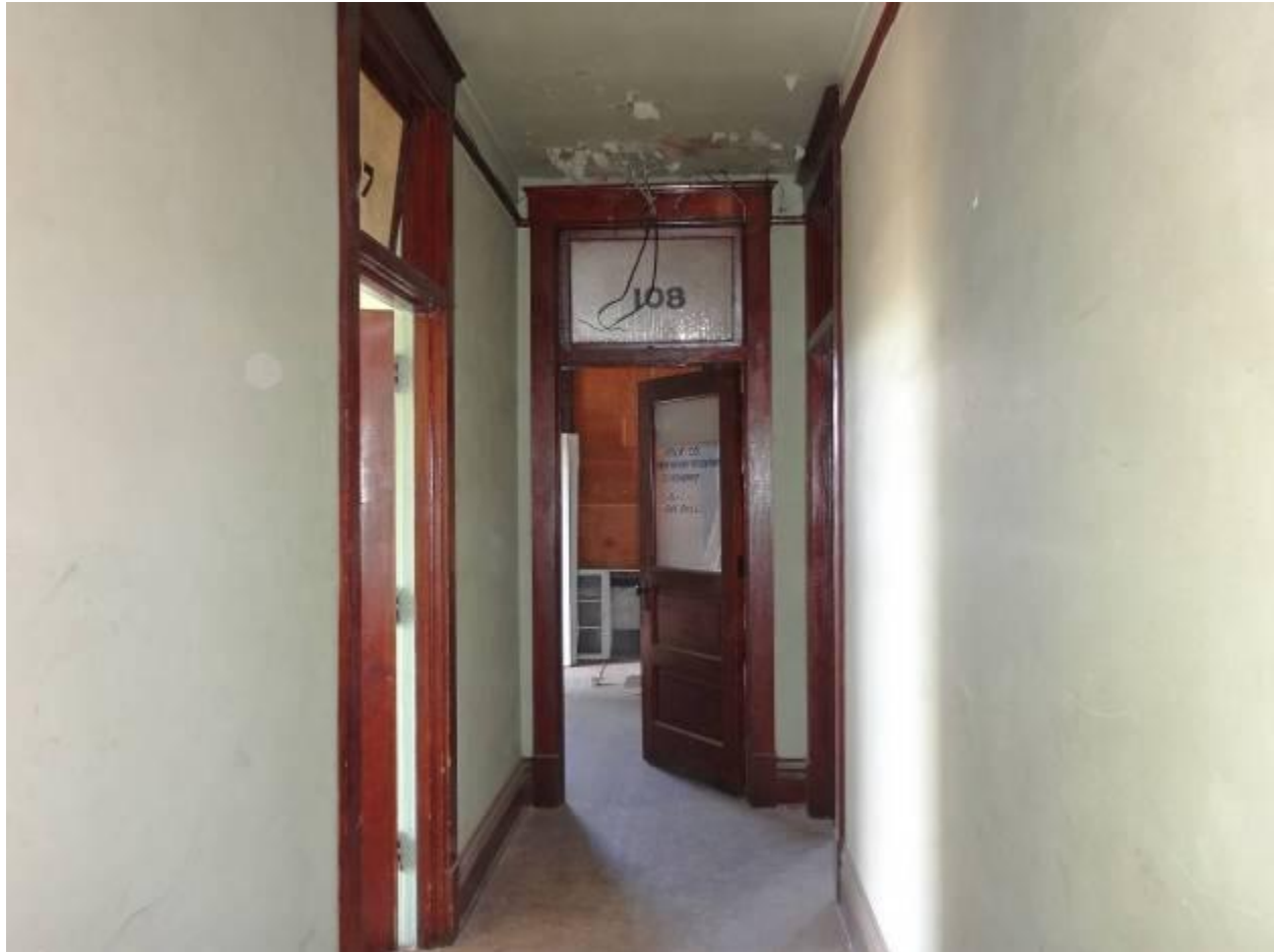
Photo 8. Second floor, north end of hallway.
