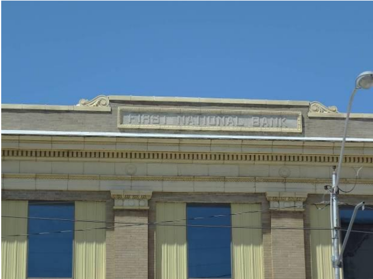
Photo 3. Façade detail—name plate.
