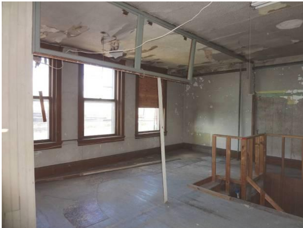
Photo 7. Second floor, back wall.
