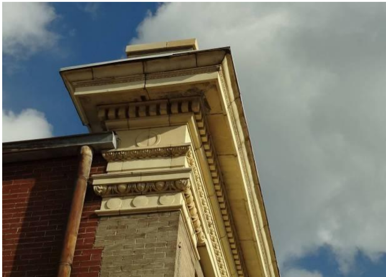
Photo 4. Northwest corner—terra cotta cornice.
