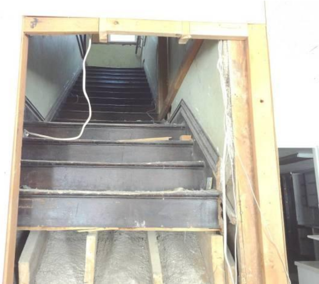
Photo 11. First floor, remaining original stairs to second.
