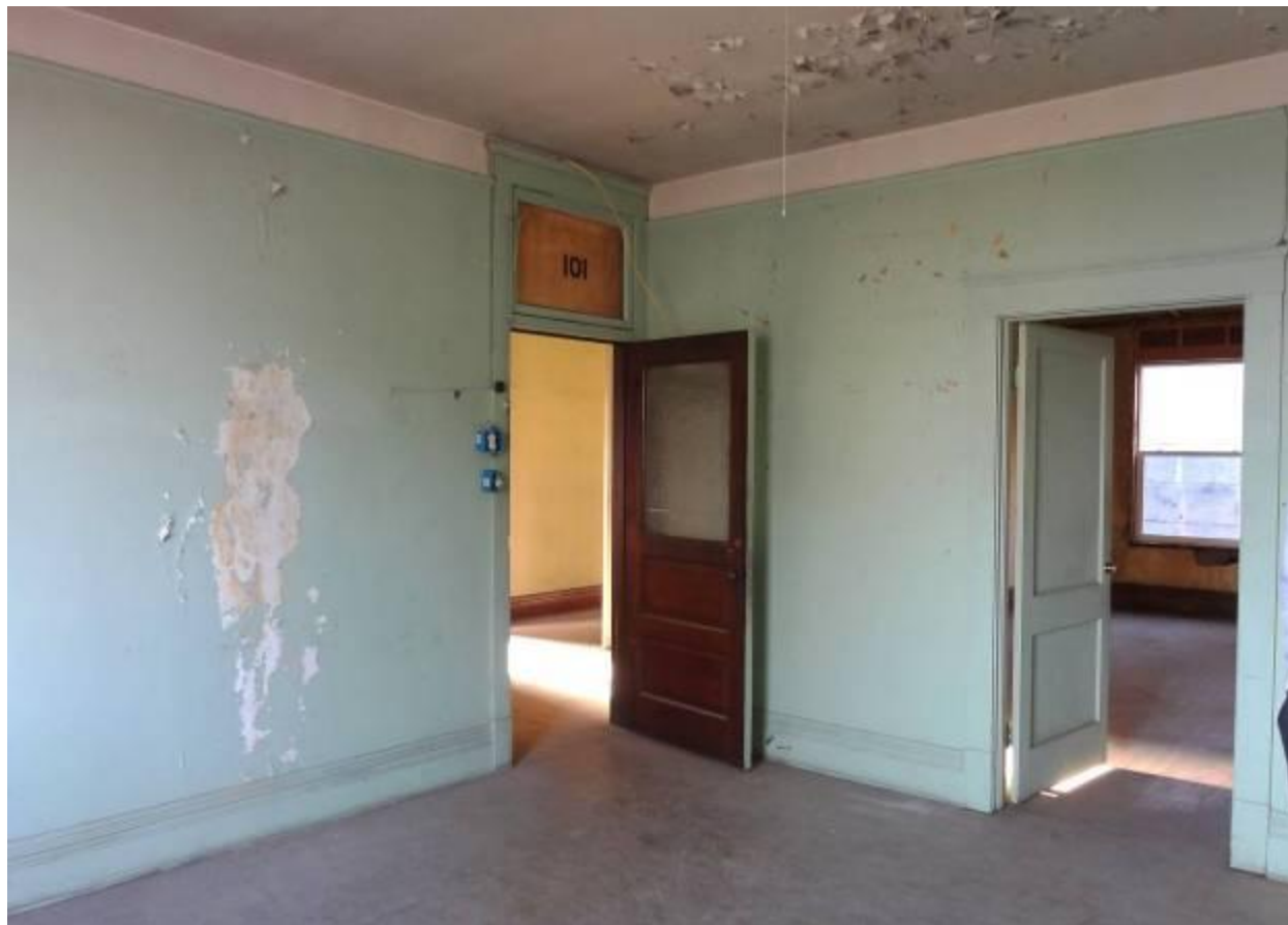
Photo 9. Second floor, front office.
