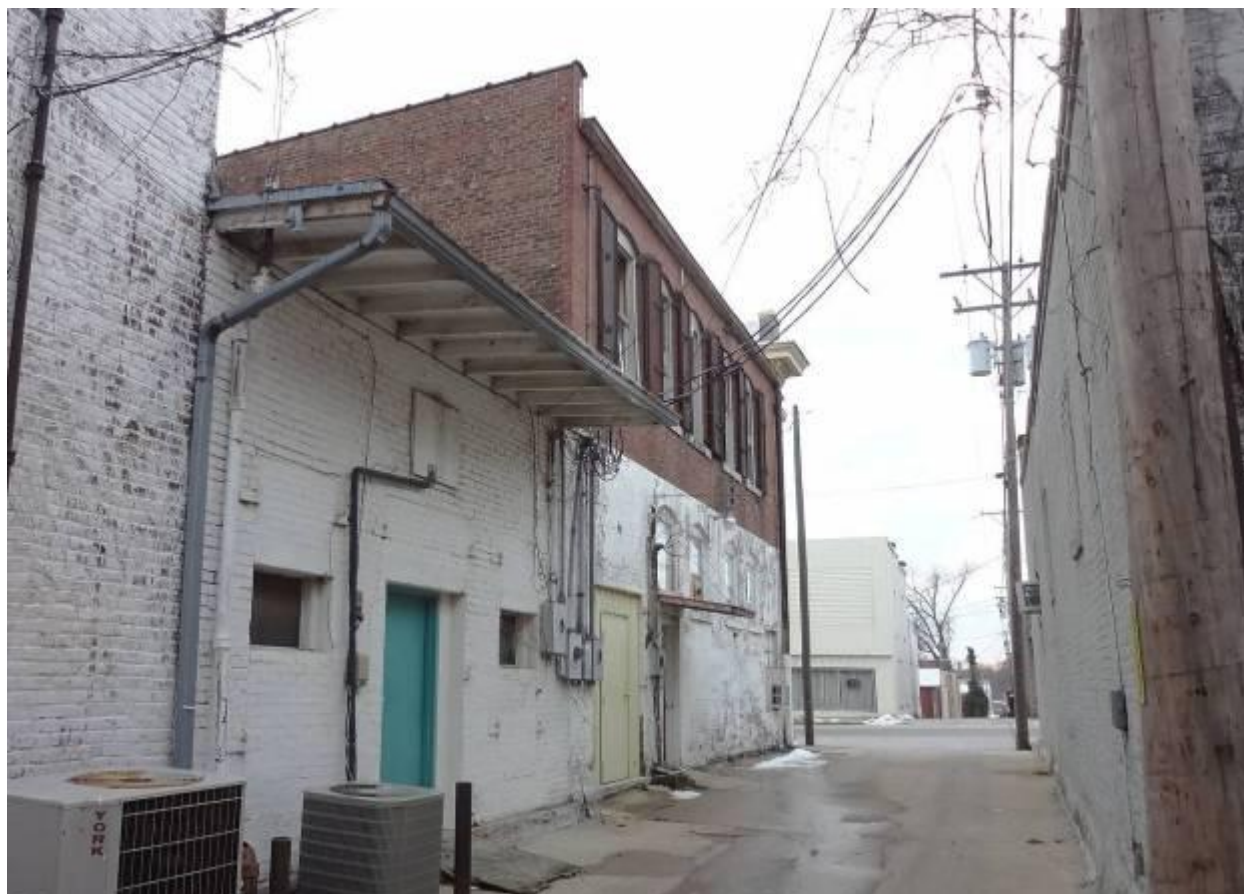
Photo 6. North (back) wall, from the east.
