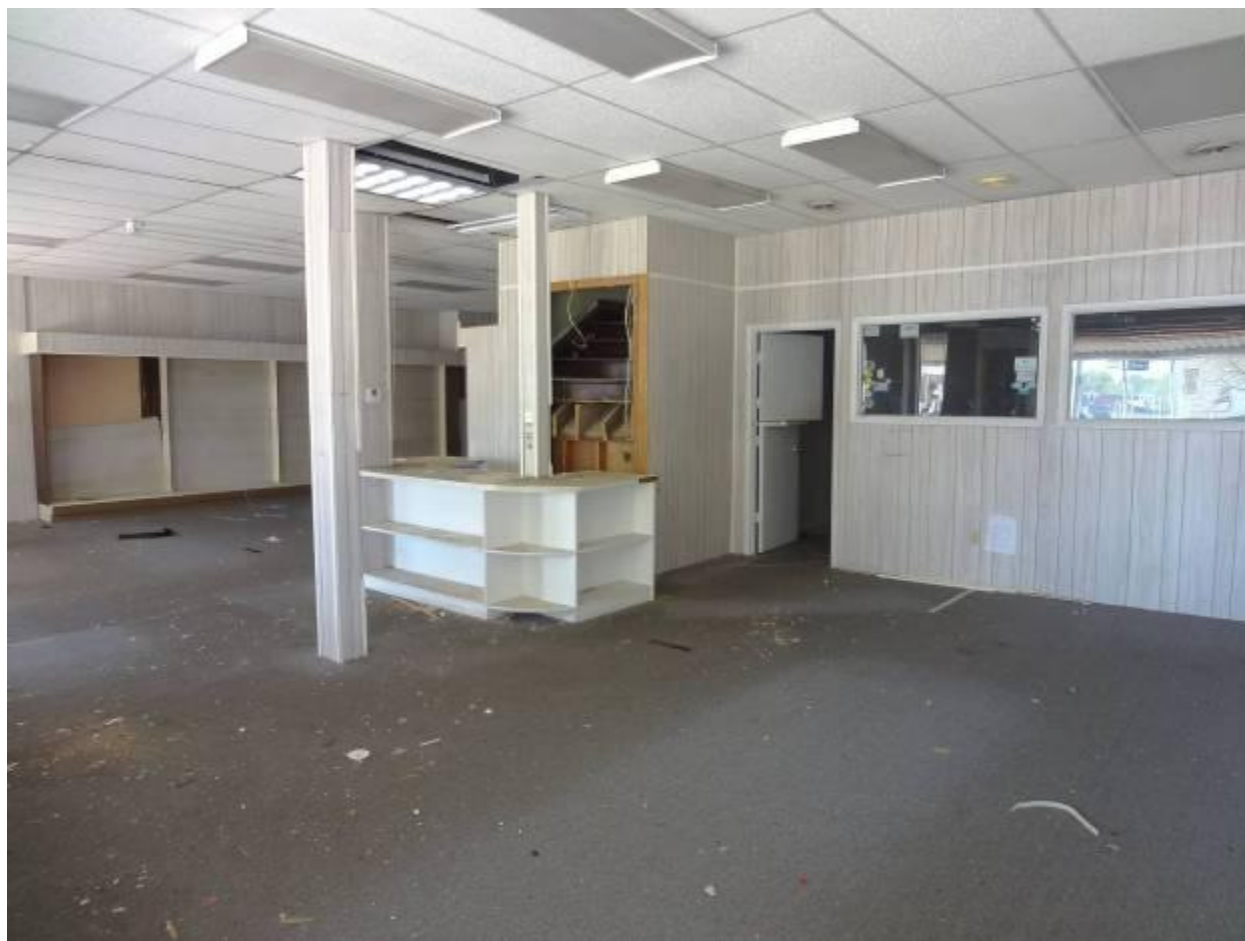
Photo 12. First floor, front rooms, looking west.
