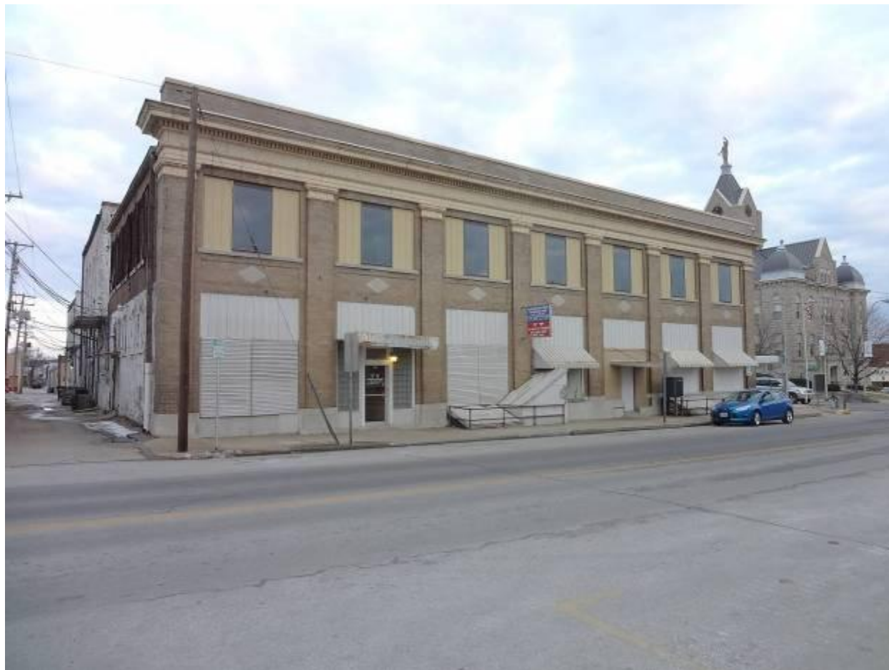
Photo 5. West wall and northwest corner.
