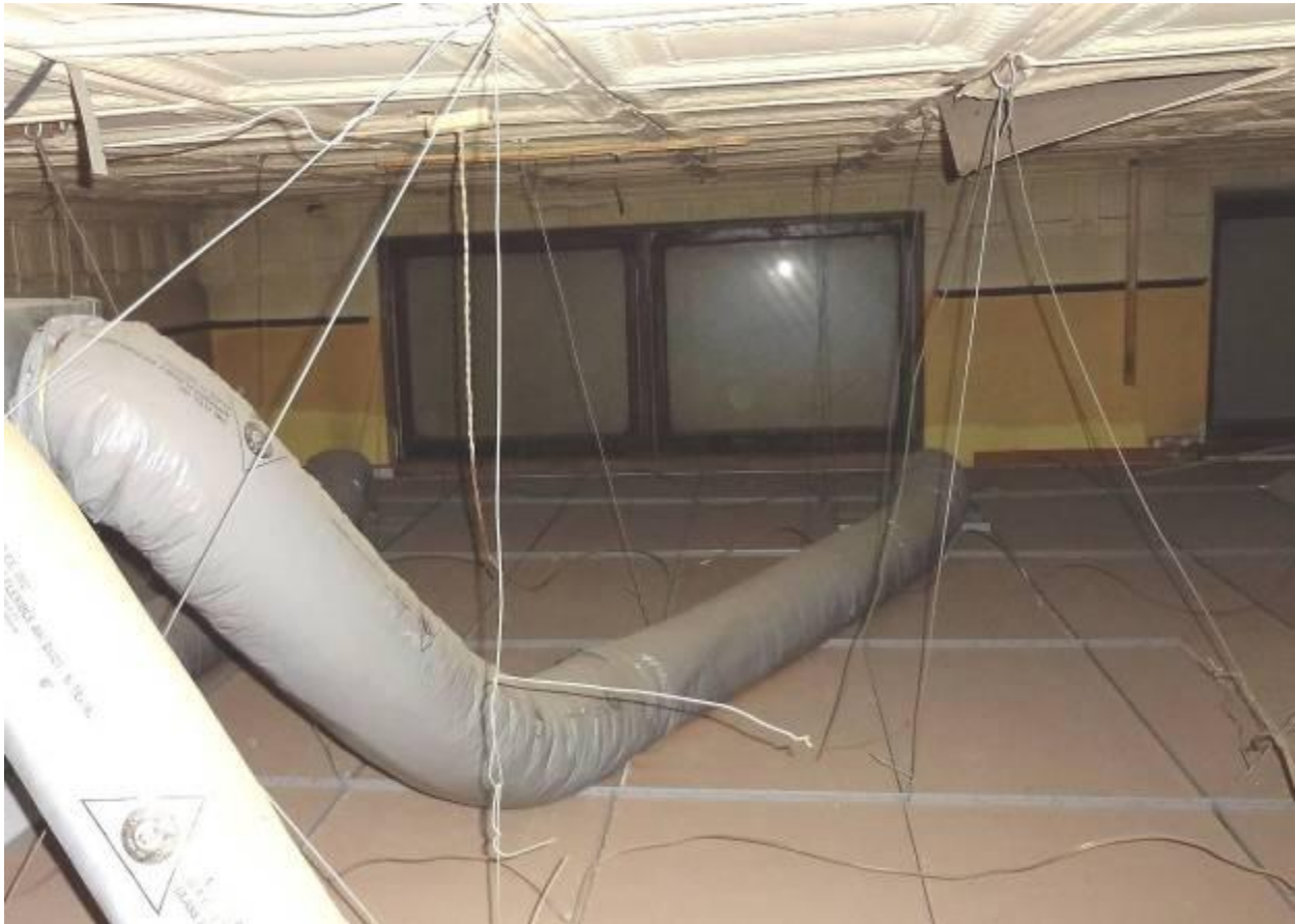
Photo13. First floor. Front transom windows and early metal ceiling above suspended ceiling.
