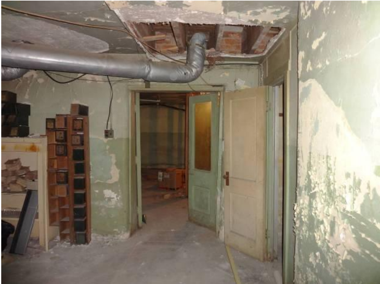
Photo 16. Basement, south end.
