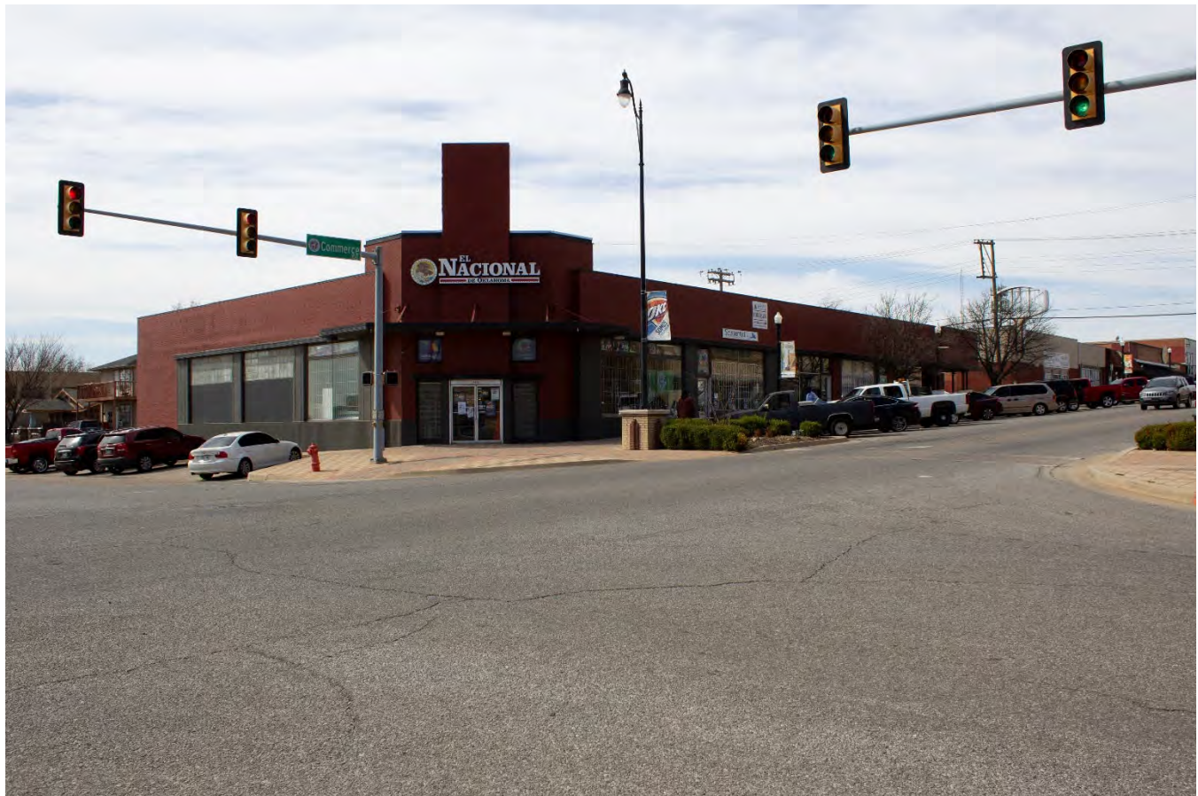
OK_Oklahoma County_Capitol Hill Commercial Historic District_0013
