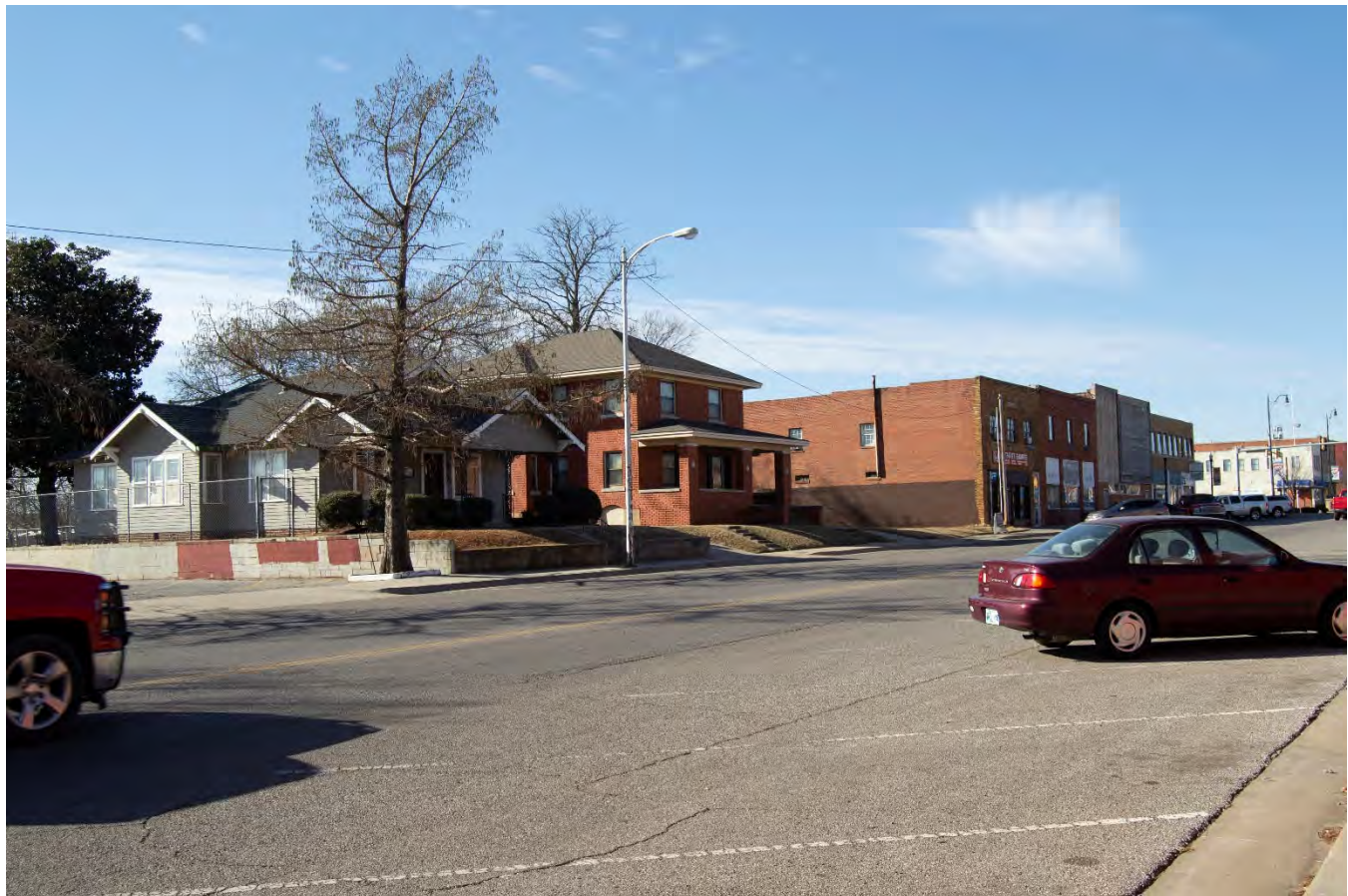
OK_Oklahoma County_Capitol Hill Commercial Historic District_0001
