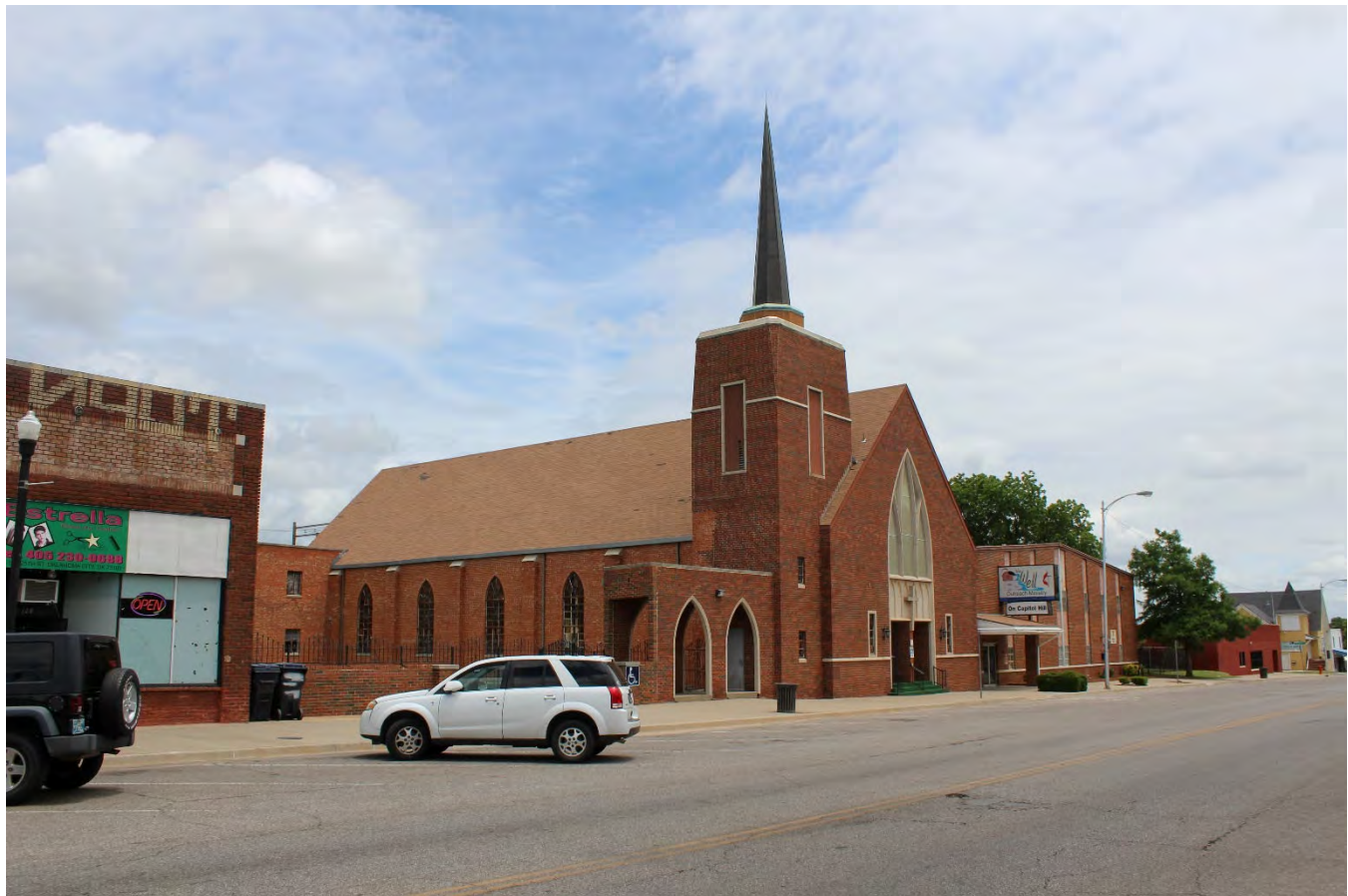
OK_Oklahoma County_Capitol Hill Commercial Historic District_0003
