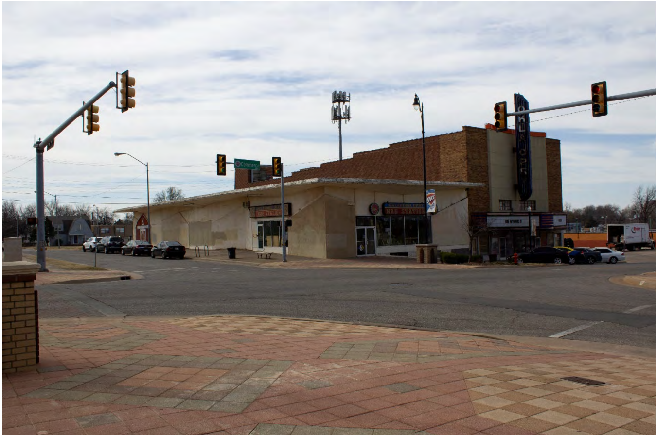
OK_Oklahoma County_Capitol Hill Commercial Historic District_0015
