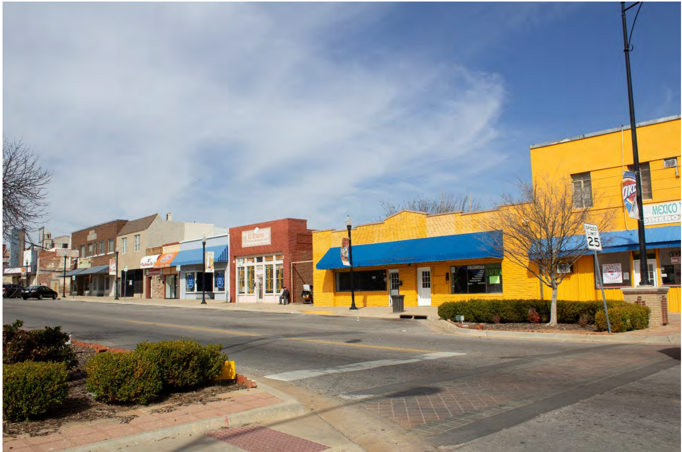
OK_Oklahoma County_Capitol Hill Commercial Historic District_0009
