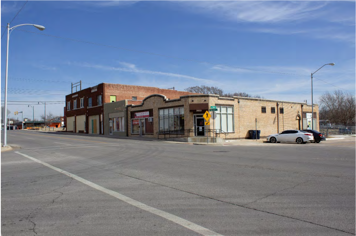
OK_Oklahoma County_Capitol Hill Commercial Historic District_0005
