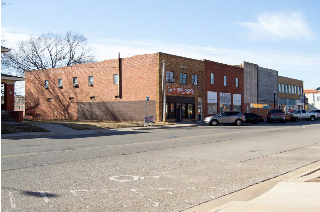
OK_Oklahoma County_Capitol Hill Commercial Historic District_0002
