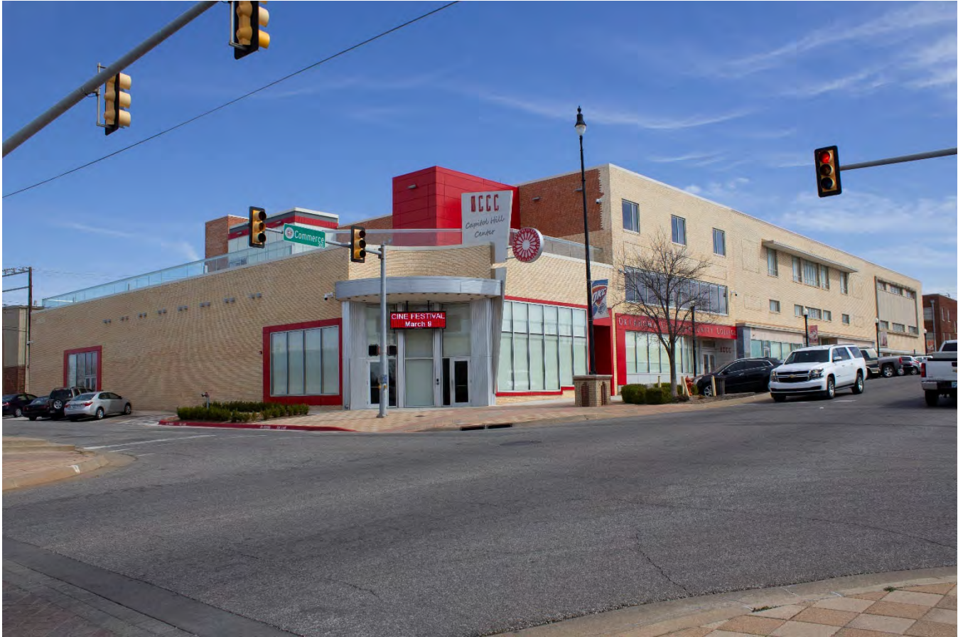
OK_Oklahoma County_Capitol Hill Commercial Historic District_0016
