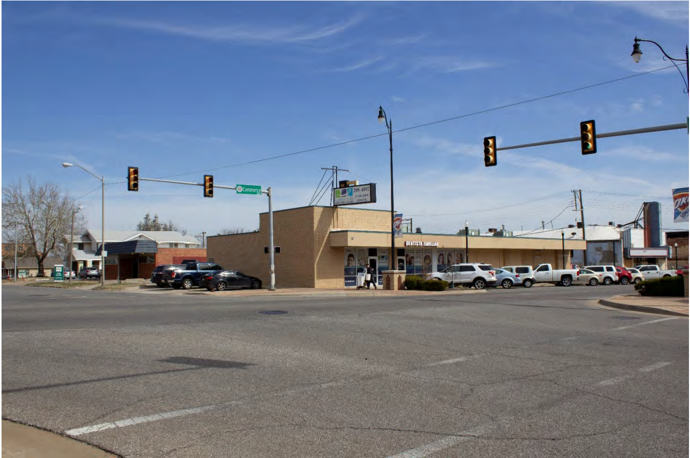
OK_Oklahoma County_Capitol Hill Commercial Historic District_0011
