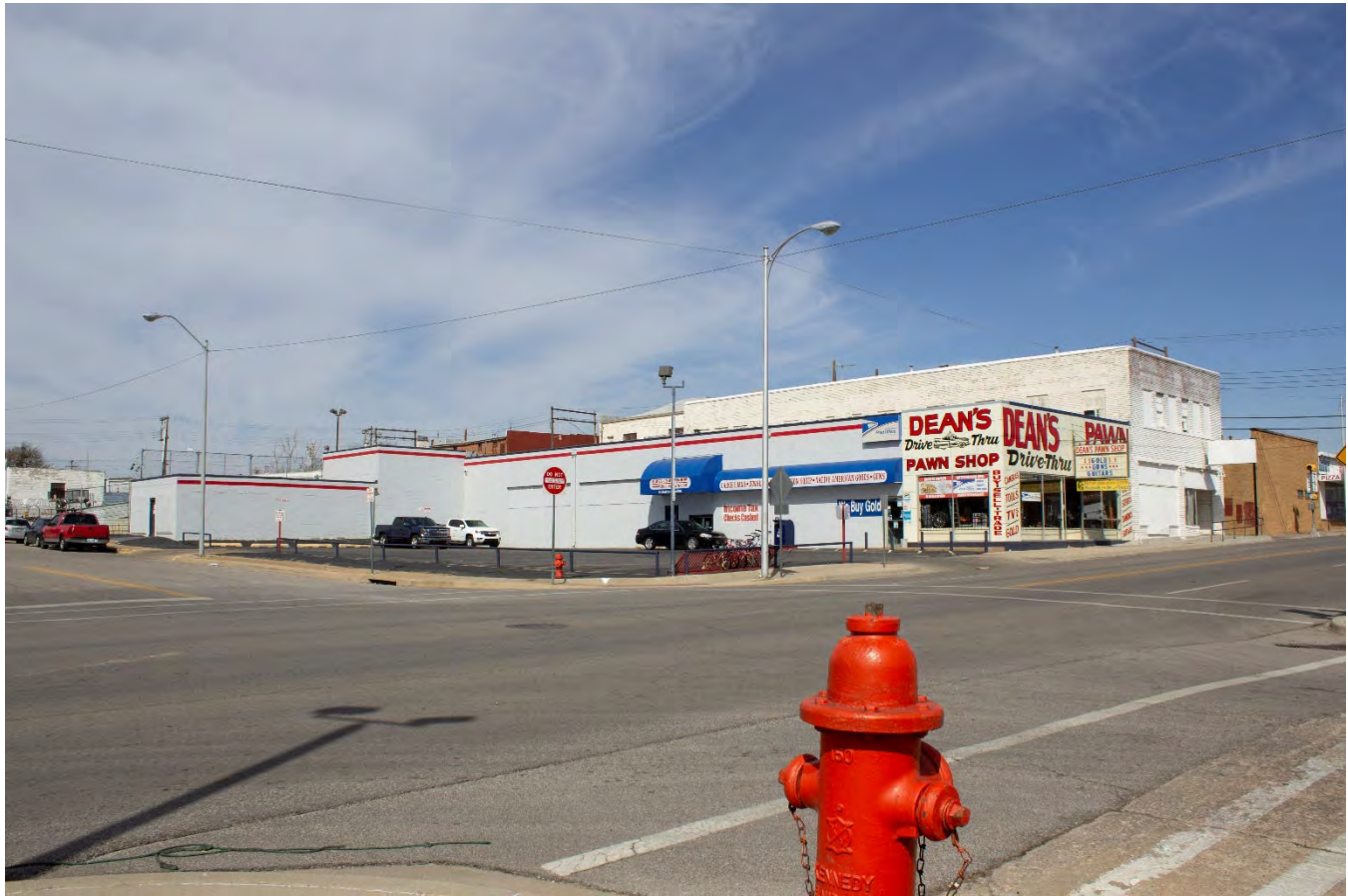
OK_Oklahoma County_Capitol Hill Commercial Historic District_0006
