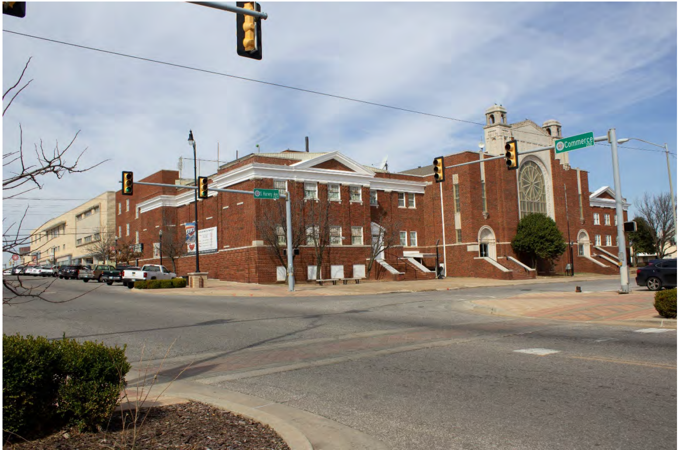
OK_Oklahoma County_Capitol Hill Commercial Historic District_0014
