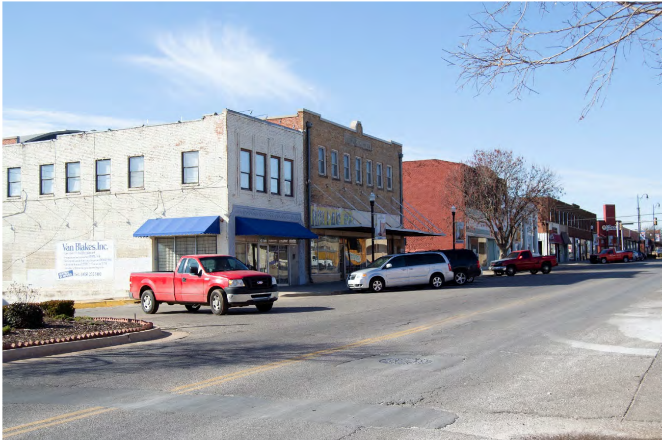
OK_Oklahoma County_Capitol Hill Commercial Historic District_0010
