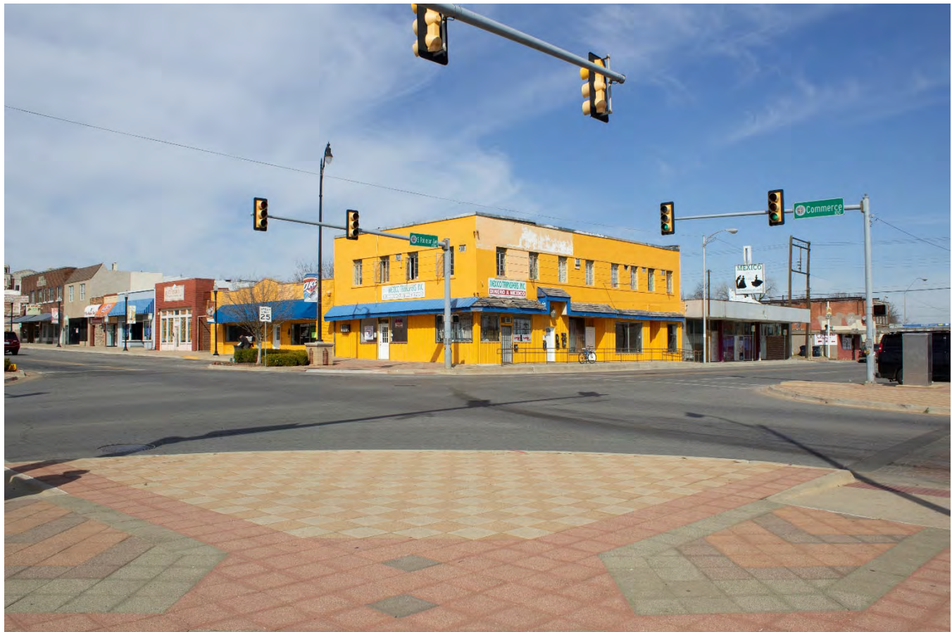
OK_Oklahoma County_Capitol Hill Commercial Historic District_0008
