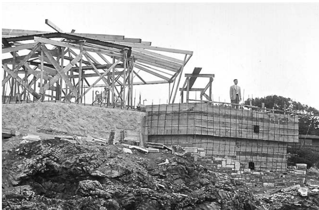
Figure 7 Walker House under construction with first desert masonry wall cladding and Wellington (Hendy) Henderson Jr.
