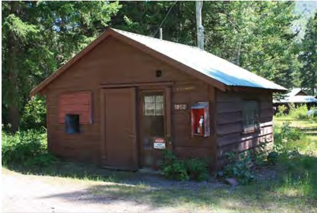
Photo 0027: BC Generator Shed, view to east.
