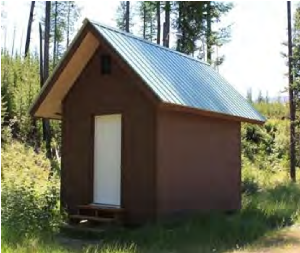
Photo 0031: Solar Storage Shed.
