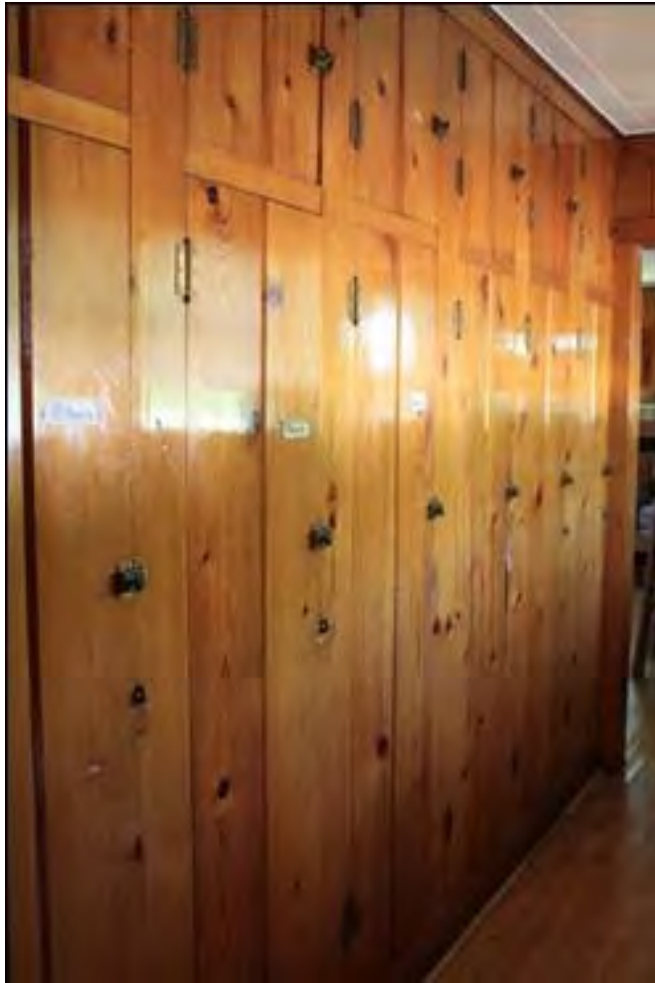
Photo 0018: Bunkhouse/Boys Dorm, Closets.
