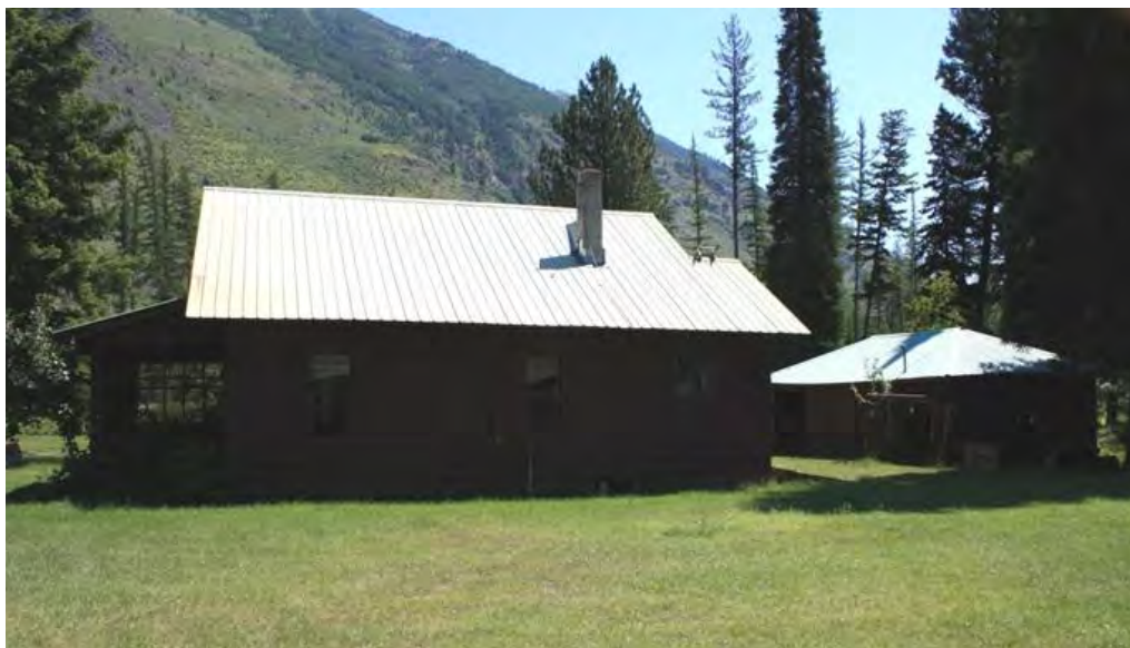
Photo 0005: Below: Ranger House, Ranger House & Garage, view to the east.
