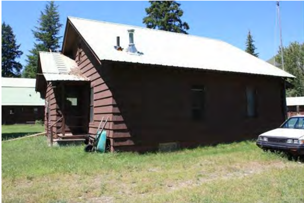
Photo 0004: Above: Ranger House, view to the west.
