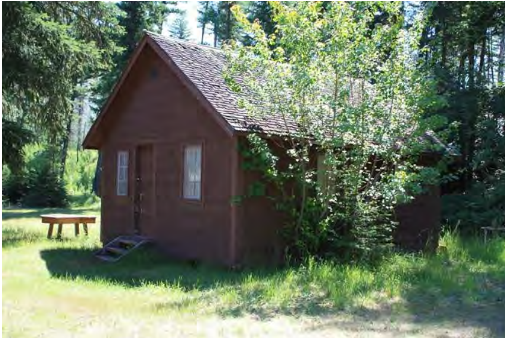
Photo 0025: Fire Cache/Recreation Building, view to southeast.
