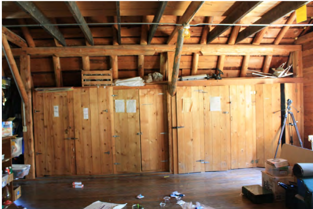
Photo 0013: Below Cookhouse Interior, Attic.
