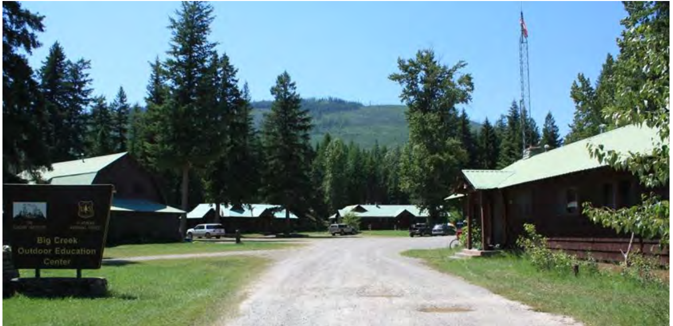
Photo 0001: Big Creek Ranger Station, view to west.
