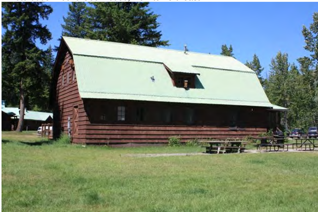
Photo 0009: Below Cookhouse, view to west.
