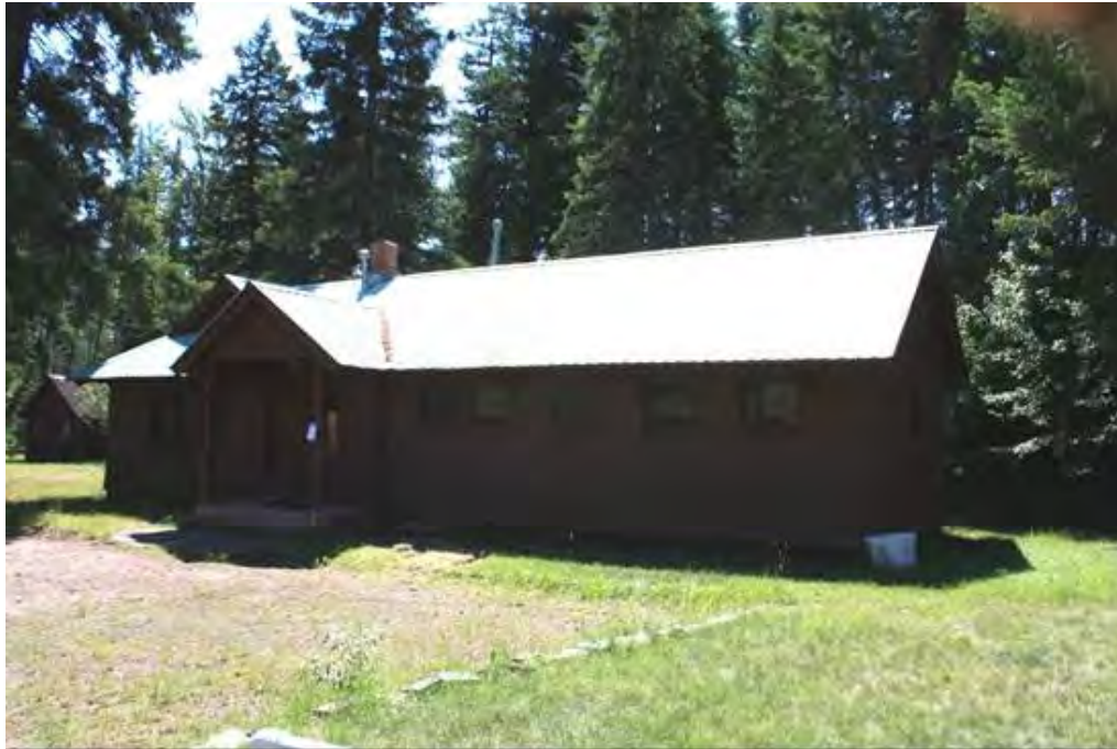
Photo 0014: Bunkhouse/Boys Dorm, view to southeast.
