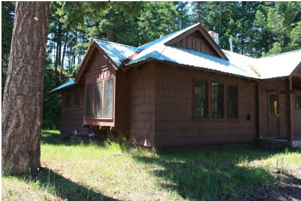
Photo 0015: Bunkhouse/Boys Dorm, northeast corner, view to southwest.
