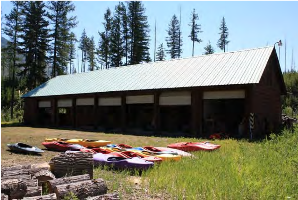
Photo 0029: Fire Compound Garage, view to southeast.
