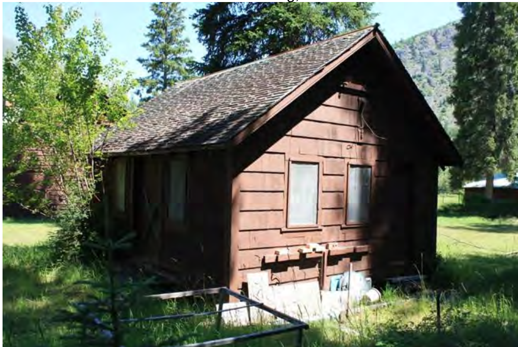
Photo 0026: Fire Cache/Recreation Building, view to northwest.
