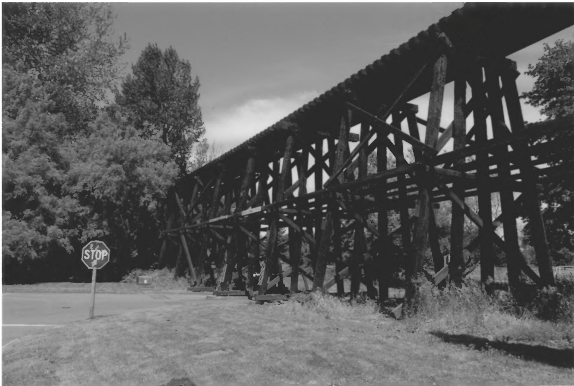
Picture 8. Trestle from park roadway, looking west.
