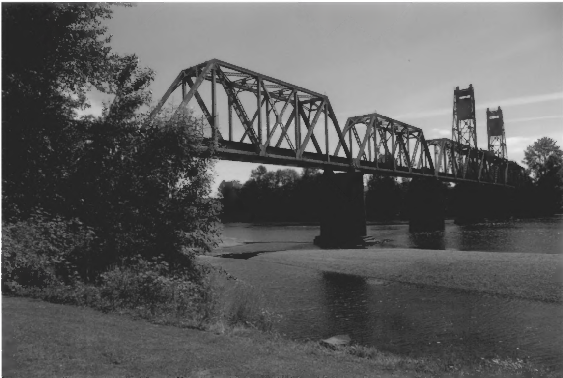
Picture 4. Bridge from west bank, looking east.
