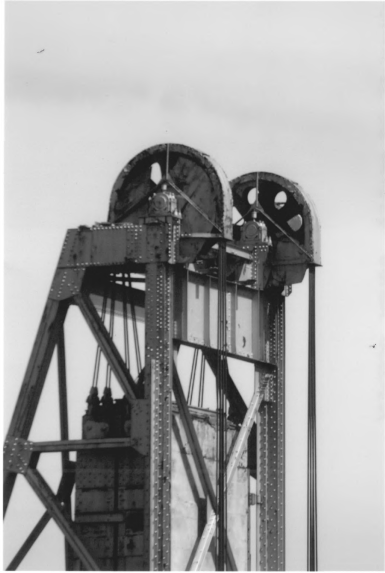
Picture 12. Western lift tower, looking north.
