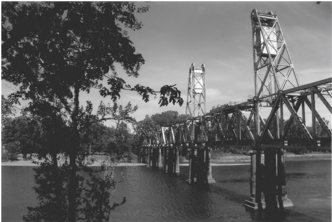
Picture 2. Bridge from east bank, looking northwest.
