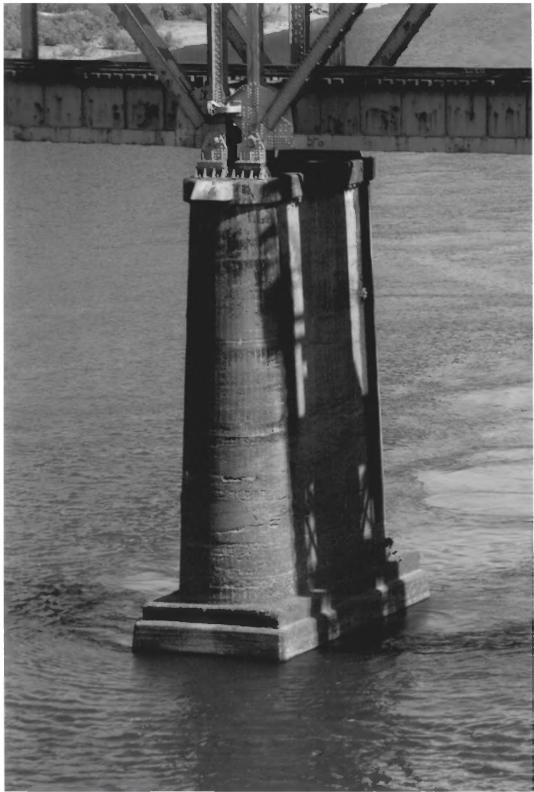
Picture 16. Pier 4, looking north.
