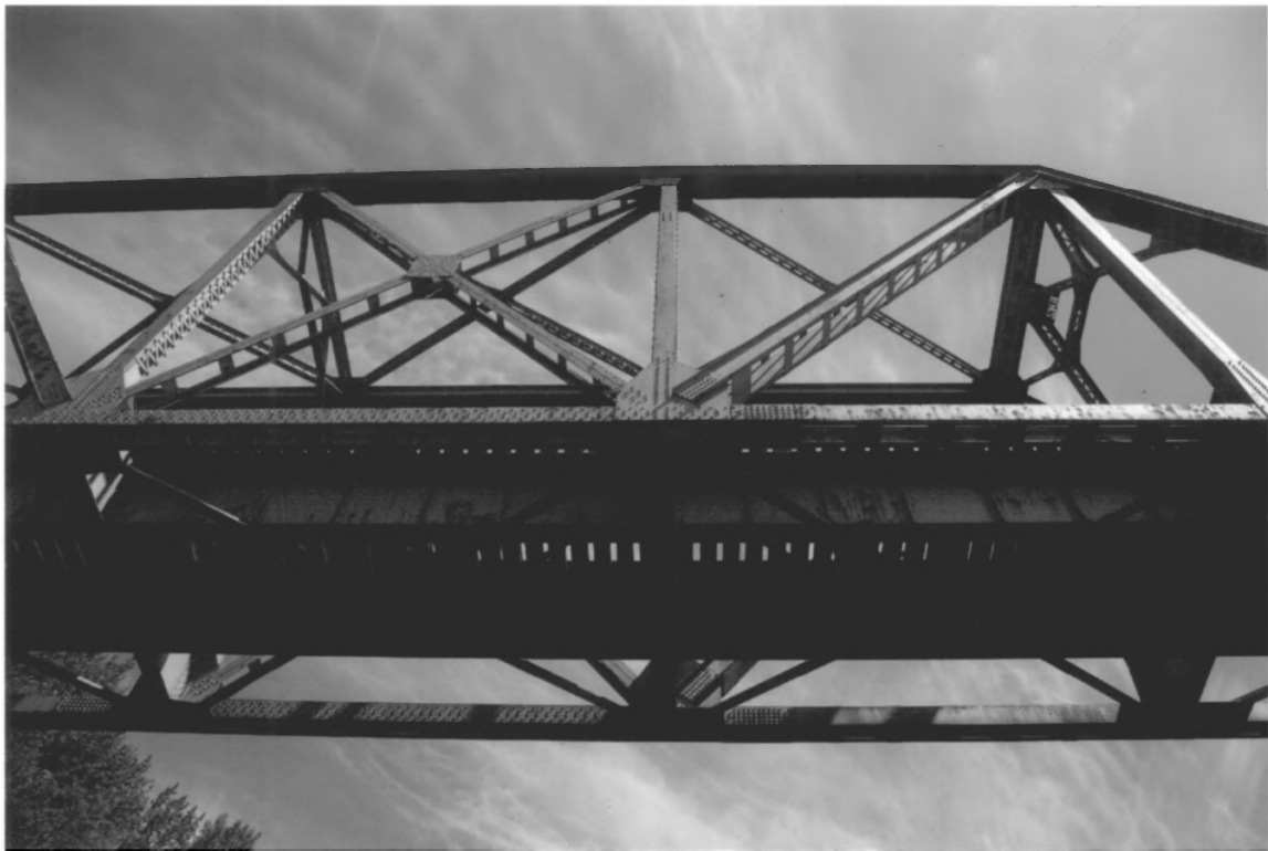
Picture 17. Truss detail, from below.
