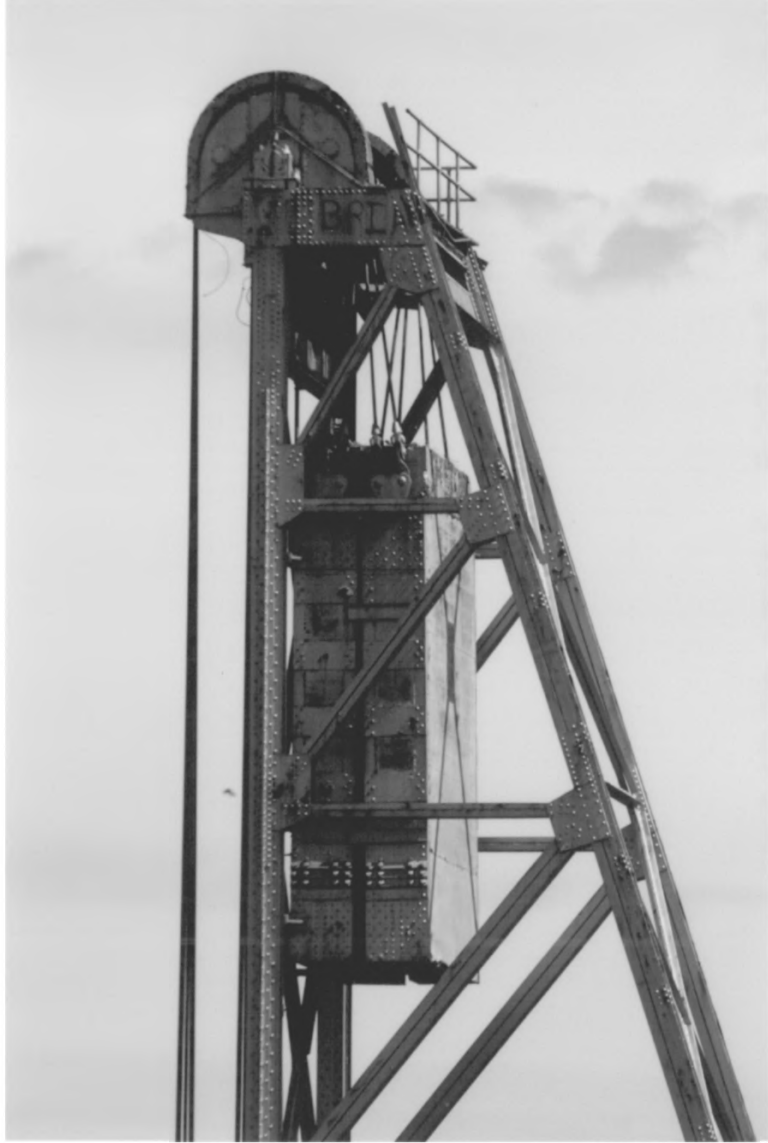
Picture 11. Eastern lift tower, looking north.
