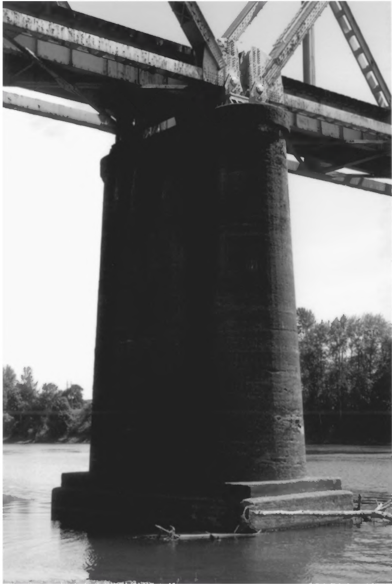
Picture 15. Pier2, looking northeast.
