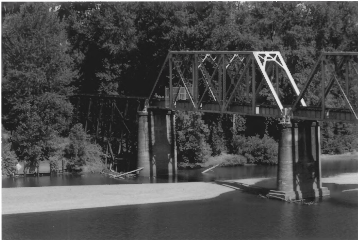
Picture 5. Bridge connection to trestle, looking northwest.
