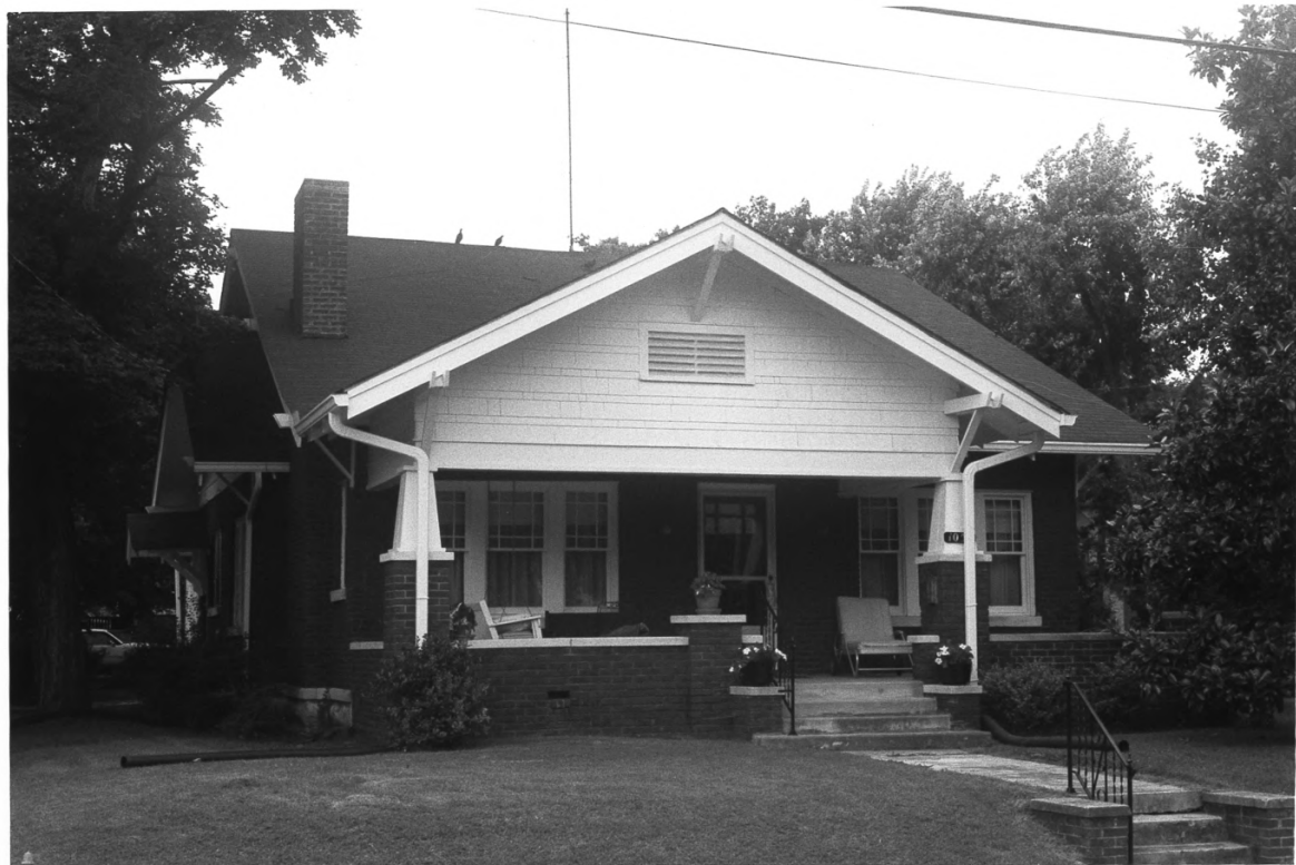
Magnolia St. Historic District, Warren Co. KY PHOTO 4
