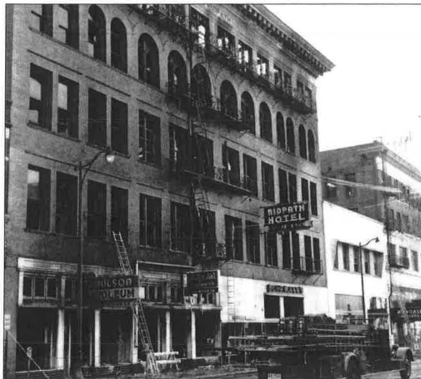
1950 photo of fire damaged Ridpath Hotel
