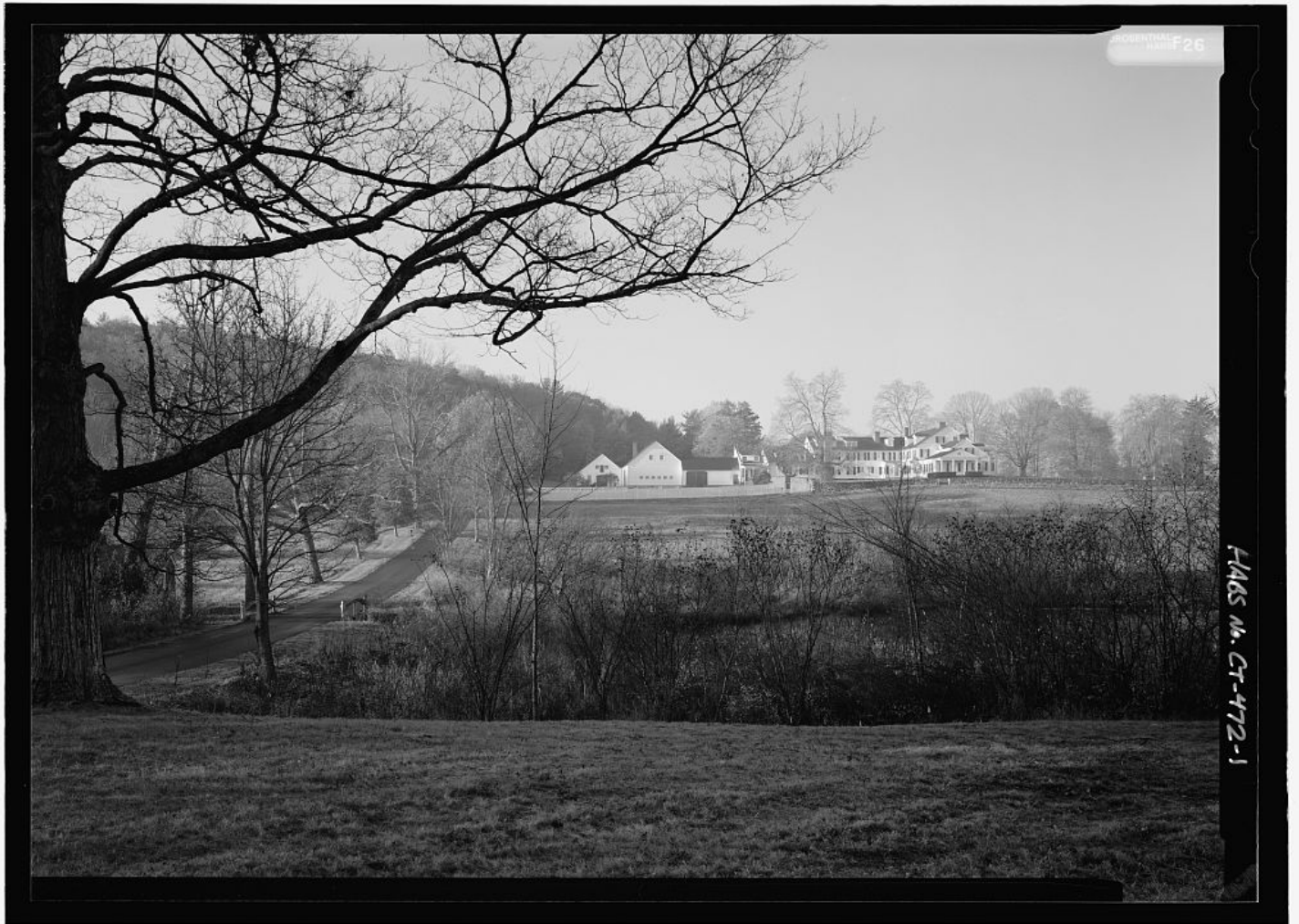
Photo 1. General View of Hill-Stead (Pope-Riddle House)—complex and landscape from east/northeast. HABS CT-472-1, 2006.
