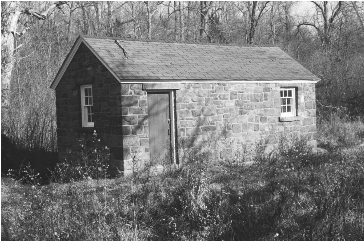
Photo 13. Pump House, looking northwest. Photograph by Peter Aaslestad, September 2017.
