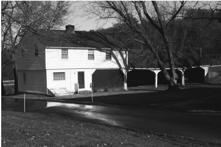
Photo 9. Shepard's Cottage, looking southwest. Photograph by Hill-Stead staff, 2011.
