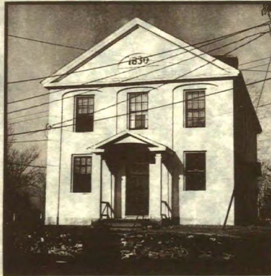
Brick School House 1830
