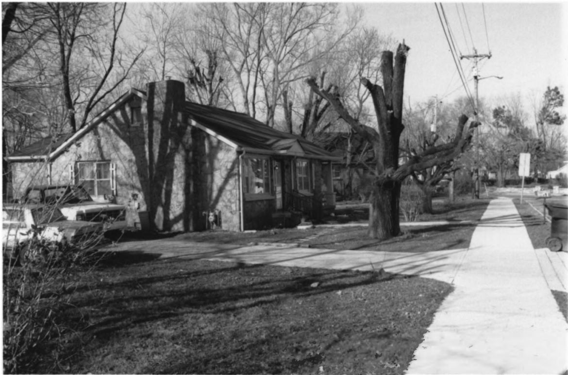
NATCHEZ STREET HISTORIC DISTRICT WILLIAMSON COUNTY, TN
