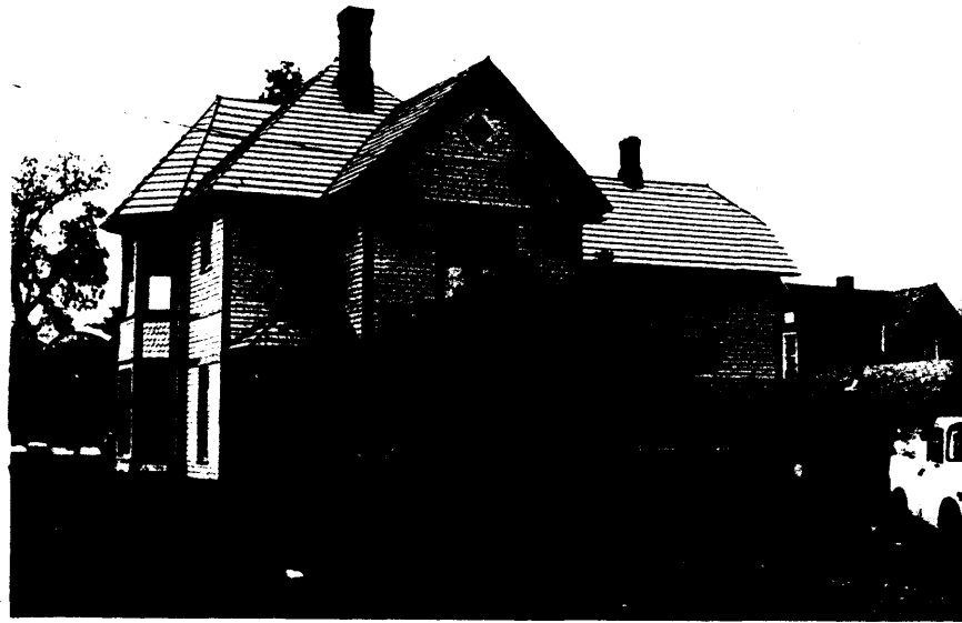
Allison-Reinkeh House; east elevation, 1987 photograph.
