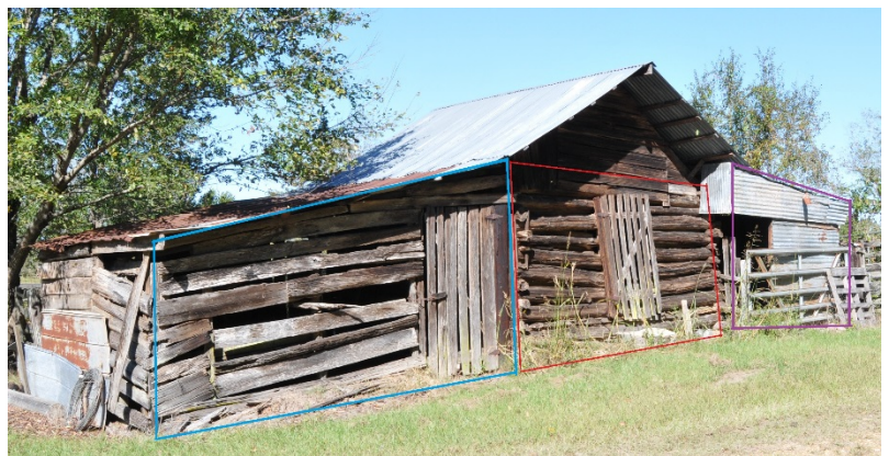
Figure 1. Red outline is the original one room structure. Blue is the 2 nd addition, purple is the 3 rd addition.
