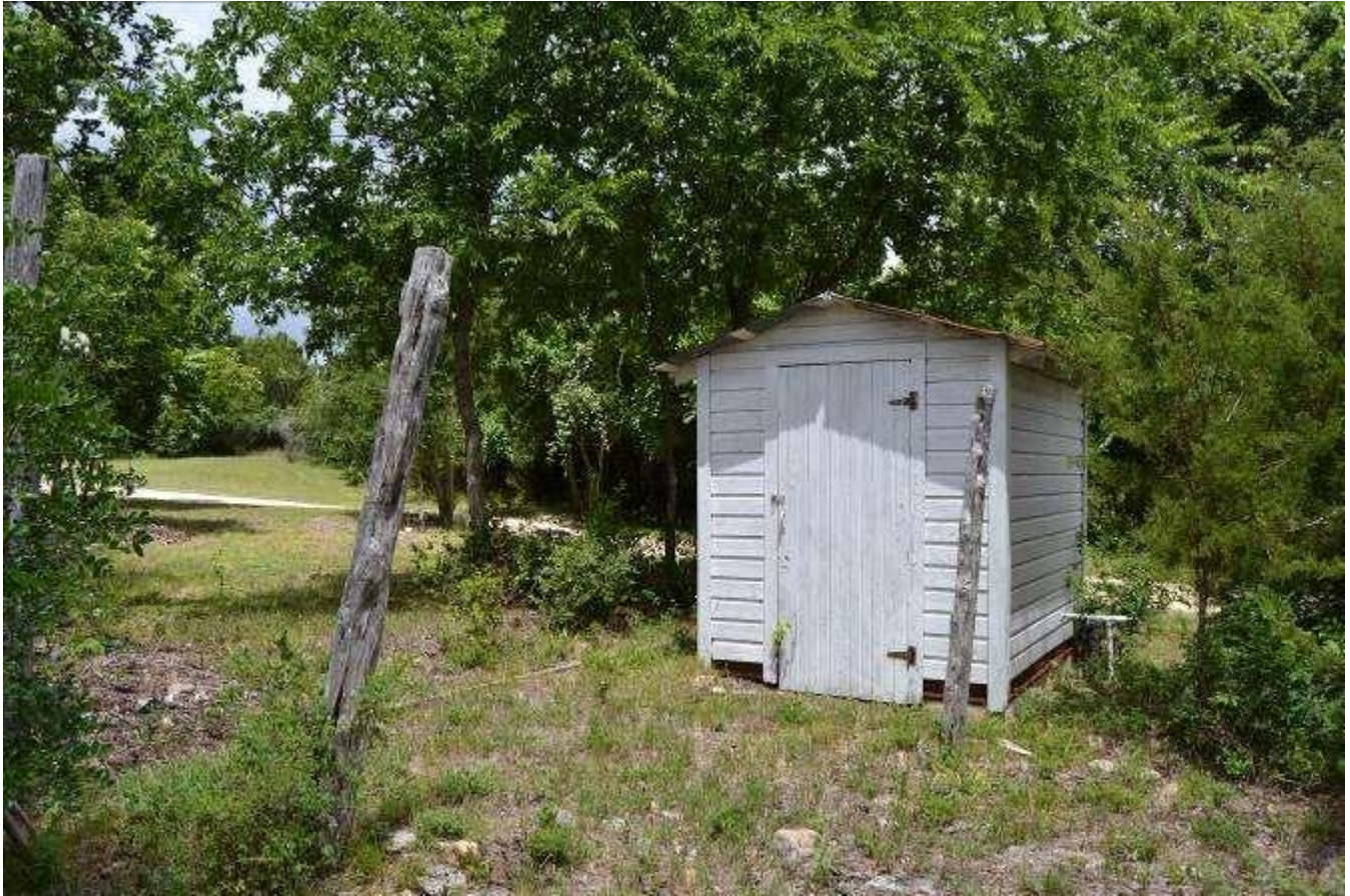
Photo No. 31. View of well house (Resource F). View facing northwest.
