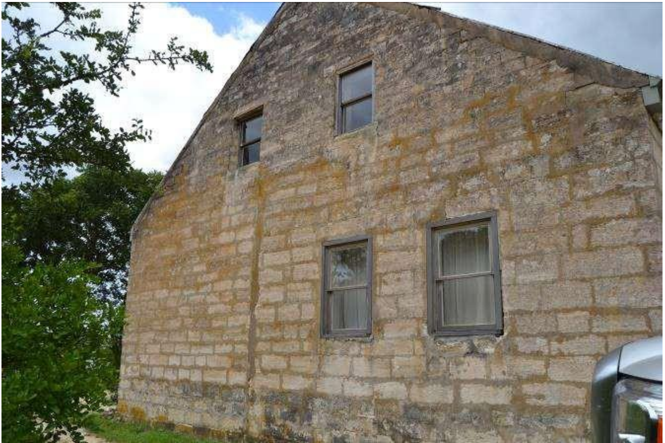
Photo No. 10. View of side northeast façade (Resource A). Note joint separating oldest portion of the house from room to the southeast. View facing south.
