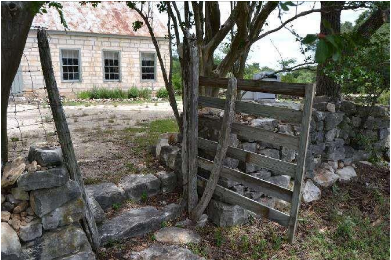
Photo No. 2. View of fencing separating house (Resource A) from former garden and grazing area to the south. View facing north.
