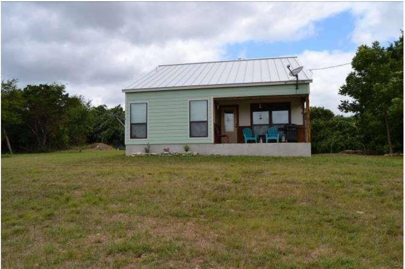
Photo No. 32. View of new house (Resource I). View facing northwest.
