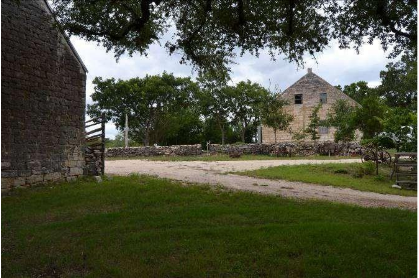
Photo No. 3. View of stone fencing separating house (Resource A) and barn (Resource B). View facing southwest.
