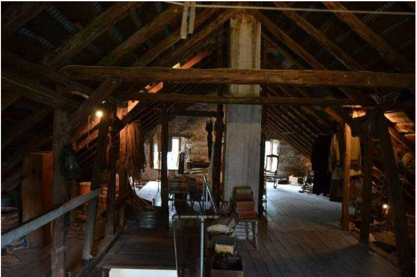
Photo No. 21. Interior view of attic (Resource A). View facing southwest.
