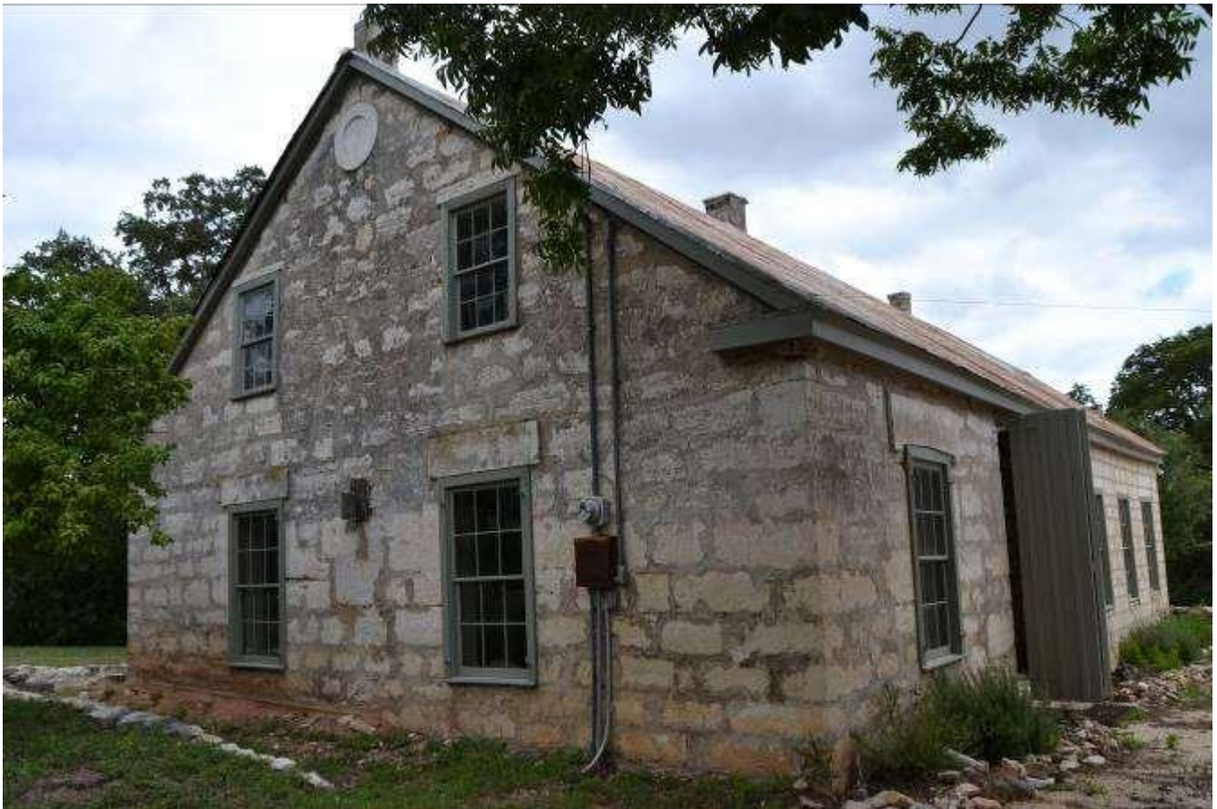
Photo No. 14. Side southwest façade (Resource A). View facing north.
