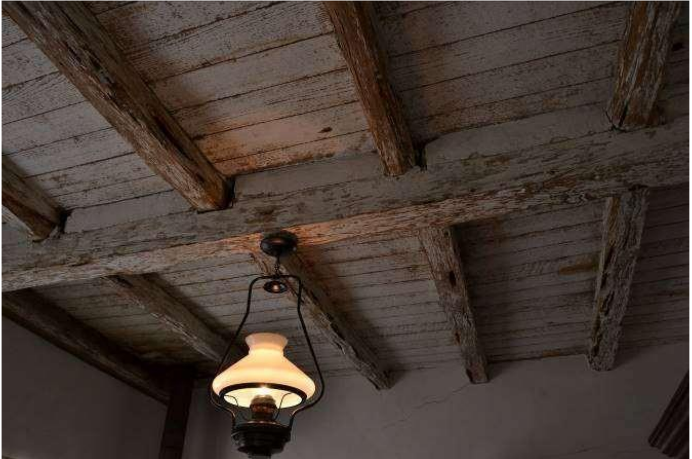
Photo No. 19. Interior view of ceiling and "summer beam" in Room 2 (Resource A). View facing south.
