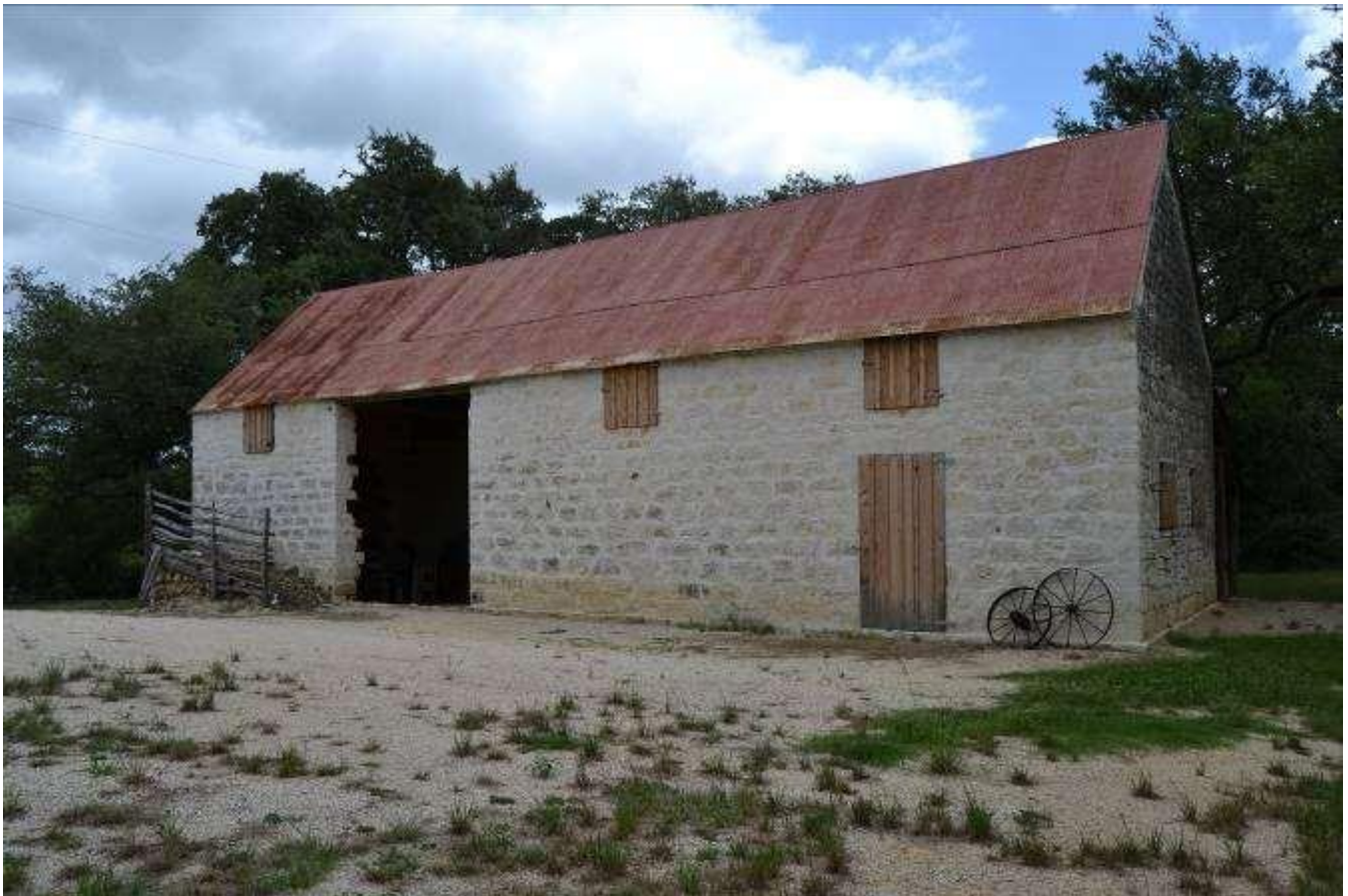
Photo No. 23. Oblique view of main west façade of barn (Resource B). View facing northeast.
