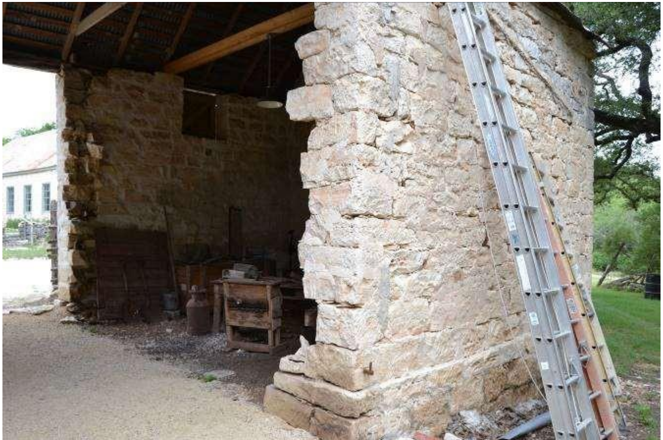
Photo No. 26. Interior view of barn (Resource B). View facing southwest.
