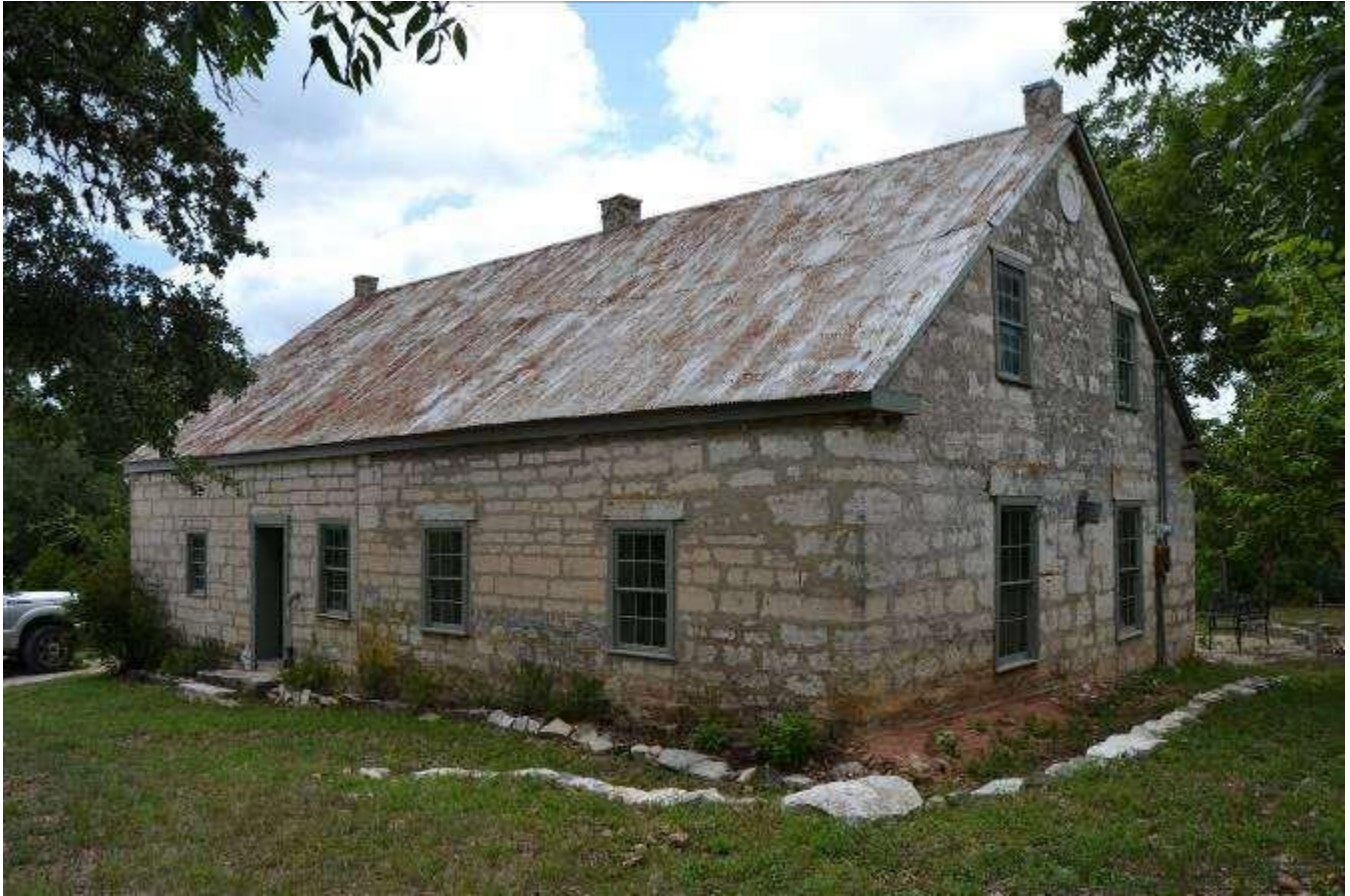
Photo No. 13. Rear northwest façade (Resource A). View facing southeast.
