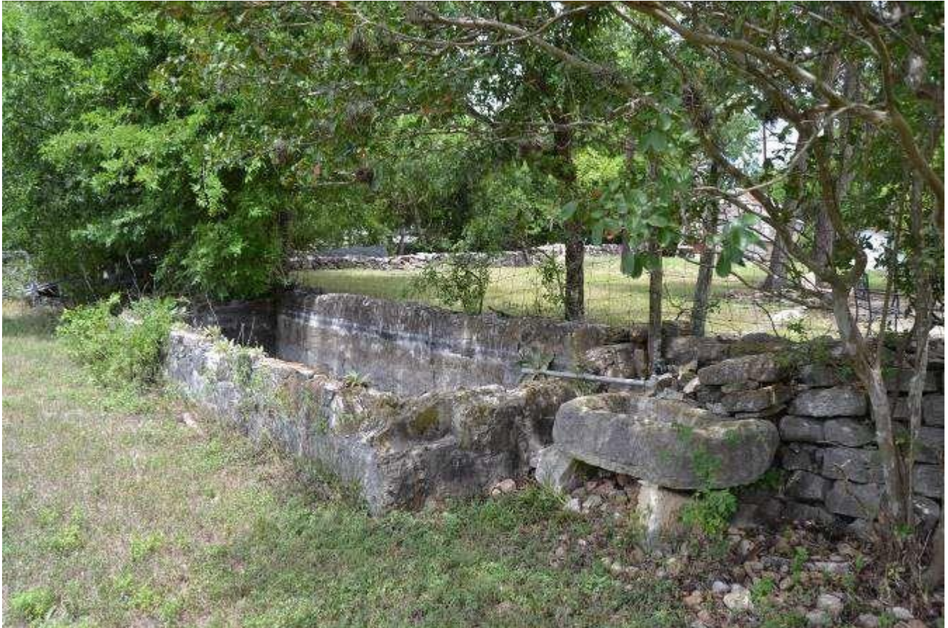
Photo No. 5. View of troughs (Resources H and J) along stone fencing. View facing west.
