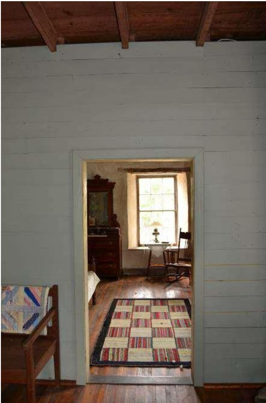
Photo No. 17. Interior view from Room 4, looking southeast into Room 5 (Resource A).
