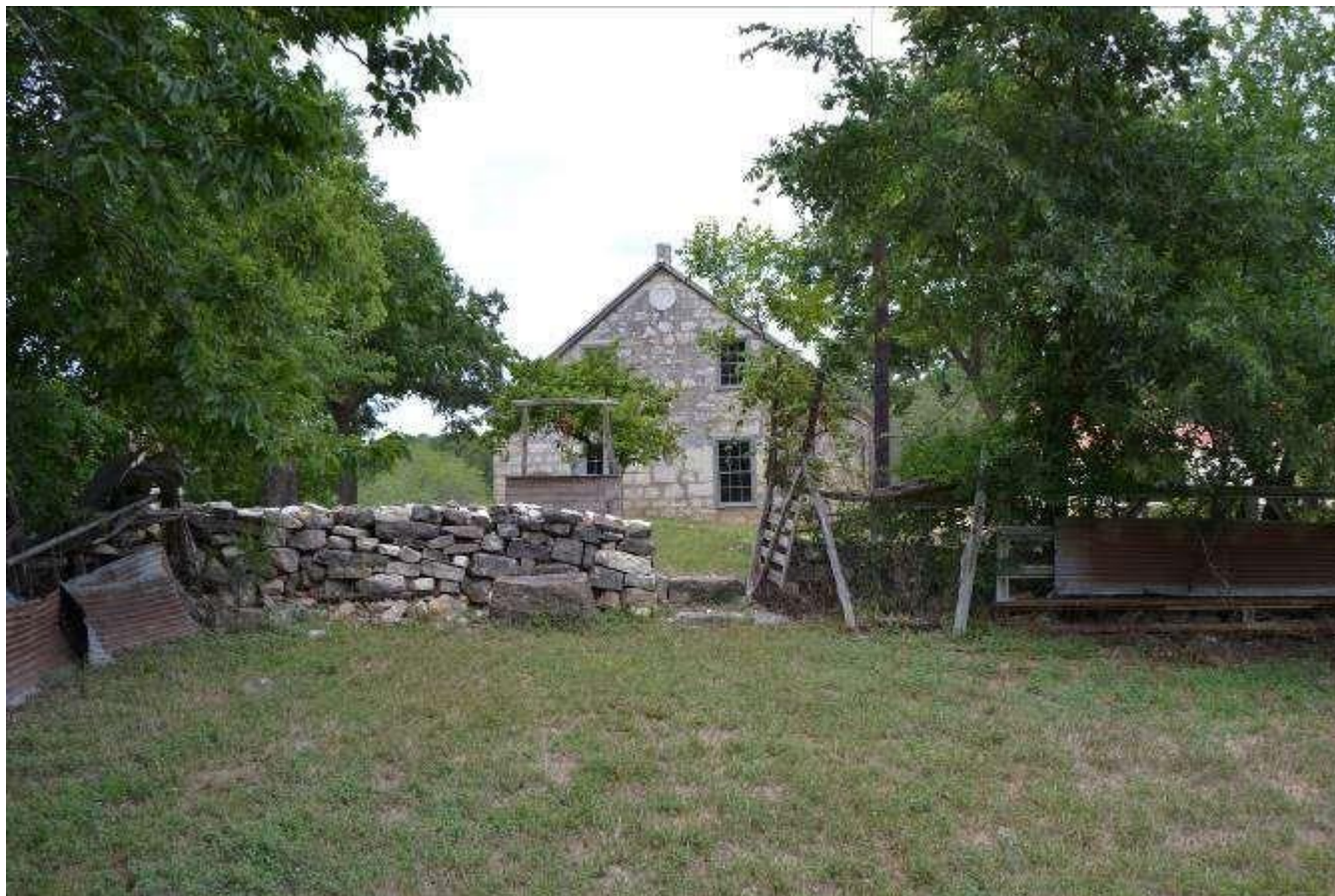
Photo No. 4. View of stone and wood post fencing separating house and former pen area. View facing northeast.
