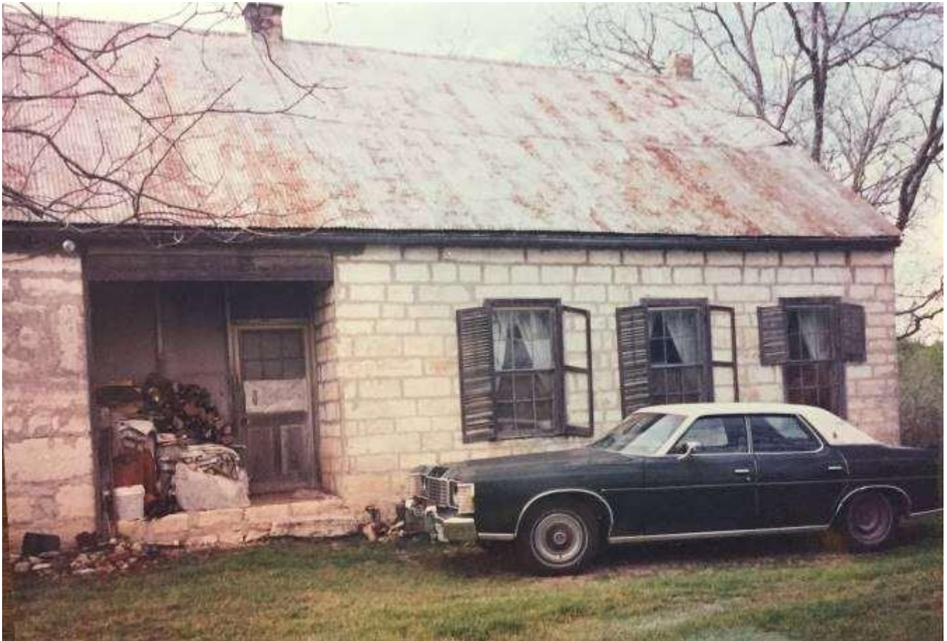
Figure 2. Historic photograph (undated) of Arnold-Rauch-Brandt house (Resource A) before inset porch was enclosed. Source: New Braunfels Conservation Society.
