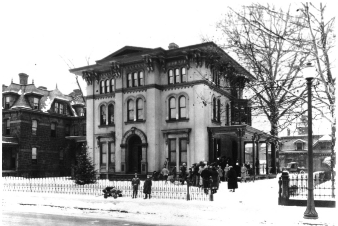
N.G., MERCER CO., CHARLES BREARLEY HOUSE, ATTACHMENT #6
