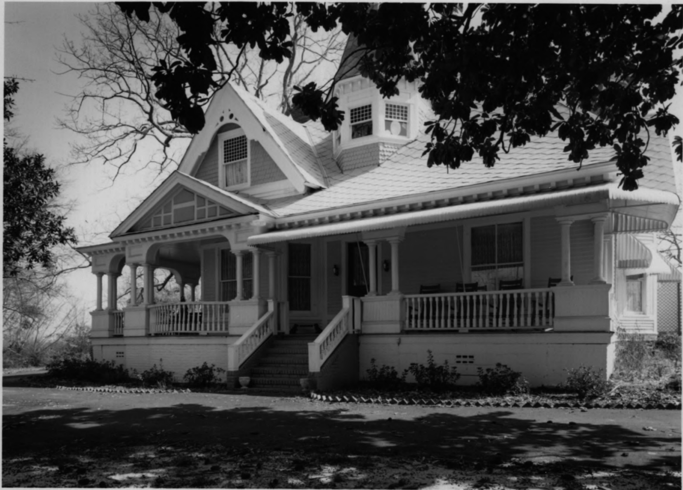
BENJAMIN F. BULLOCH HOUSE MERWETHER COUNTY, GEORGIA WARM SPRINGS, GA
