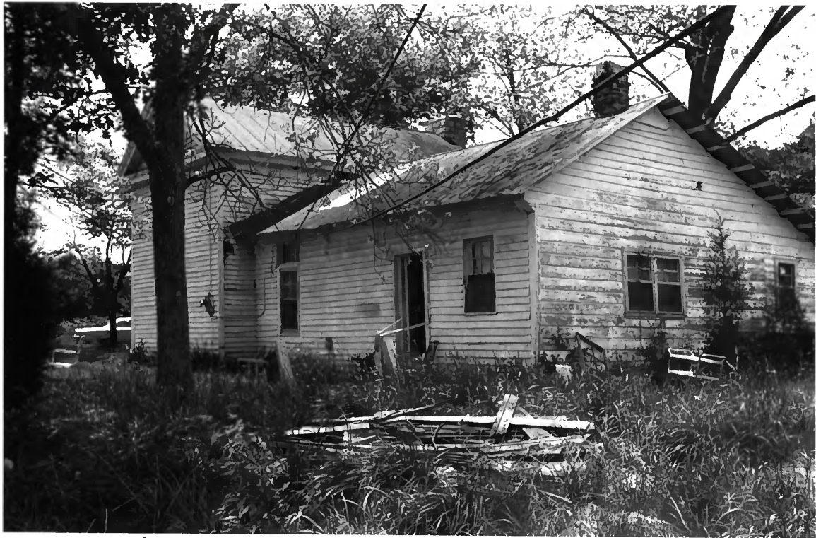
Derryberry House Spring Hill vicinity, Maury Co., TN
