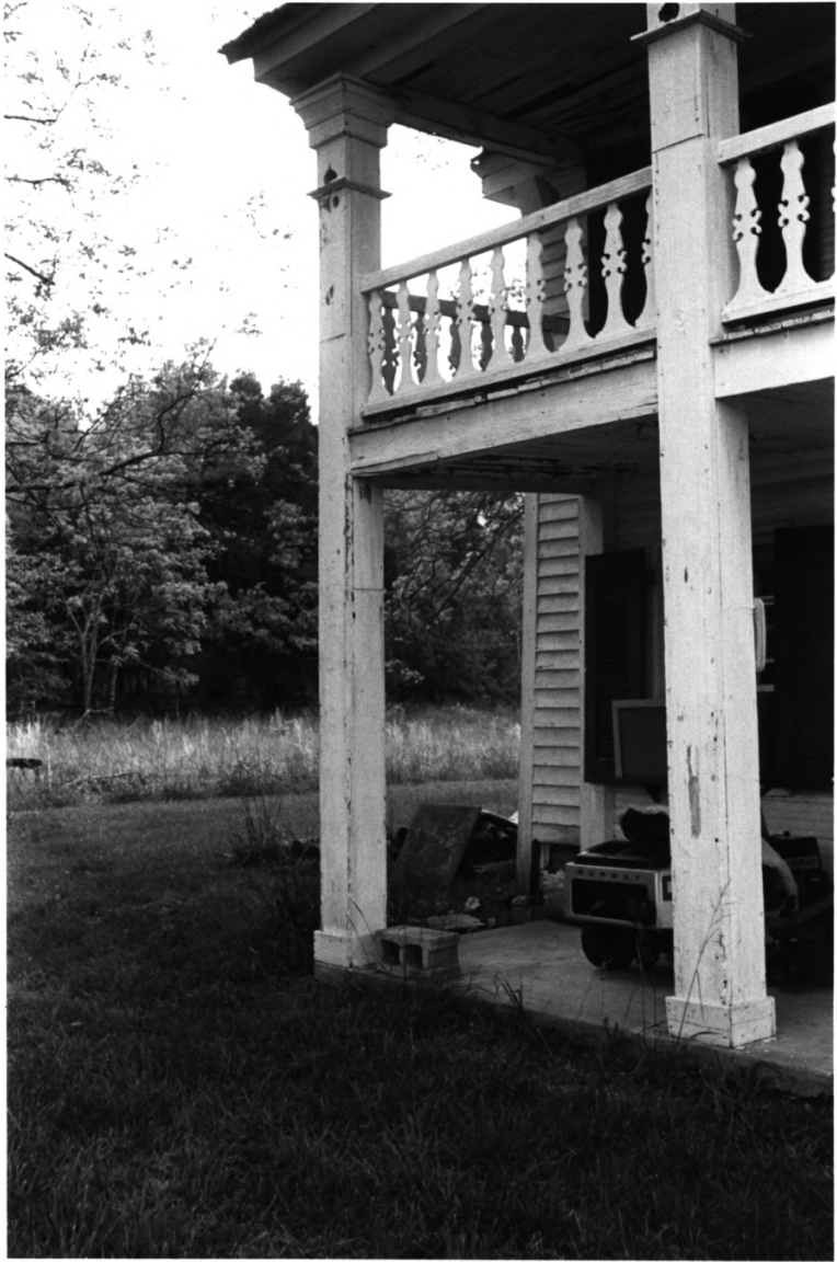
Derryberry House Spring Hill vicinity, Maury Co., TN
