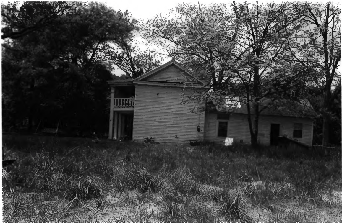
Derryberry House Spring Hill vicinity, Maury Co., TN
