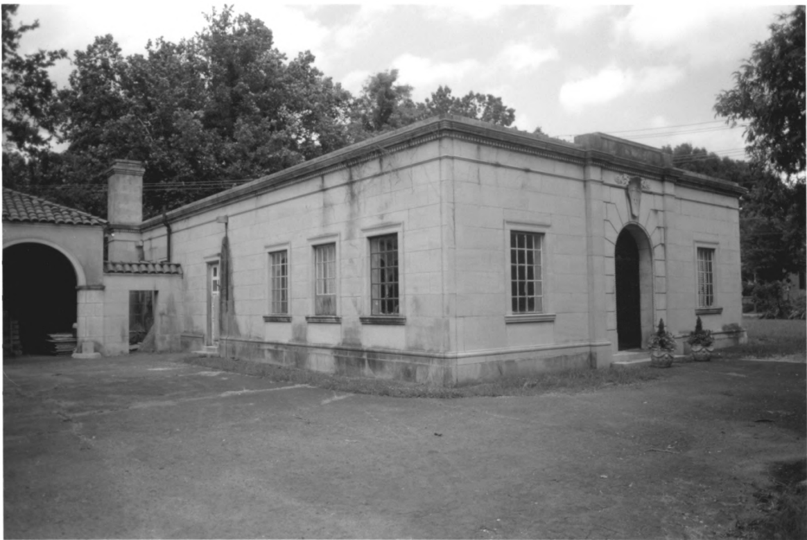
CANDORO MARBLE COMPANY SHOWROOM & GARAGE KNOX COUNTY TN 10 OF 24
