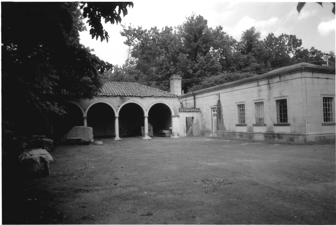
CANDORO MARBLE COMPANY SHOWROOM & GARAGE KNOX COUNTY TN 9 OF 24
