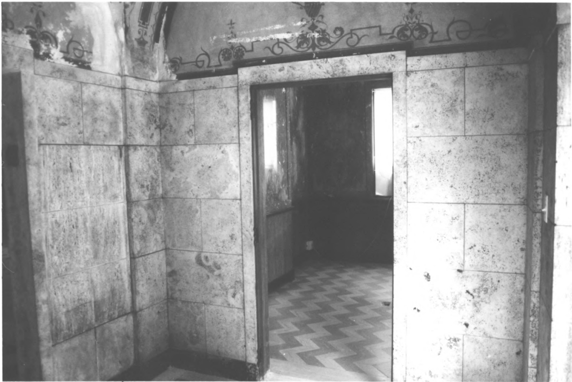
CANDORO MARBLE COMPANY SHOWROOM & GARAGE KNOX COUNTY TN 23 OF 24
