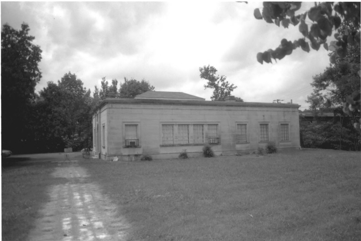
CANDORO MARBLE COMPANY SHOWROOM & GARAGE KNOX COUNTY TN 3 OF 29
