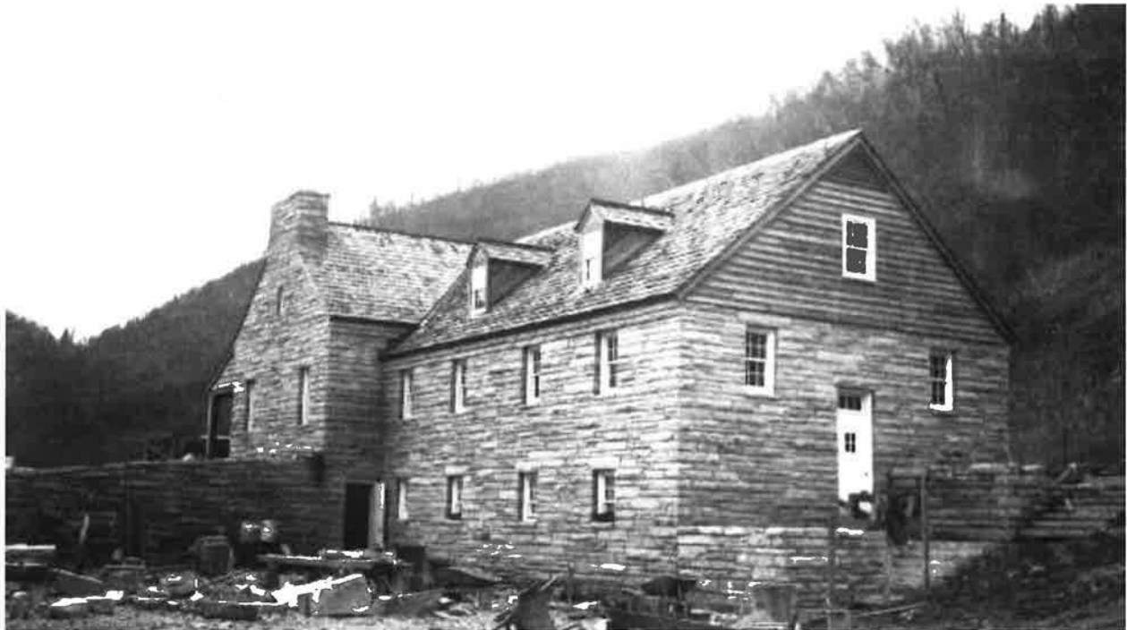
Figure 4. Photograph of Oconaluftee Ranger Station during construction, rear and east side, n.d. Neg. No. 1491 (source: Great Smoky Mountains NP, Gatlinburg, TN).
