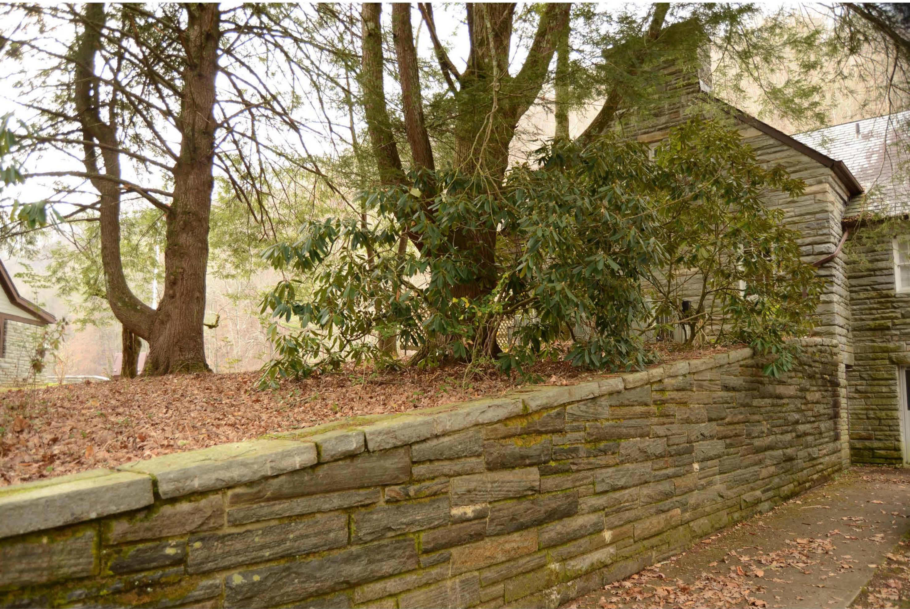
Oconaluftee Ranger Station Swain County, North Carolina Photo 6 of 13
