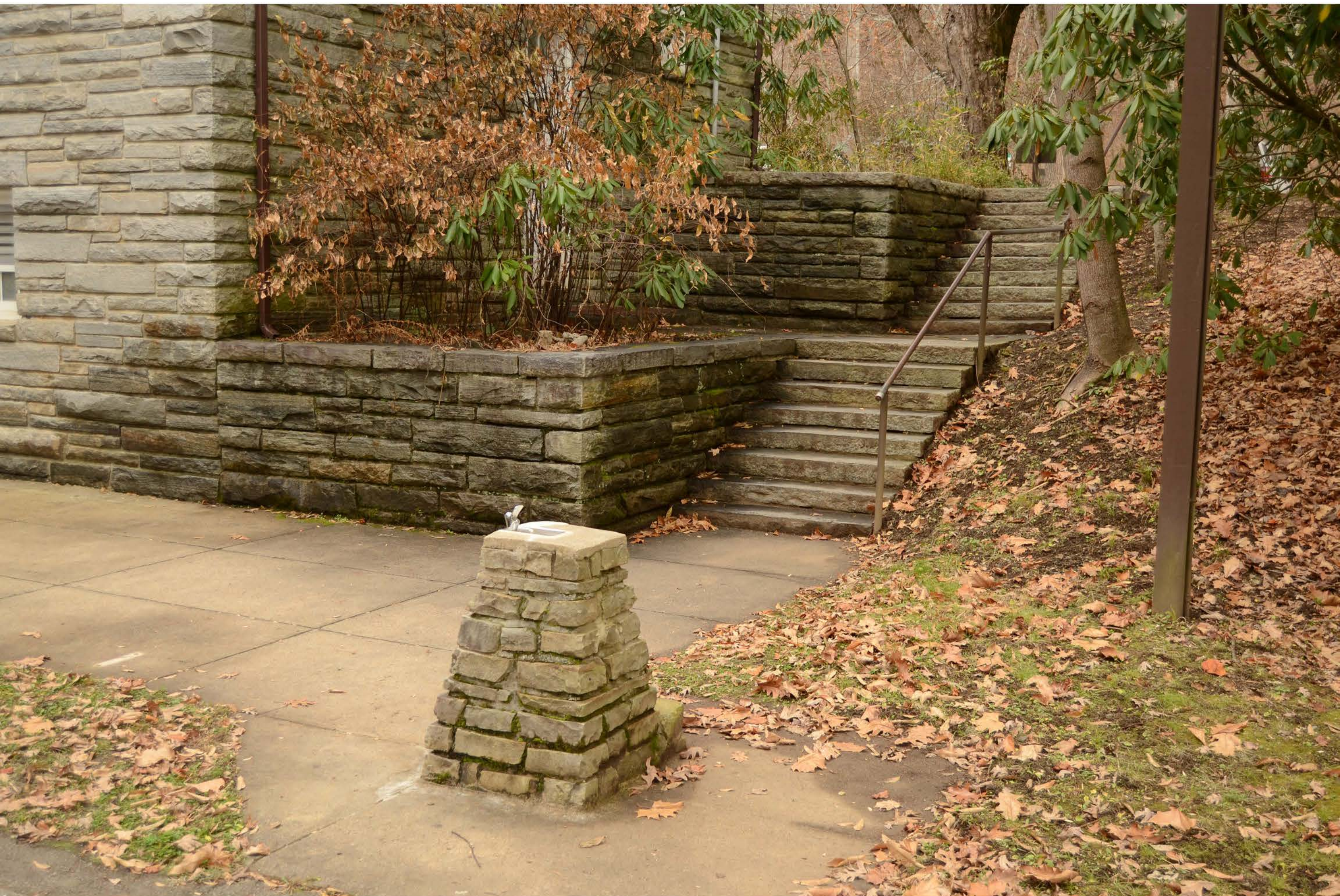
Oconaluftee Ranger Station Swain County, North Carolina Photo 7 of 13
