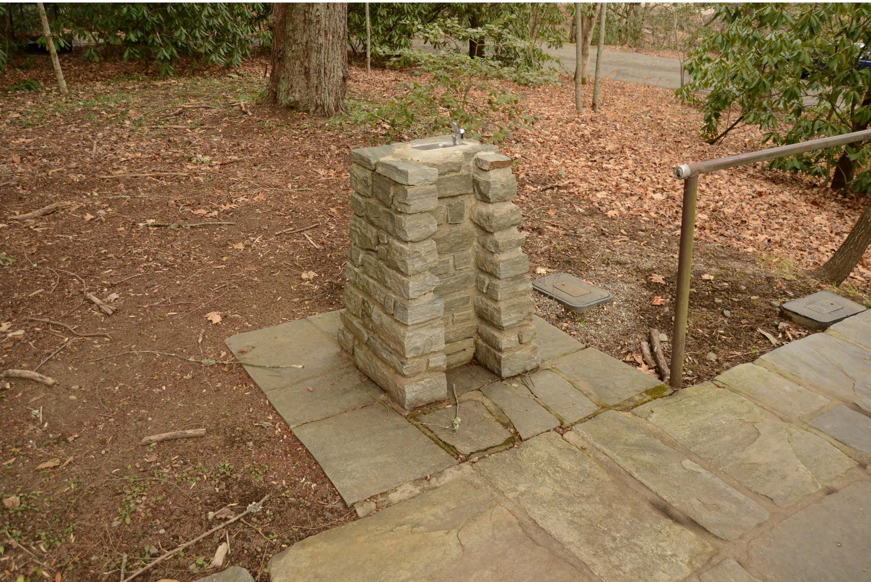
Oconaluftee Ranger Station Swain County, North Carolina Photo 8 of 13
