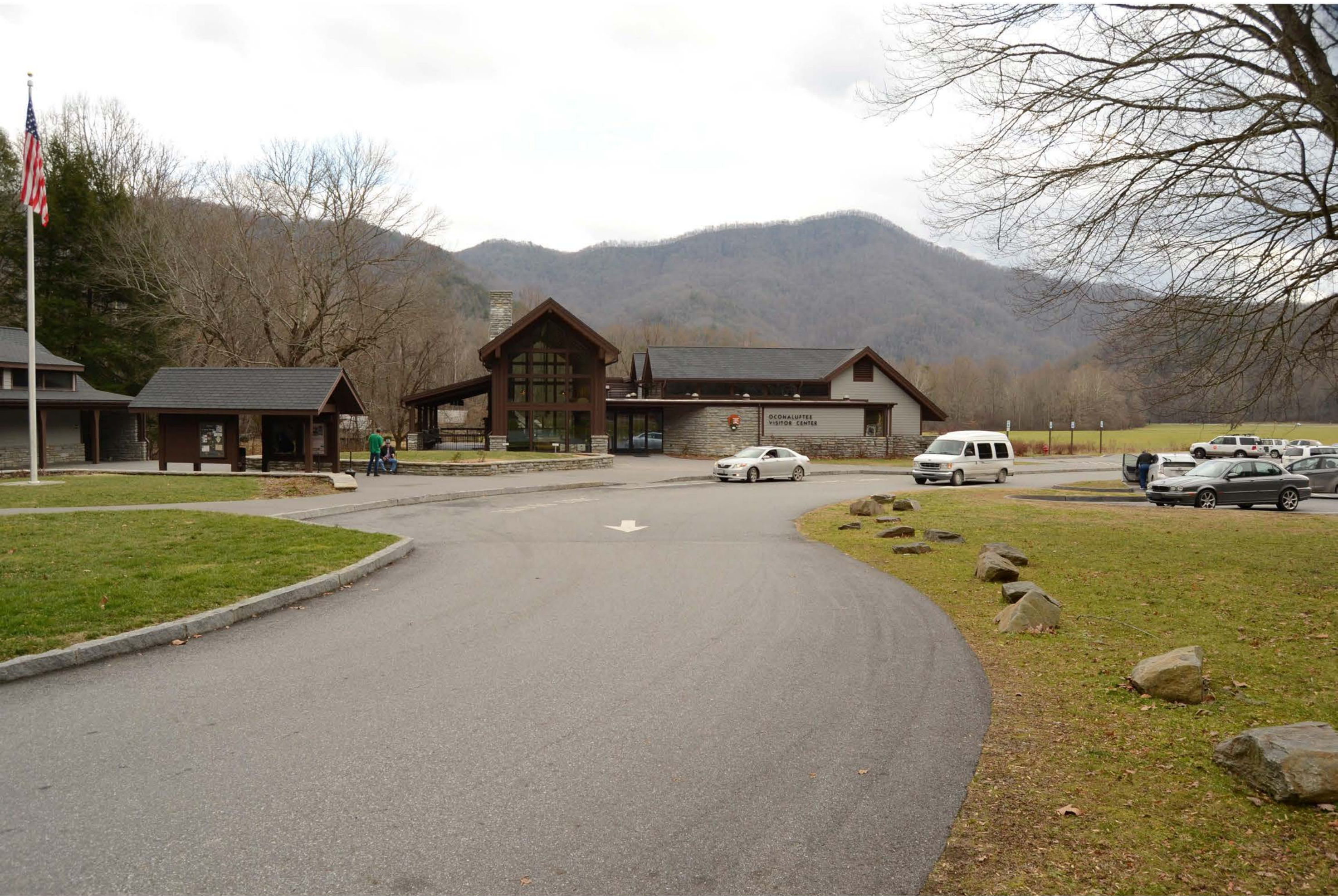
Oconaluftee Ranger Station Swain County, North Carolina Photo 10 of 13
