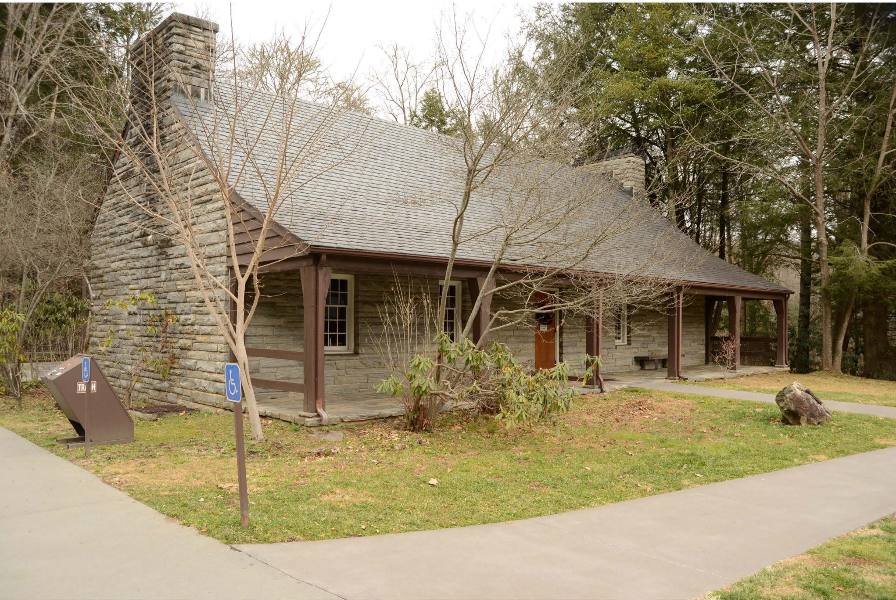
Oconaluftee Ranger Station Swain County, North Carolina Photo 1 of 13
