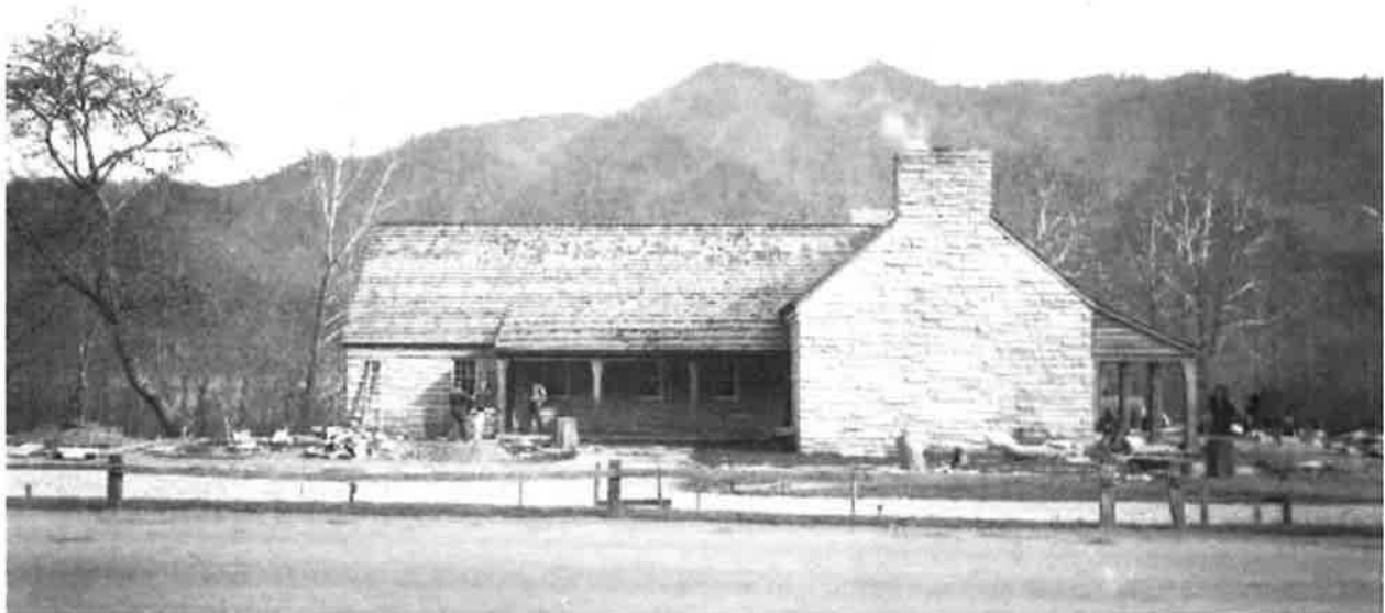
Figure 5. Photograph of Oconaluftee Ranger Station during construction, west side, n.d. Neg. No. 1490 (source: Great Smoky Mountains NP, Gatlinburg, TN).
