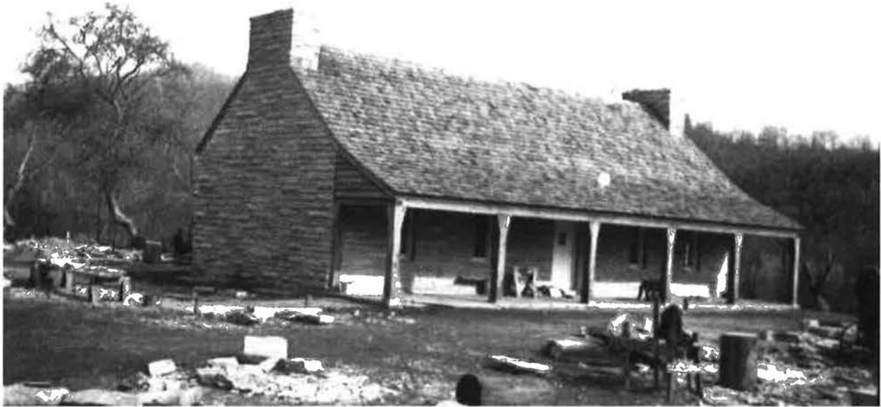
Figure 2. Photograph of Oconaluftee Ranger Station during construction, front, n.d. Neg. No. 1487 (source: Great Smoky Mountains NP, Gatlinburg, TN).
