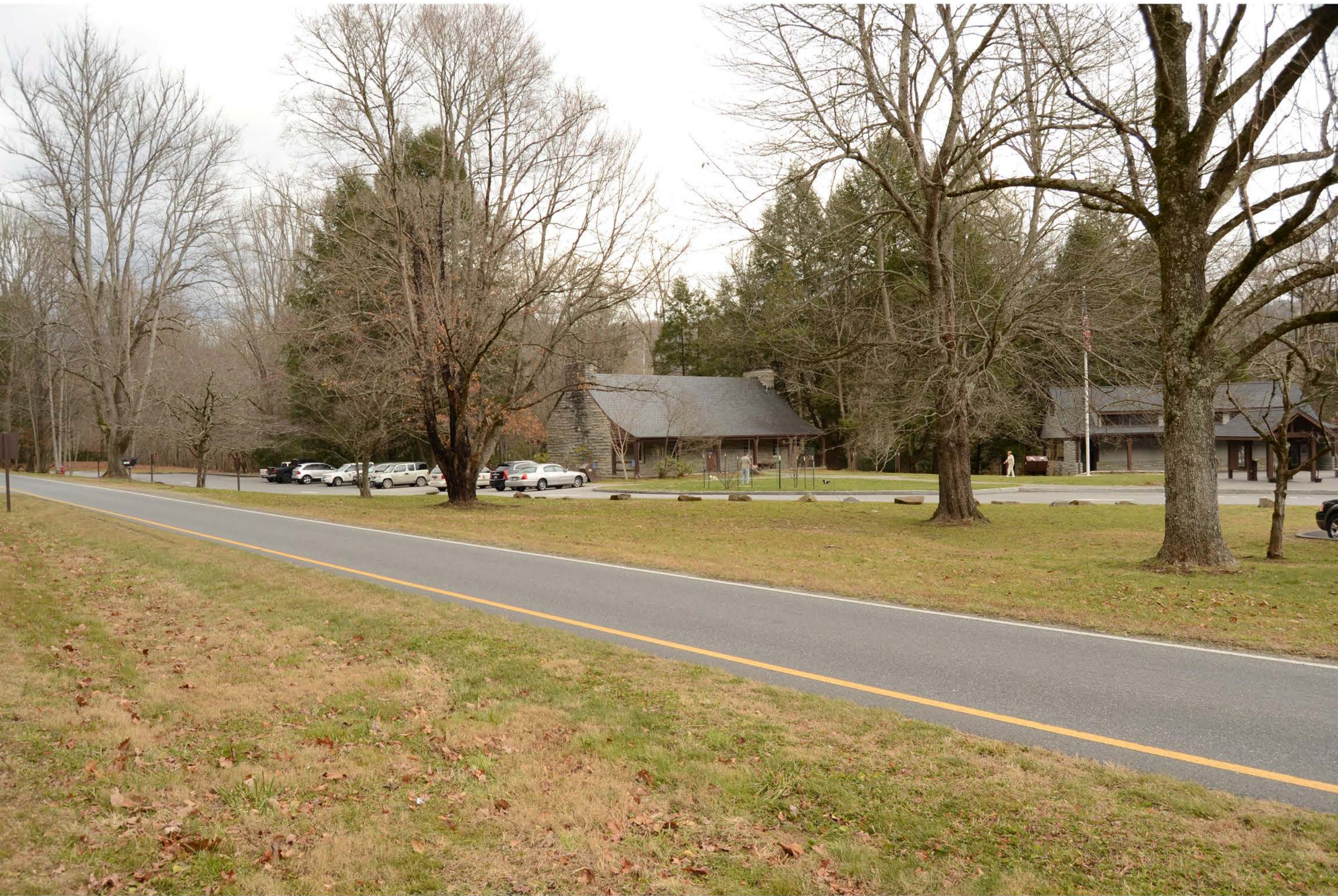
Oconaluftee Ranger Station Swain County, North Carolina Photo 9 of 13
