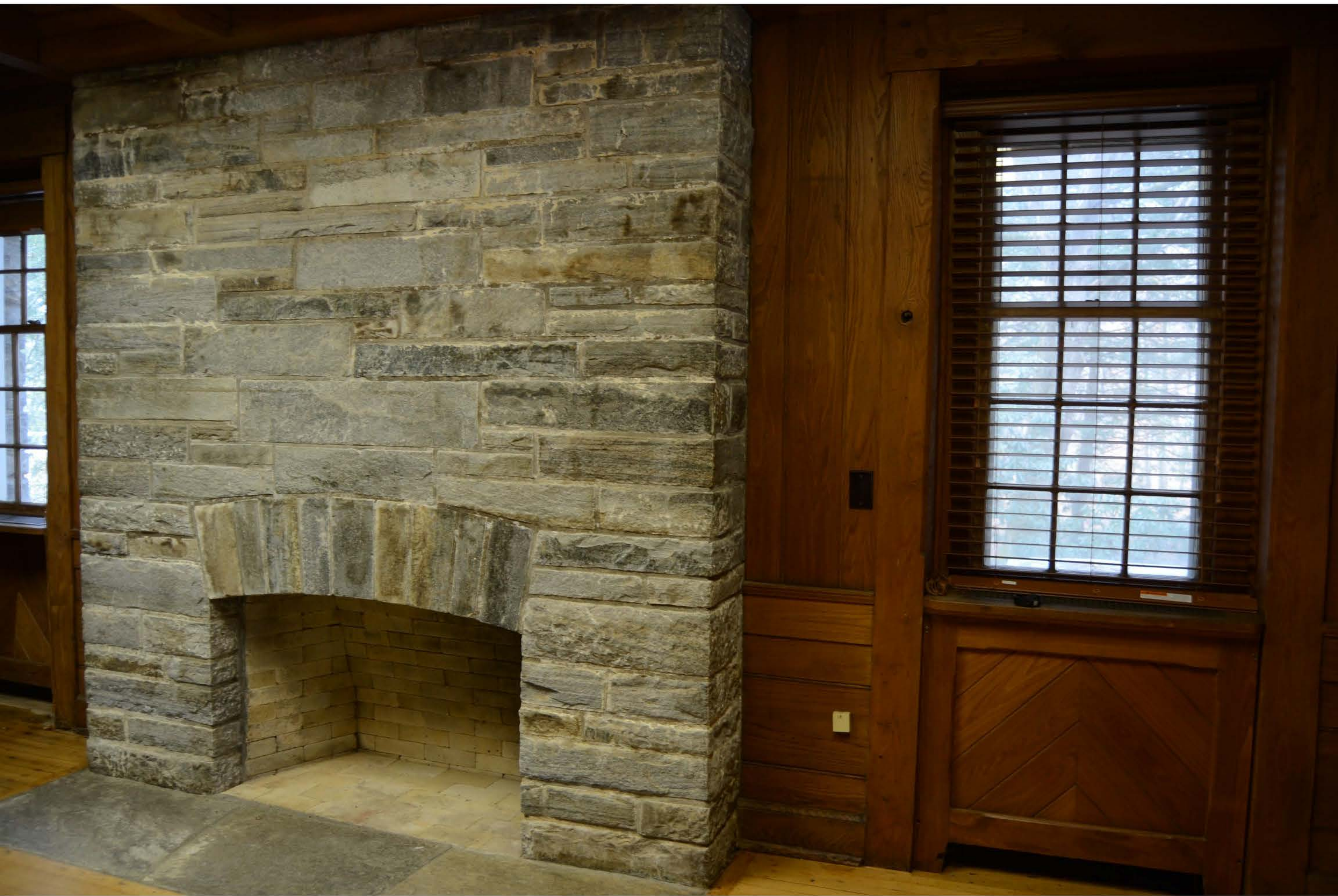
Oconaluftee Ranger Station Swain County, North Carolina Photo 13 of 13
