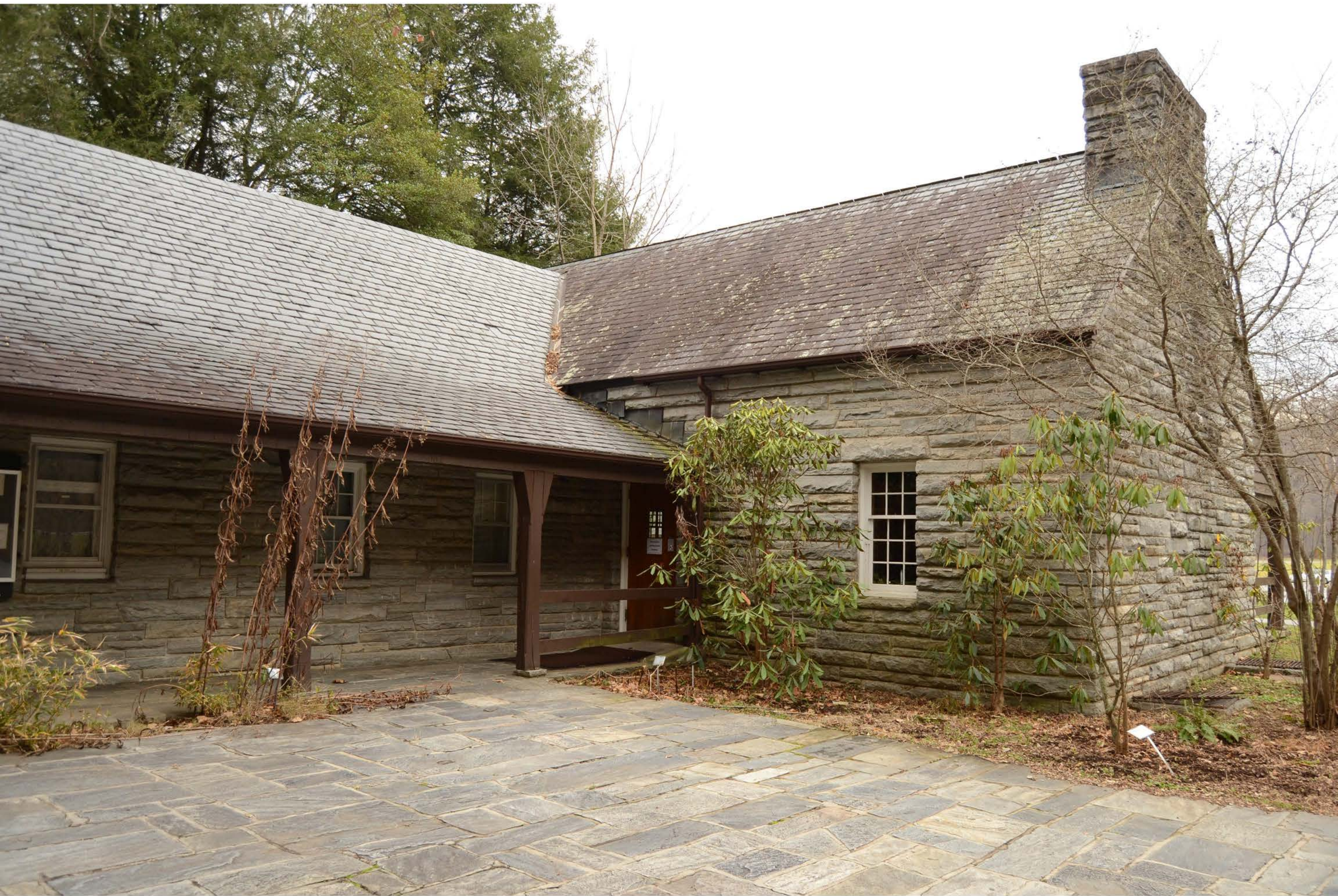
Oconaluftee Ranger Station Swain County, North Carolina Photo 2 of 13
