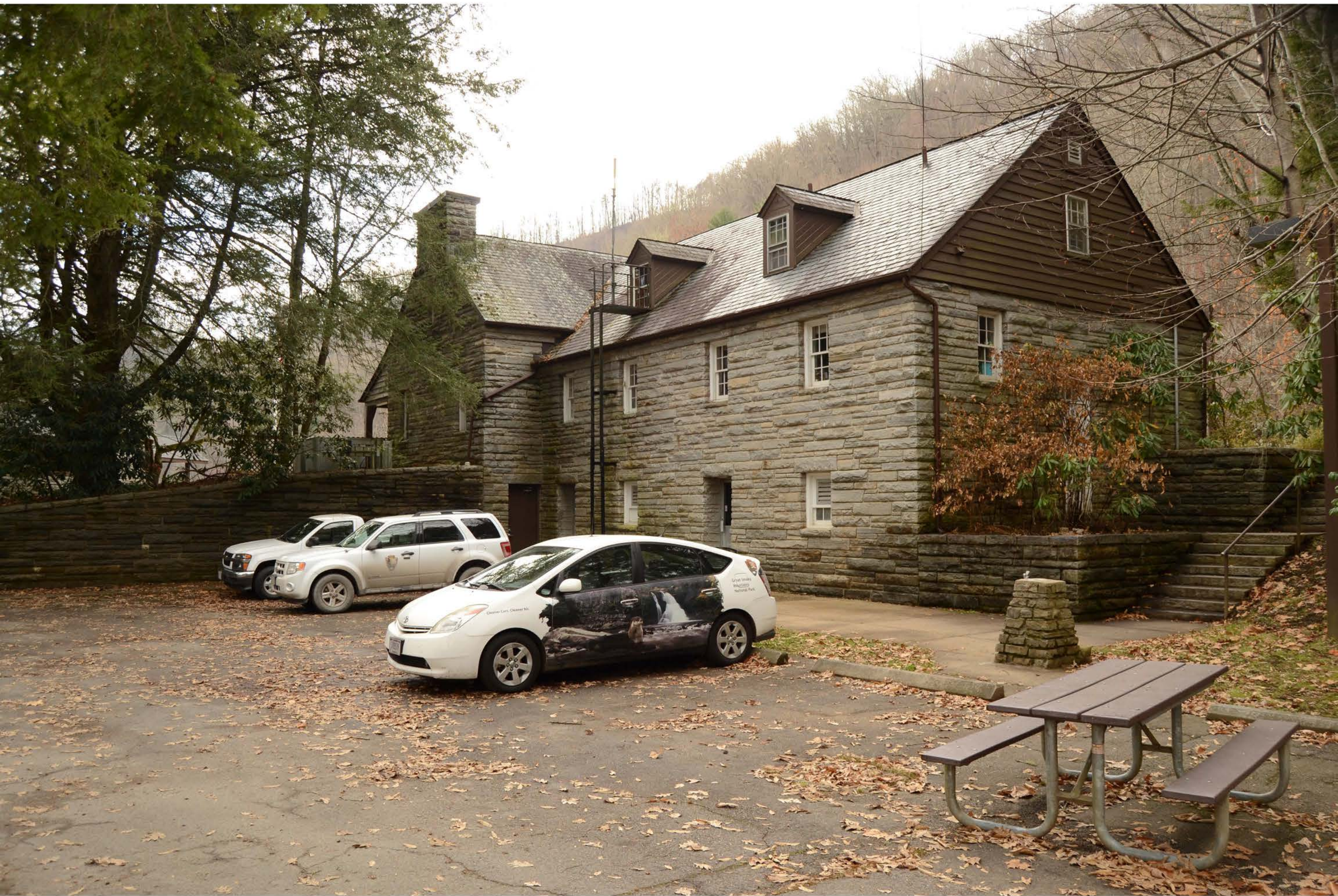
Oconaluftee Ranger Station Swain County, North Carolina Photo 4 of 13
