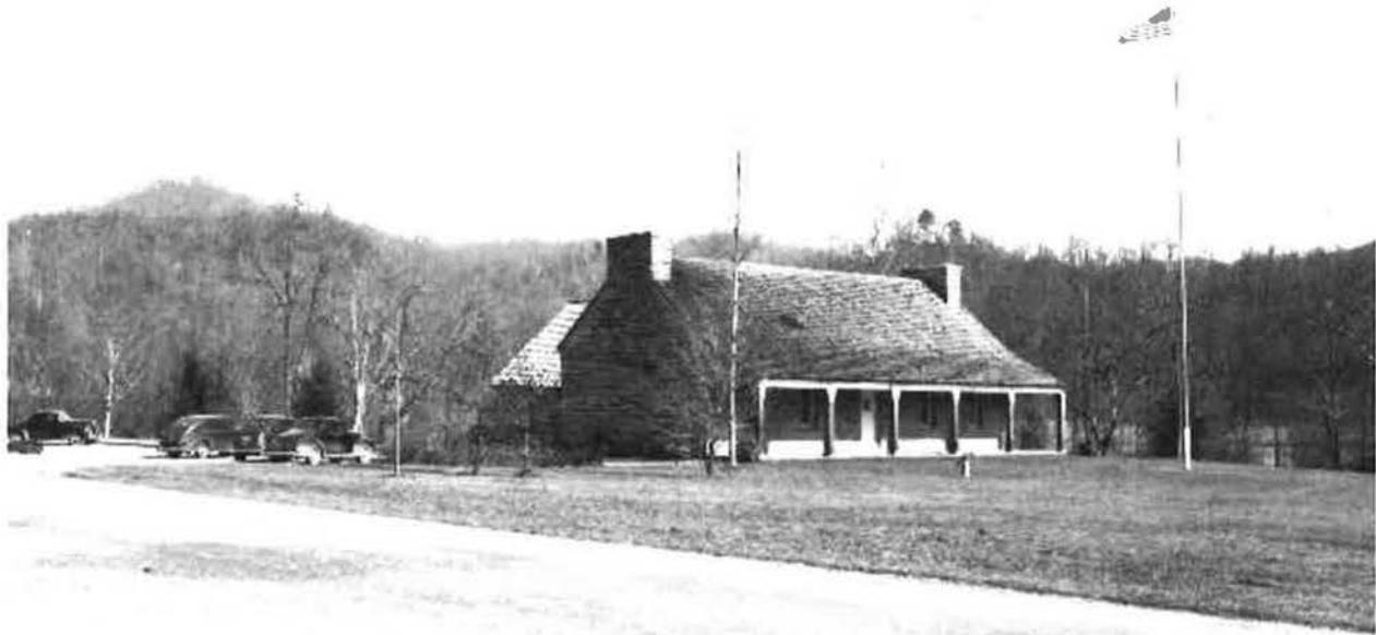
Figure 6. Photograph of Oconaluftee Ranger Station, front, n.d. Neg. No. 1474 (source: Great Smoky Mountains NP, Gatlinburg, TN).
