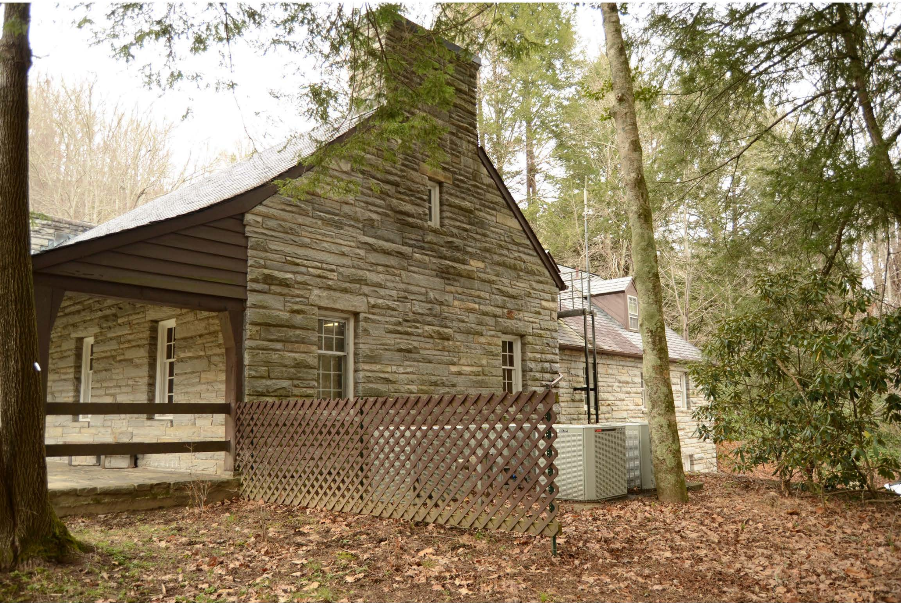
Oconaluftee Ranger Station Swain County, North Carolina Photo 5 of 13
