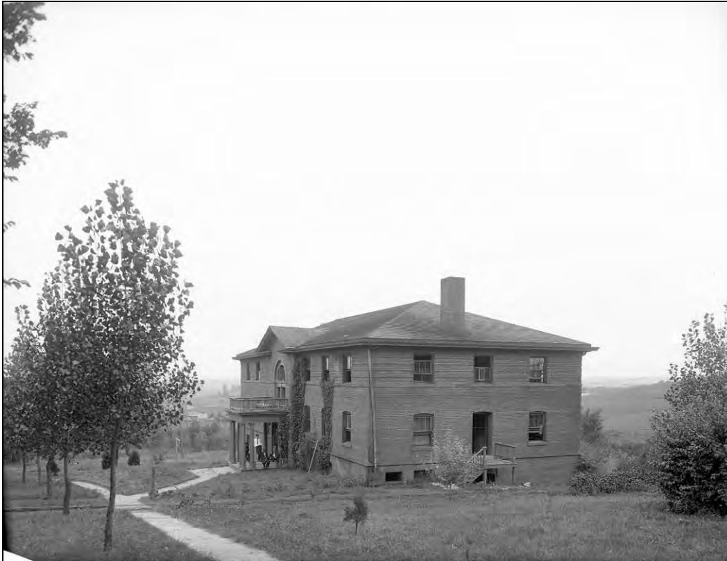
Figure 29: Hamilton Hall, looking south-southwest, circa 1915. From the Durham Museum's Photography Archive.
