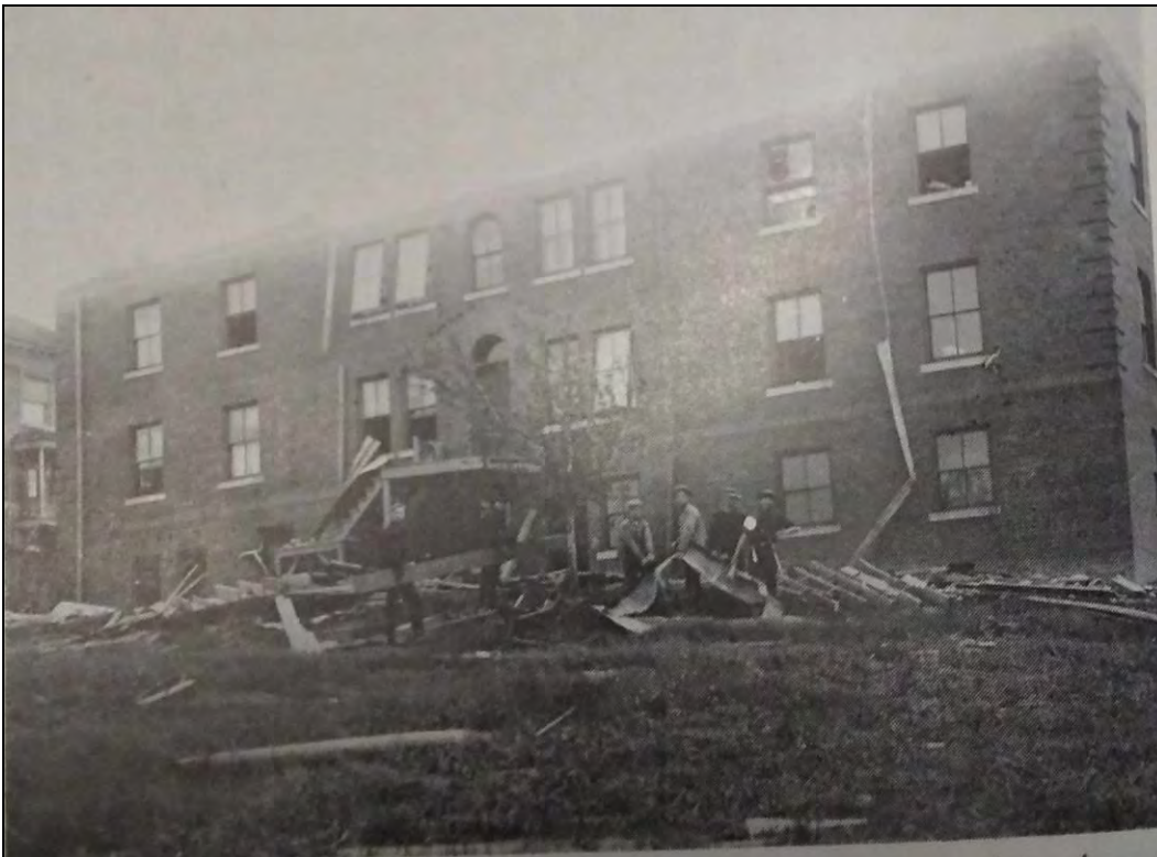
Figure 276: Tornado damage along the rear of Lowrie Hall, 1908. Note the central arched door in the center, and the arched window above it. From Creigh, 1963.
