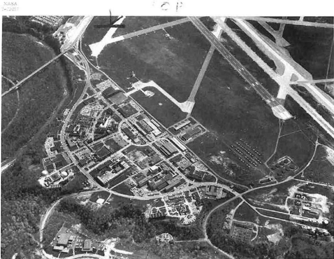
FIGURE 2 – NASA Lewis Research Center, 1964, aerial view looking northeast; National Aeronautics and Space Administration (NASA), Photo C-69627, Cleveland Public Library, Picture Collection: NASA. The Development Engineering Building & Annex are located in the upper left corner of the photo.
