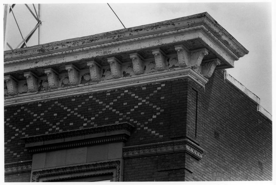
Detail of bracketted cornice with twisted rope above and eqq and dart moldings below brackets. Band of patterned brick work beneath cornice, window lintel with and egg and dart molding. D.C. Department of Recreation field offices 750 Park Road, N.W. Washington, D.C., 1985
