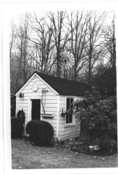
Rubble and frame accessory building and metal windmill. Looking NE. neg. file #19844-16 slide
