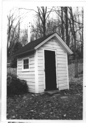
Frame accessory building Looking N. neg. file #19844-17 slide
