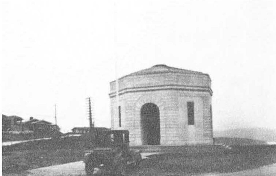
Figure 7: Memorial Hall just completed, looking northeast, circa 1924-25. Note there is no landscaping and there are four concrete steps and a base visible at the plinth. Photo from the collection of the Crockett Museum and Historical Society.
