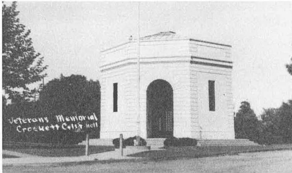
Figure 9: Postcard of Memorial Hall after the 1938 basement reconstruction and re-landscaping. Note only three concrete steps and a base are visible.
