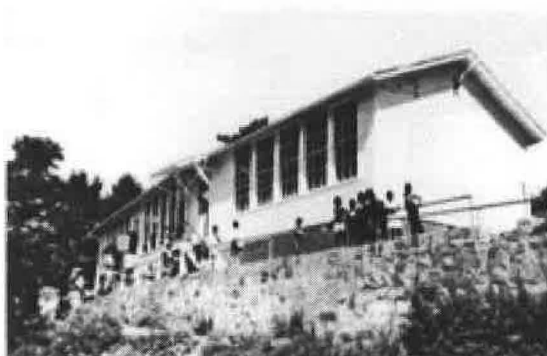
Plate 9. Switchback (Union Hurst) School, Bath County VA, late 1930s. Bath County Historical Society, Warm Springs VA. This photograph shows the added stone retaining walls and railings.
