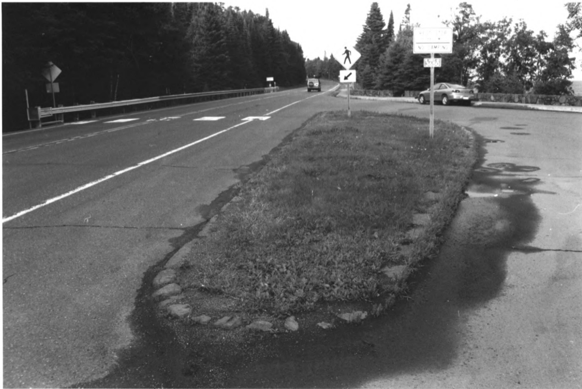
Cascade River wayside Traffic Island with stone curbing Cook Co., MN 014535-6-6
