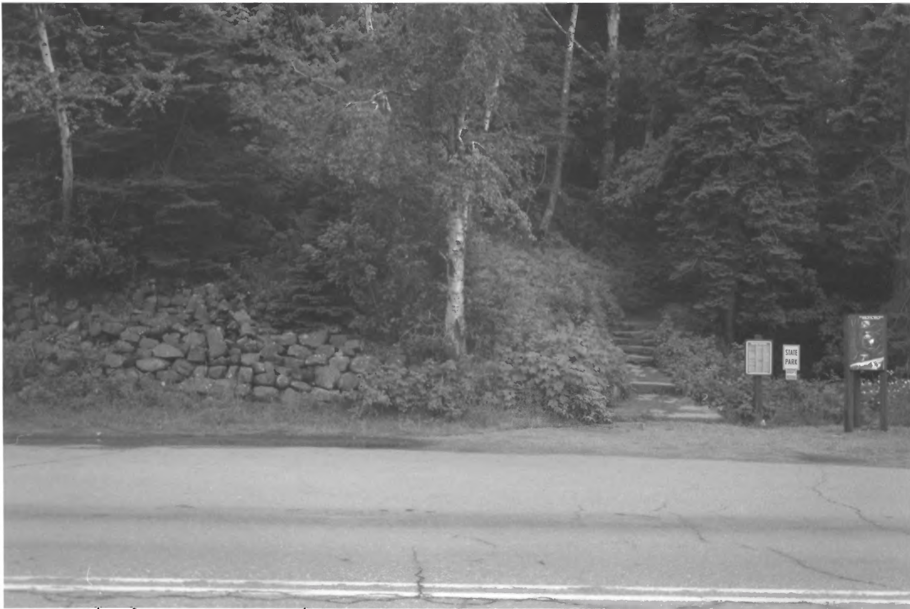
Cascade River Wayside Dry Stone Retaining Wall Cook Co., Mn 014539-14-F
