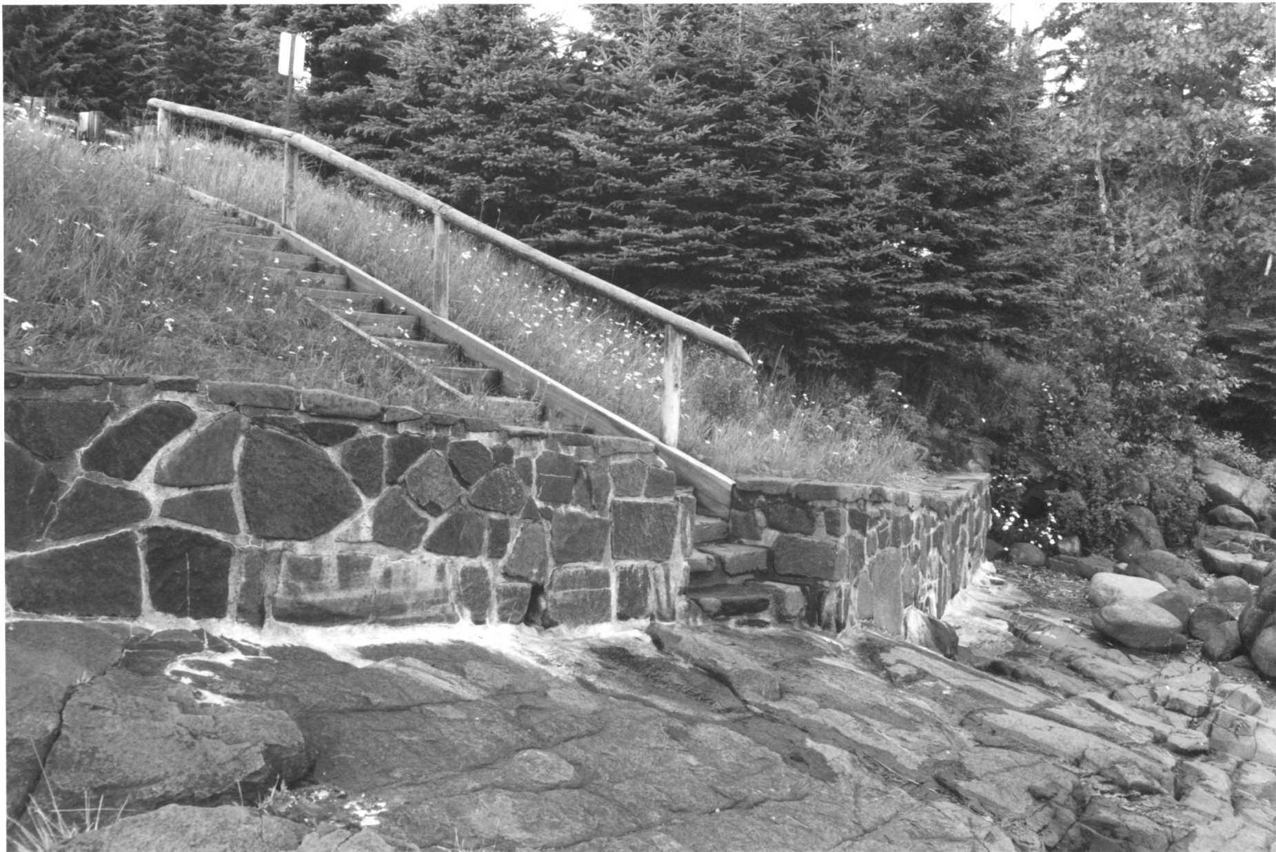
Cascade River Wayside Highway Overlook. 1981 Retaining Wall Cook Co., Mn 014535-2-5
