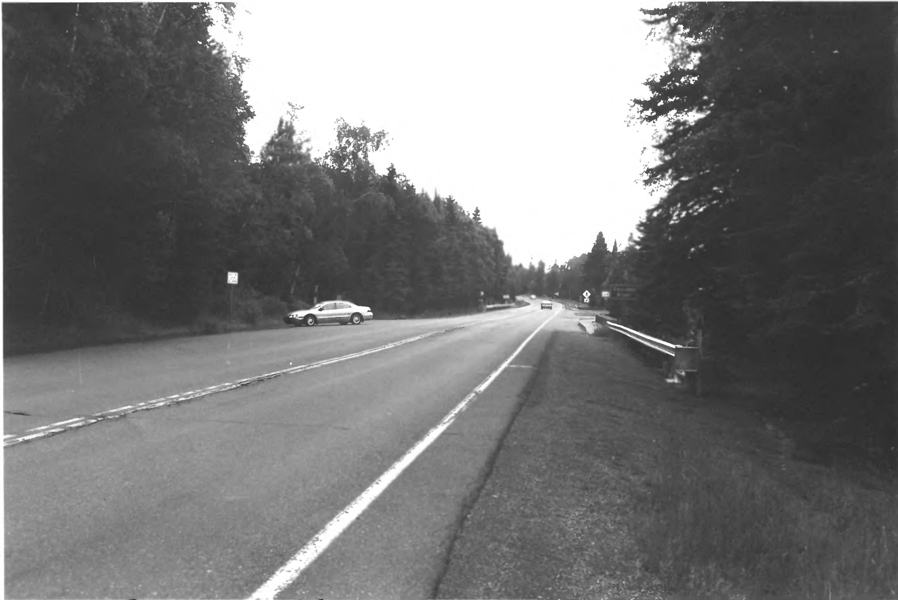
Cascade River Way side Highway 61 Within Way side Cook Co., Mn 014539-12 - 0
