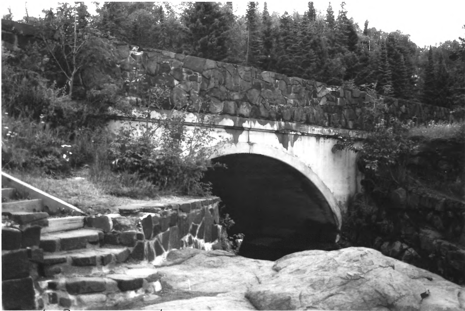
Cascade River Wayside Bridge 5132 Cook Co., Mn 014539-20 -- 5
