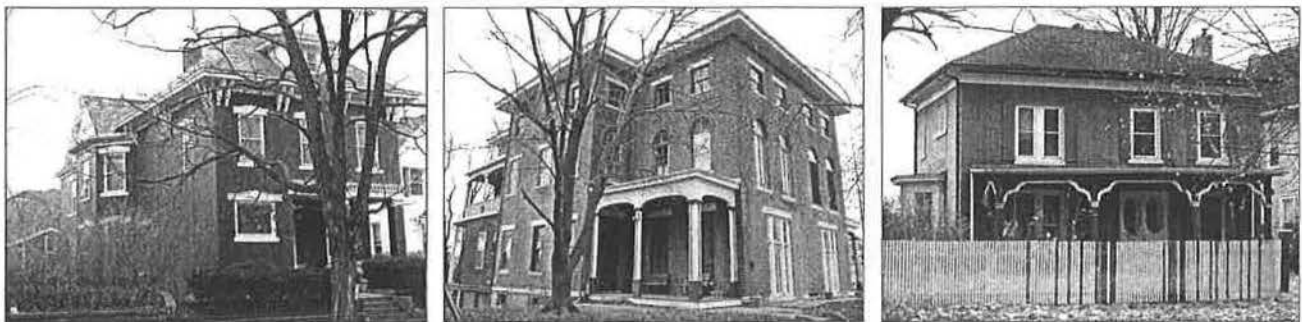
(From left to right) Figure 35. Robert W. and Catherine O. Albright House (915 Avenue E, Site #173); Figure 36. Duplex built for the families of brothers William Albright and James Albright (716–718 Avenue F, Site #044); Figure 37. Peter M. and Anna Miller House (430 Avenue F, Site #013).
