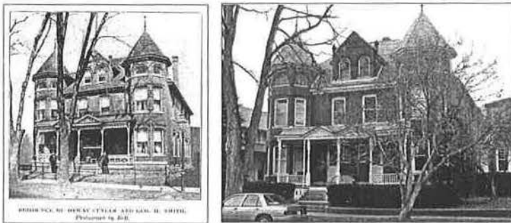
(Left) Figure 54. The Cutler Duplex (721–723 Avenue E, Site #155) as it appeared in 1896; (right) Figure 55. The same view as it appeared in 2012. 54
