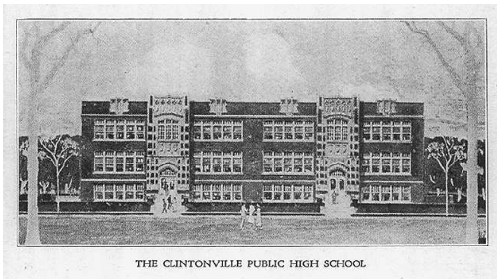
Figure 5 Clintonville High School front (north) elevation, c. 1918. (Diedrich, History of Clintonville , 1937)
