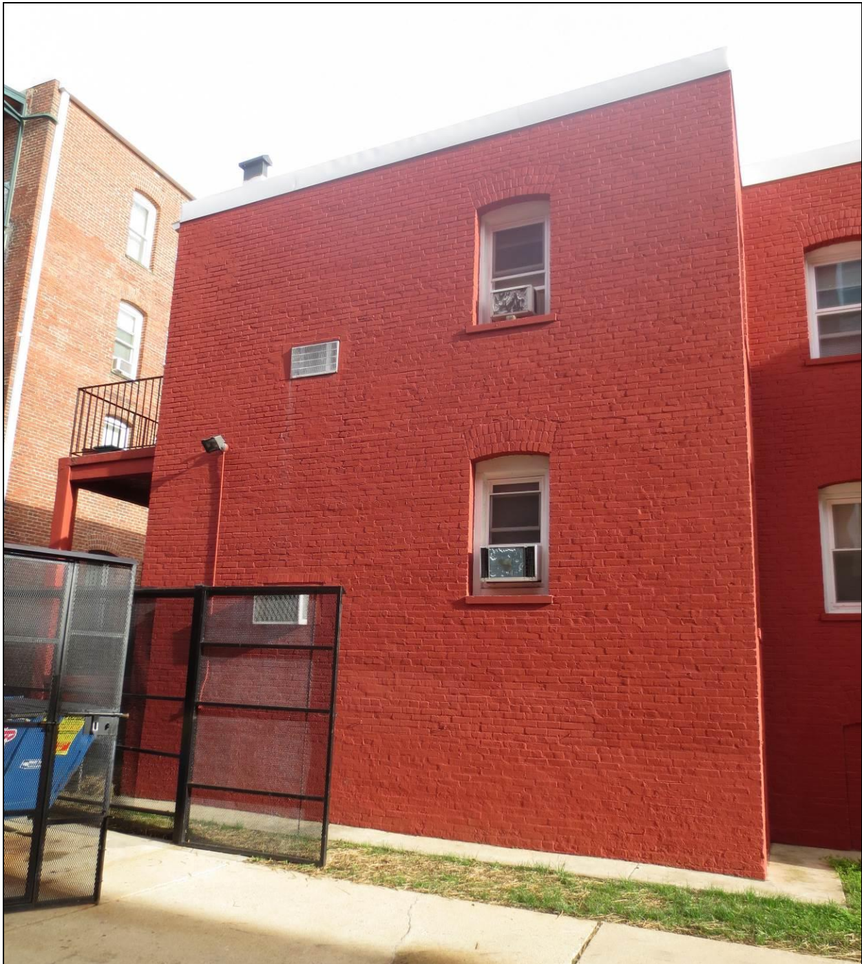
Exterior: End bay of south elevation, looking northwest
