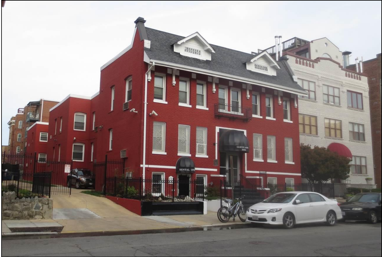
Exterior: Façade and south elevation, looking northwest
