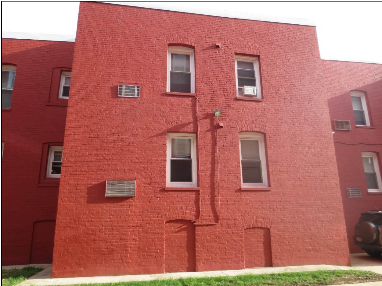
Exterior: Detail of middle bay, south elevation, looking north
