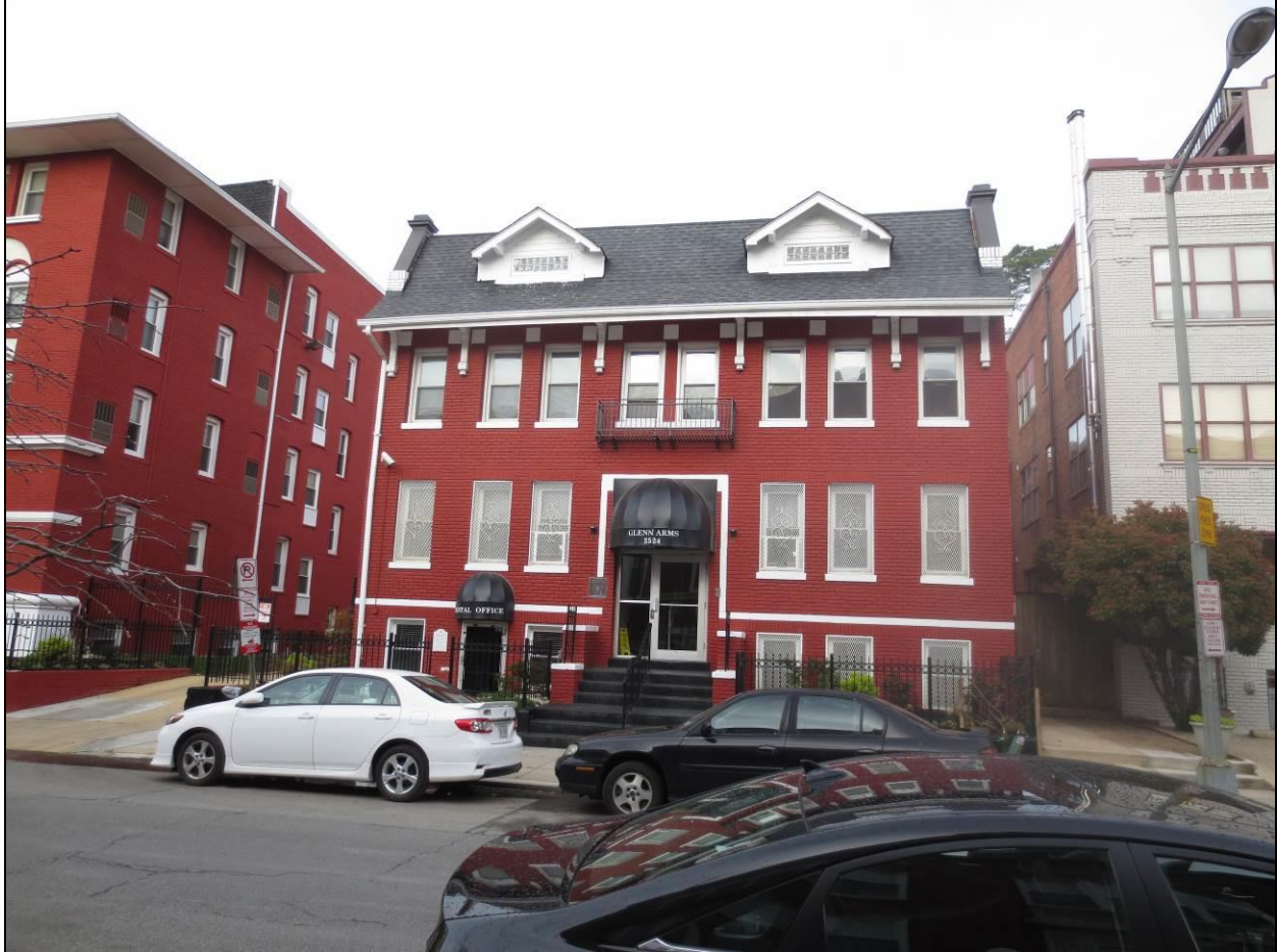
Exterior: Façade, looking southwest
