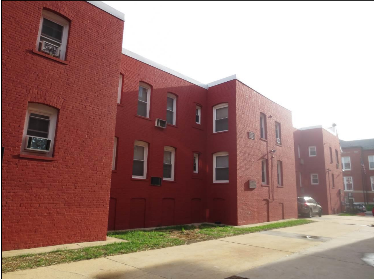
Exterior: South elevation, looking east
