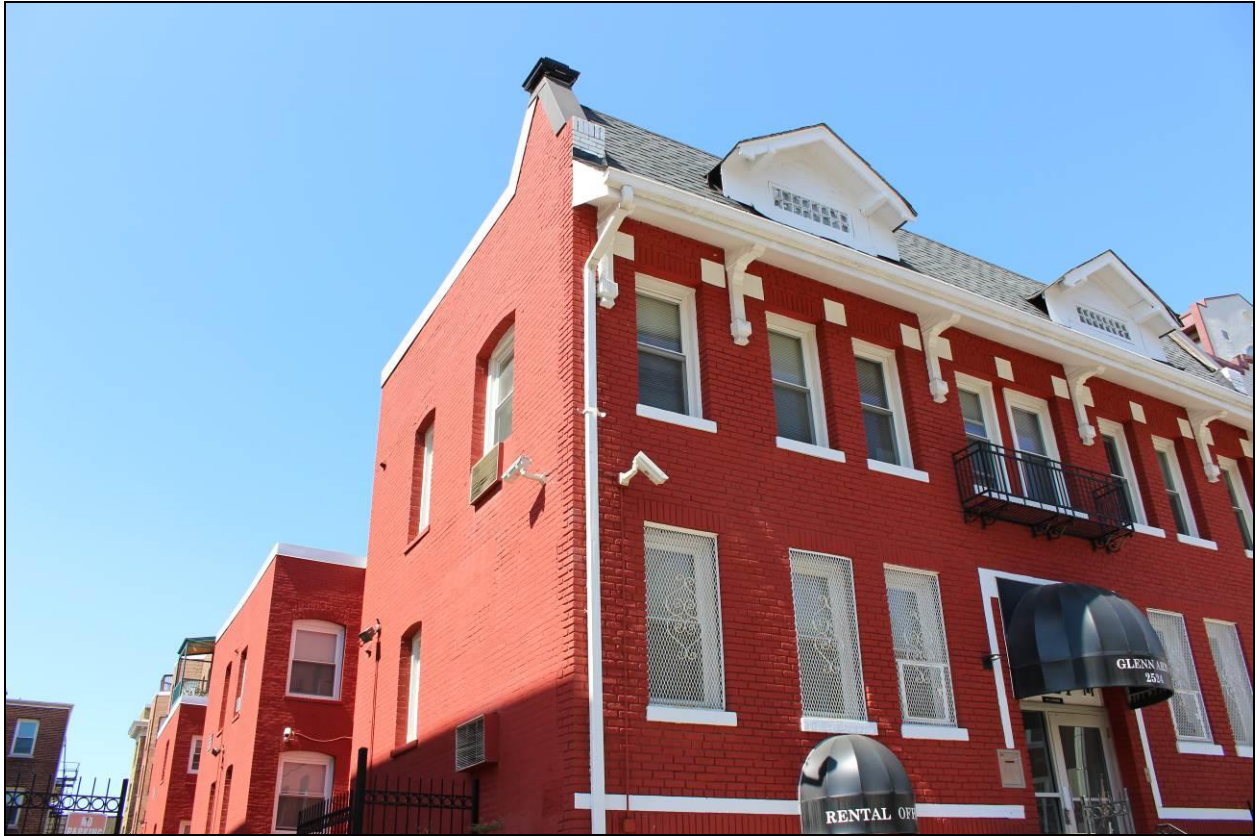
Exterior: Southeast corner, looking northwest
