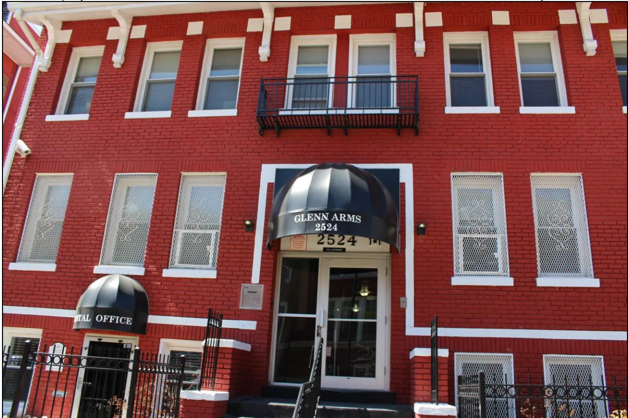
Exterior: Detail of façade, entry, looking west
