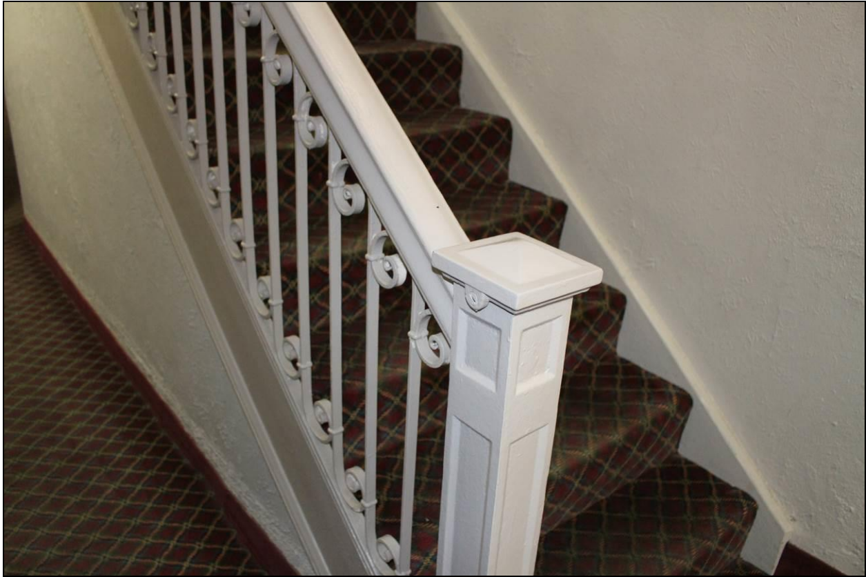
Interior: Detail of first floor stair
