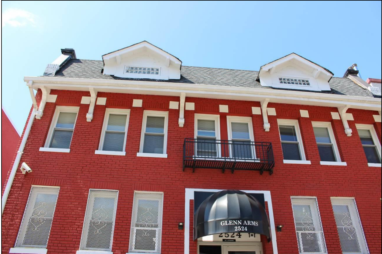
Exterior: Detail of façade, looking northwest
