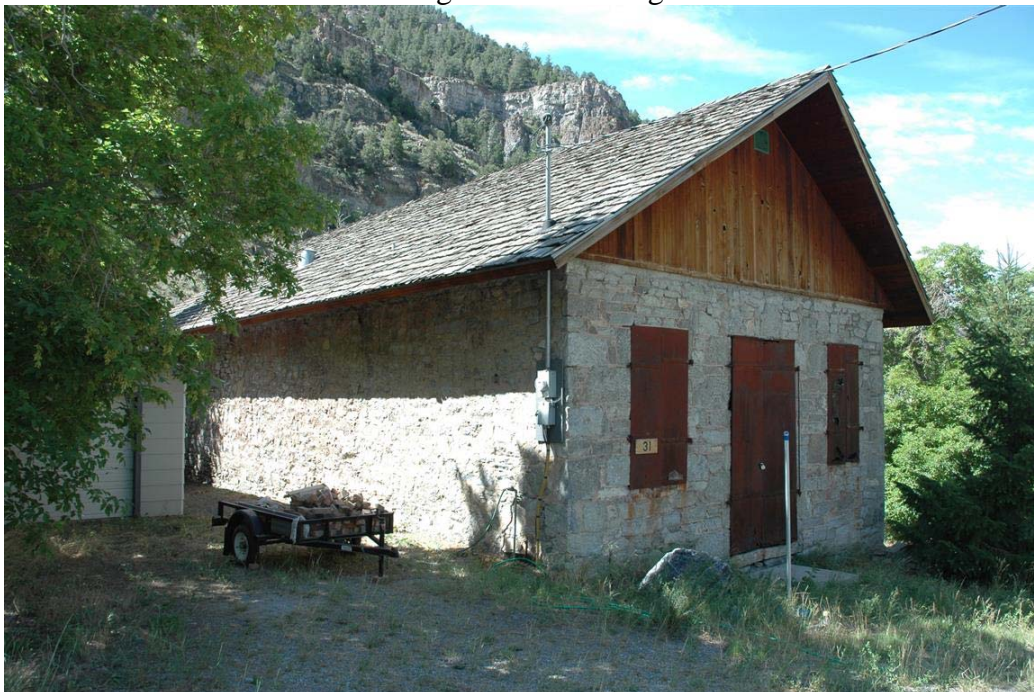
Photograph 2 of 12. North and east elevations of store building. Camera facing southwest.
