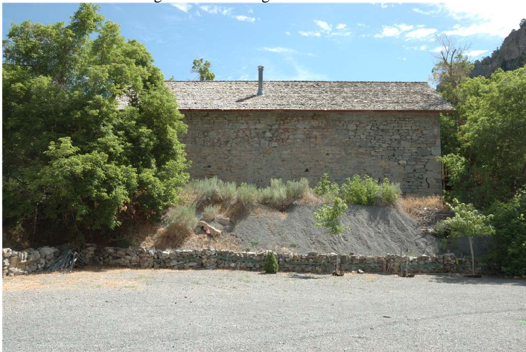
Photograph 4 of 12. West elevation of store building. Camera facing east.
