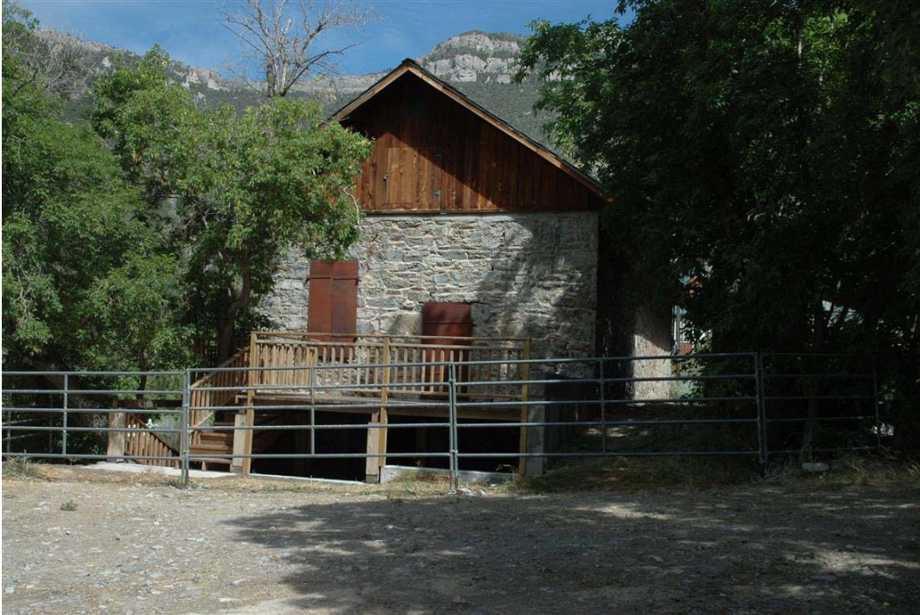
Photograph 5 of 12. South elevation of store building. Camera facing north.
