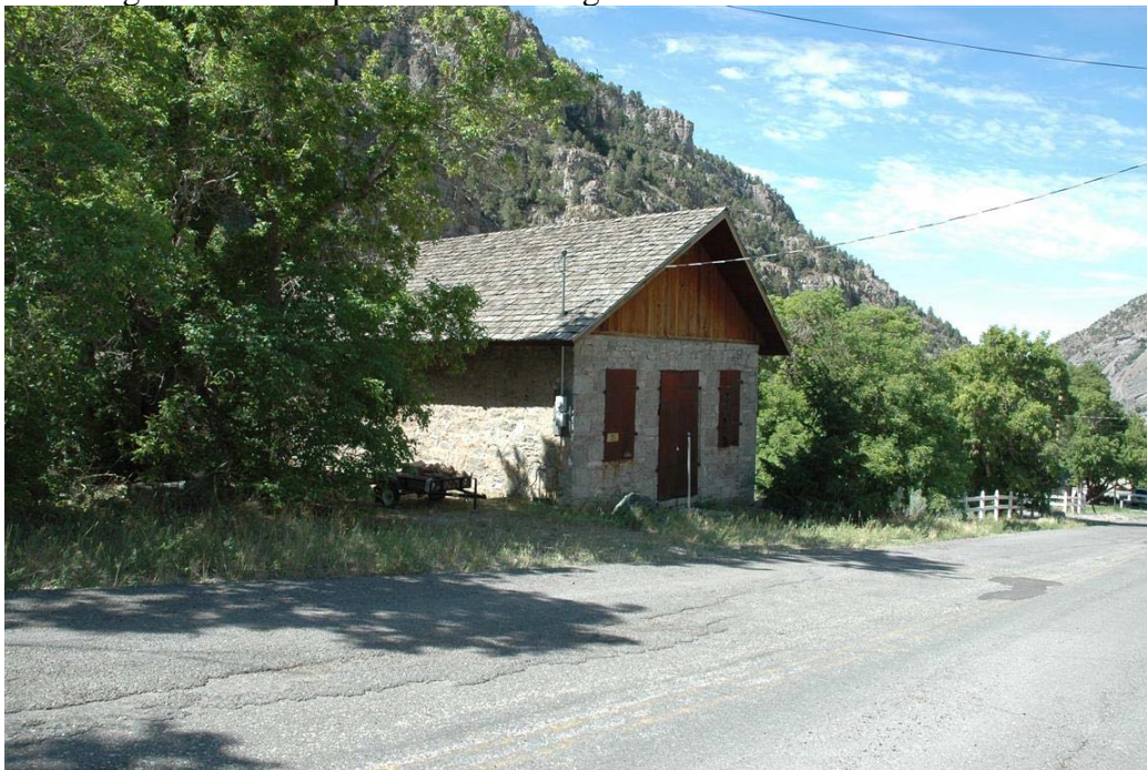
Photograph 1 of 12. View of building and streetscape. Camera facing southwest.
