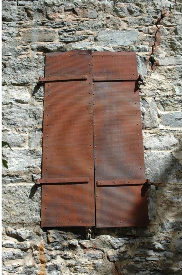
Photograph 7 of 12. South elevation of store building, shutter detail. Camera facing north.
