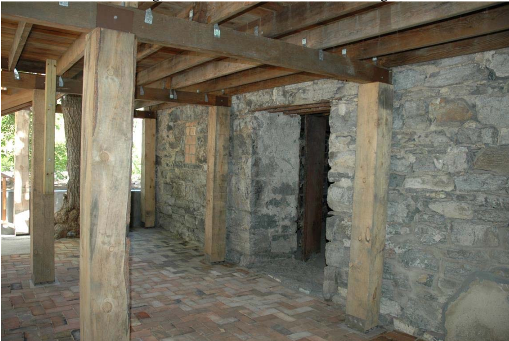
Photograph 6 of 12. South elevation of store building, basement entrance. Camera facing northwest.
