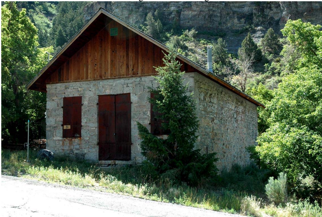
Photograph 3 of 12. North and west elevations of store building. Camera facing south.
