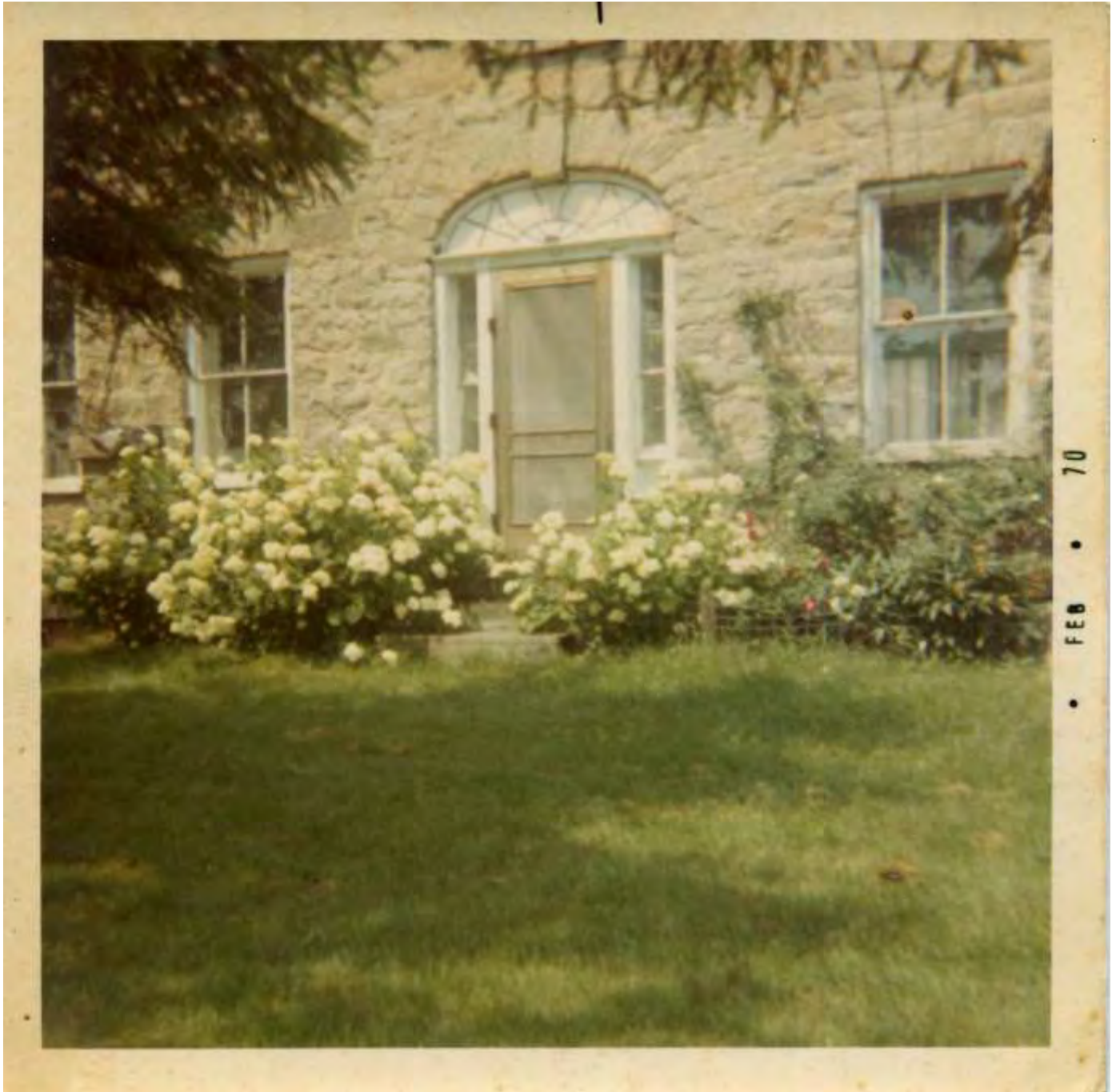
Stevens – Sommerfeldt House, Entry Door Detail ( February 1970)
